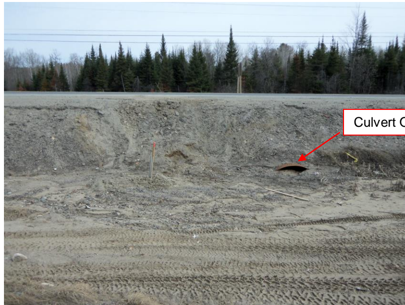
Culvert Outlet – Buried Culverts, South End
