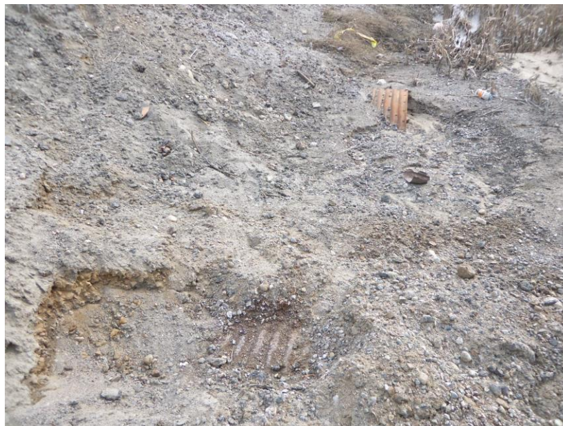
Culvert Outlet – Buried Culverts, South End
