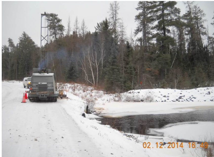
Testpit No. 2. Note: Cobbles encountered and groundwater in testpit.
