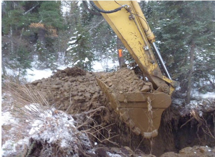
Culvert Invert – Looking West. Note: Berm of cobble/boulder size rock
