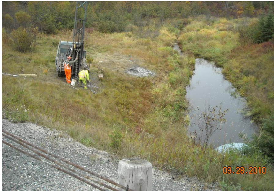
Drilling Boreholes for Culvert Extension – Looking East
