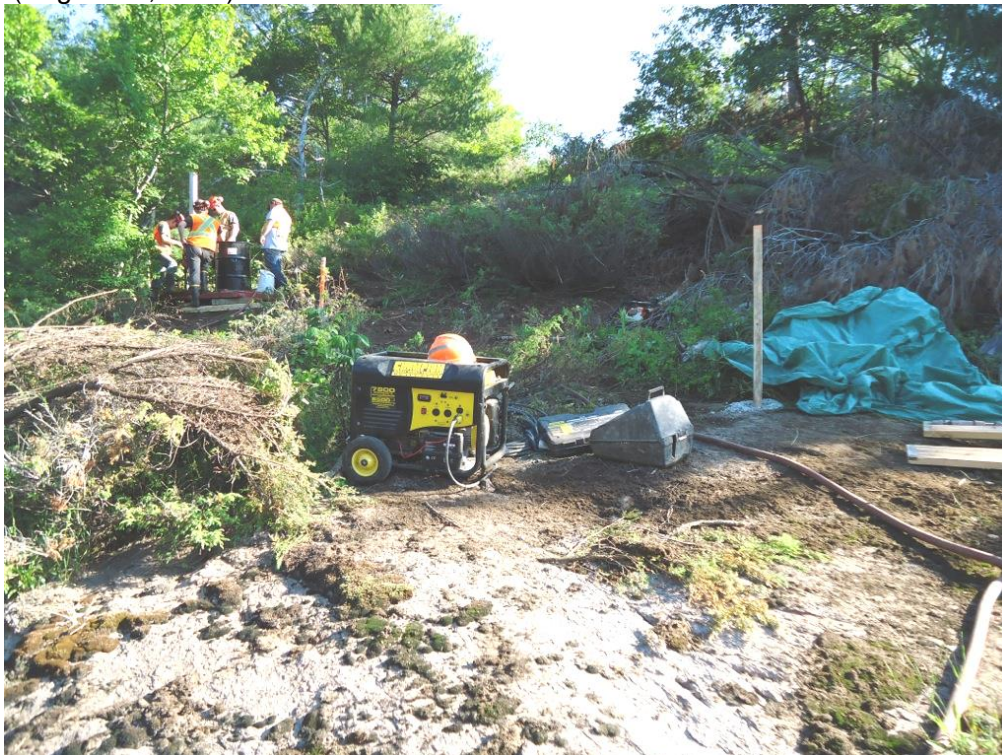
Photograph 4: Drilling at the location of borehole 3S-7 at the north pier of the SBL structure. Borehole 3S-3 is staked at right. (June 25, 2013)
