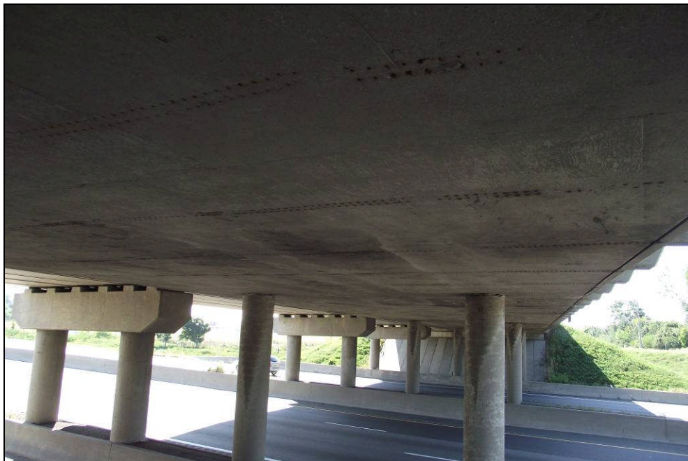
PHOTOGRAPH 1-14: Continuous deck slab and Girders of Waterloo Regional Road 36 Bridge. (August 28, 2012)
