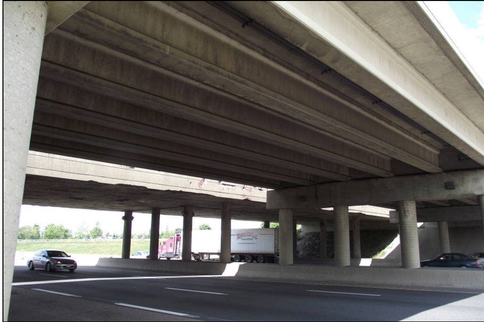
PHOTOGRAPH 1-7: Girders and continuous deck slab of Waterloo Regional Road 24 Bridge. (August 28, 2012)
