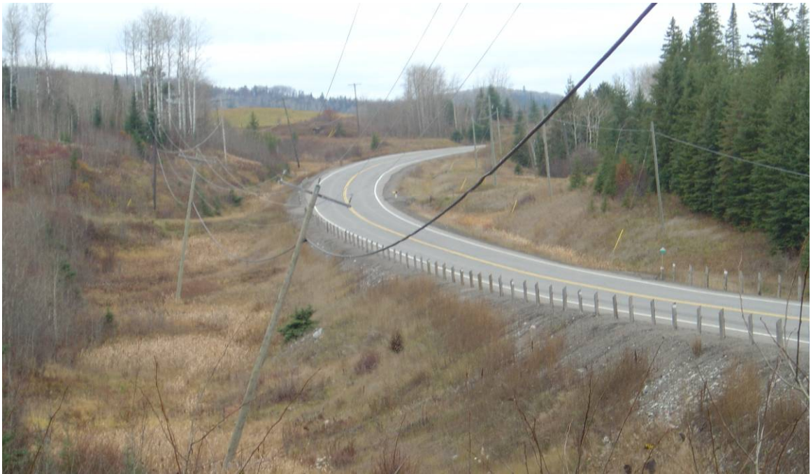
PHOTOGRAPH B5: Looking west from the south side of Highway 102, about 1.7 km east of Highway 11/17. Note the leaning hydro poles towards the north which indicates the possibility of soft soils. Approximate station 24+100 (October 27, 2009)
