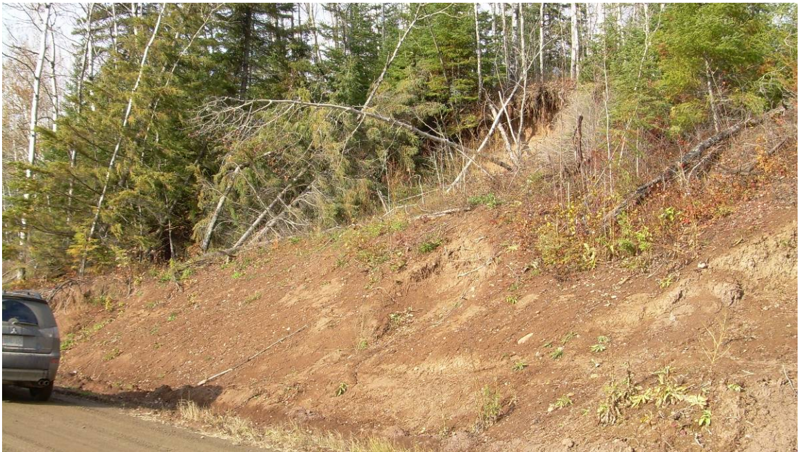
PHOTOGRAPH YS5: Looking northwest from Mokomon Road, about 100 m west of Highway 11/17. A cohesive soil slope failure is shown. Note the upper fallen trees. Approximate station 31+750 (October 27, 2009)
