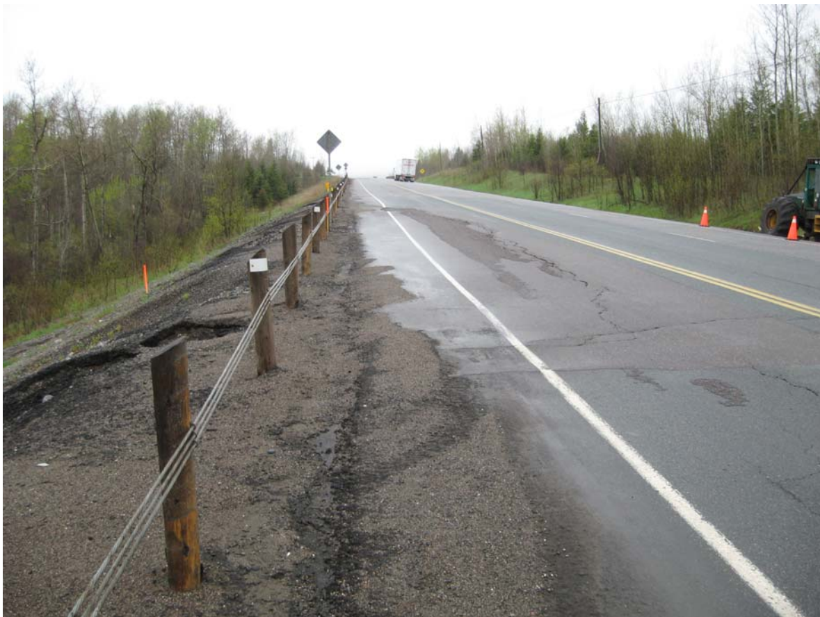
Highway 102 near station 13+500 May 30, 2008 Cracking and Asphalt Patching - Looking West
