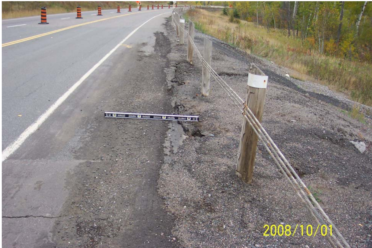
Highway 102 near station 13+500 October 1, 2008, a 180 mm vertical drop at the Rt. shoulder
