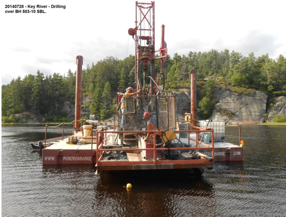
Photograph 1: Drilling from barge at SBL south pier
