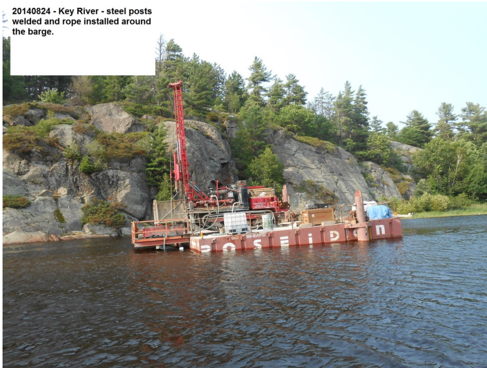
Photograph 2: Drilling from barge at SBL north pier
