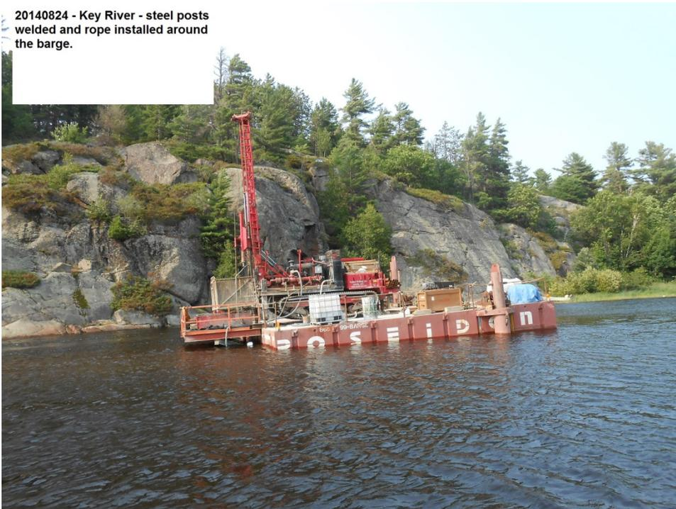
**Photograph 2: Drilling from barge at SBL north pier**
