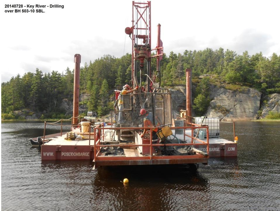
**Photograph 1: Drilling from barge at SBL south pier**
