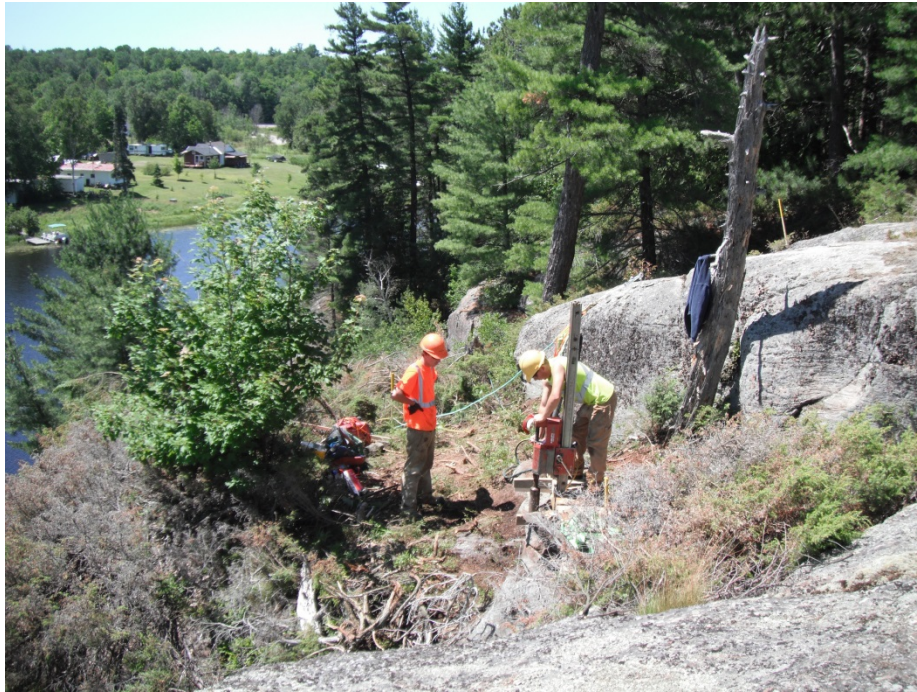
Photograph 1: Drilling with portable equipment at SBL north abutment
