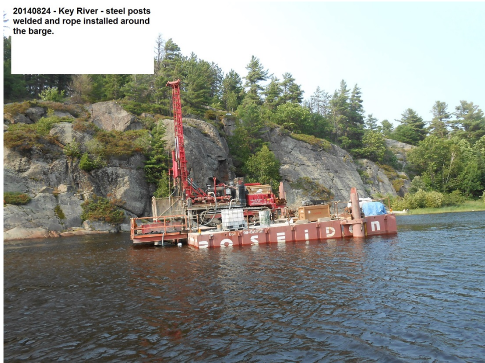
Photograph 2: Drilling from barge at SBL north pier
