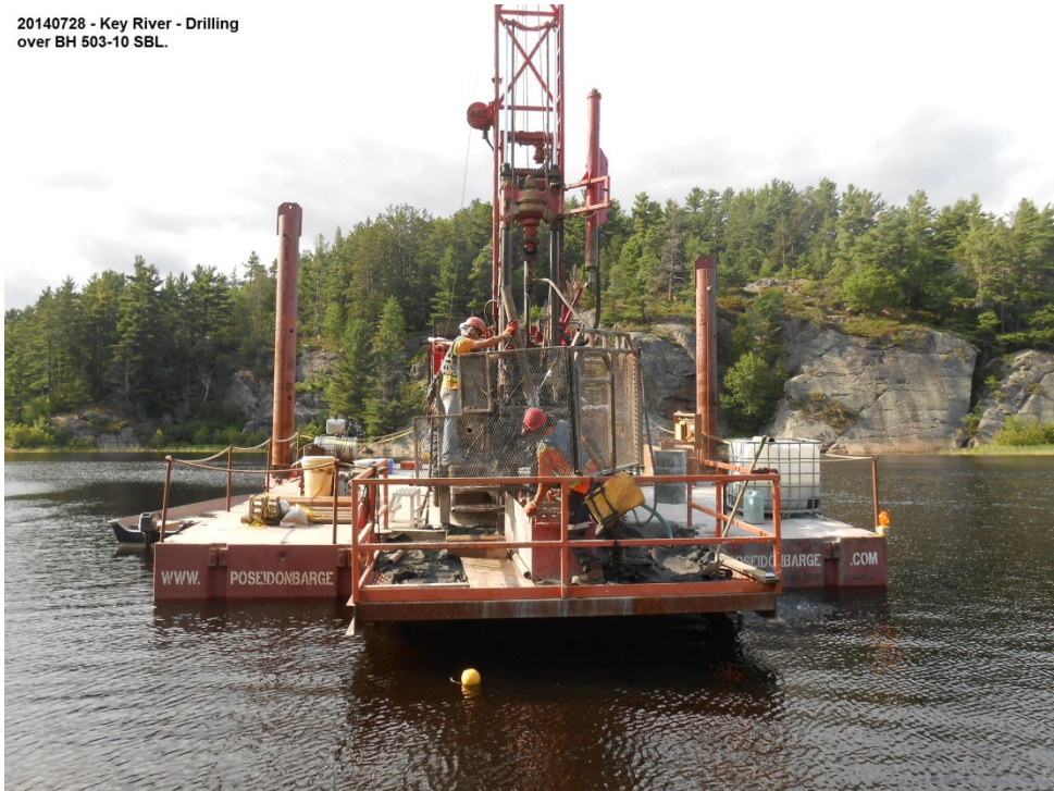
Photograph 1: Drilling from barge at SBL south pier
