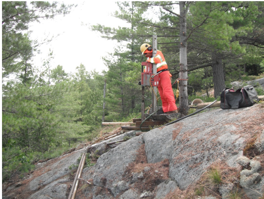
Photograph 2: Drilling with portable equipment at SBL south abutment
