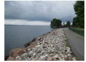
Photo 40 - Shoreline protection at end of Mowat...
