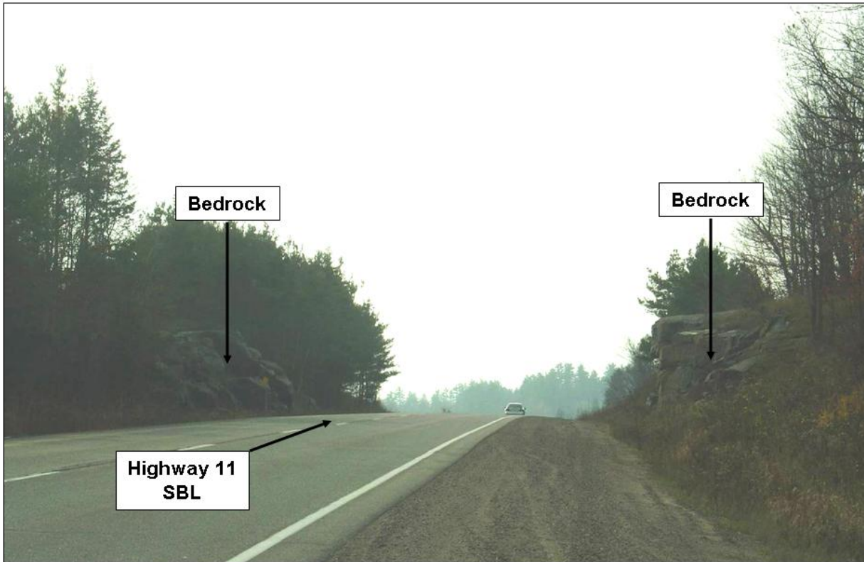
Photograph 49 VIEW: Looking south from west shoulder of Highway 11 SBL at about Sta. 22+680. Bedrock exposures (1.0 to 2.0 m) on both sides of Highway SBL at Sta. 22+620 to 22+680. (Nov. 2007)
