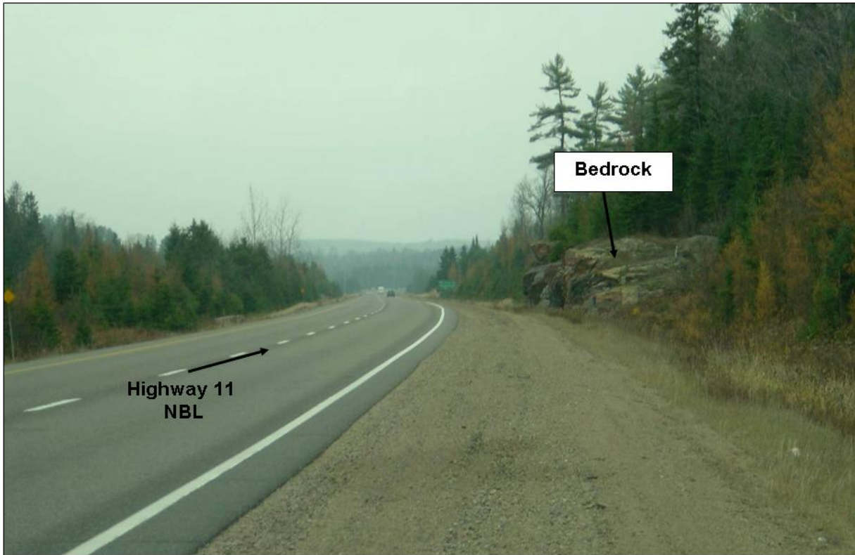
Photograph 5 VIEW: Looking north from east shoulder of Highway 11 NBL at about Sta. 18+100 at 1.5 to 2.0 m bedrock cut (Sta. 18+160). Stephenson Road 8 is 1.0 km in distance. (Nov. 2007)
