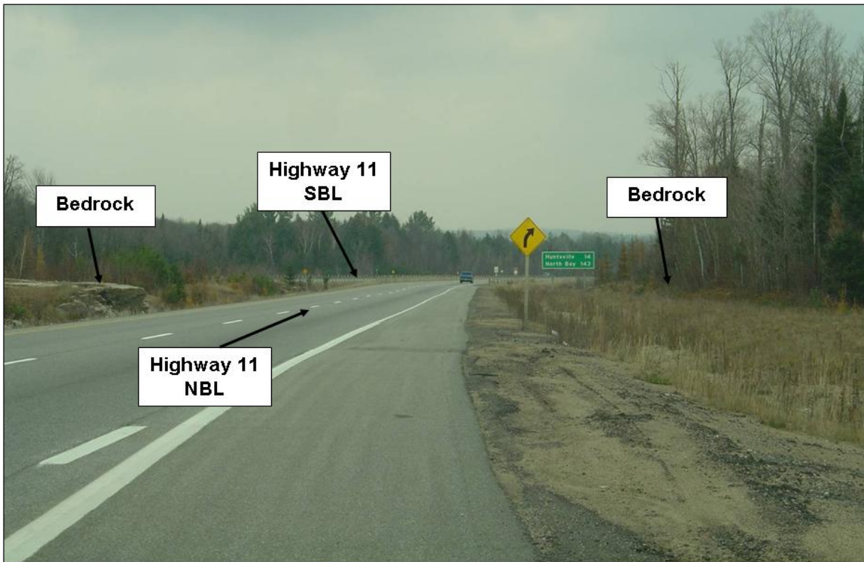
Photograph 1 VIEW: Looking north from east shoulder Highway 11 NBL at about Sta. 16+700. Bedrock outcrops typically up to 1.0 m visible in median. (Nov. 2007)
