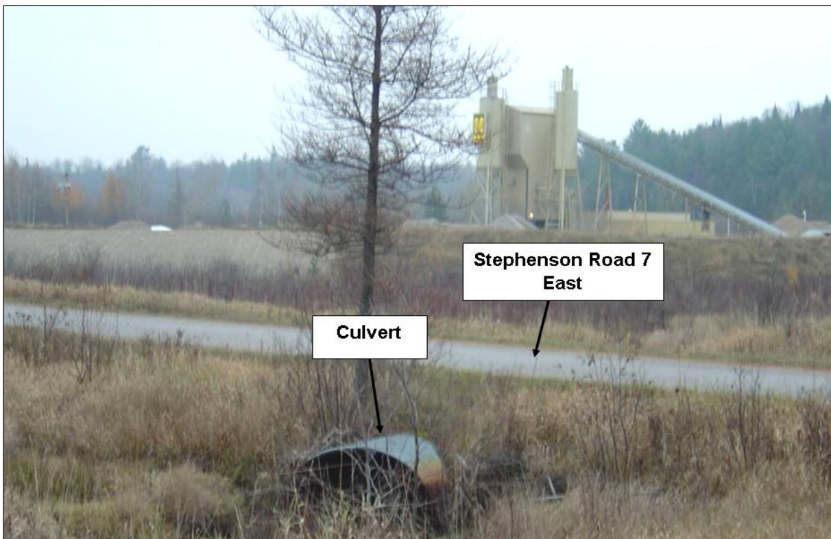
Photograph 8 VIEW: Looking east from east shoulder of Stephenson Road 8, at about Sta. 19+080. Culvert (2200 SPCSP) ON Stephenson Road 7 East in foreground with Muskoka Ready Mix Concrete plant on fill pad in background. (Nov. 2007)
