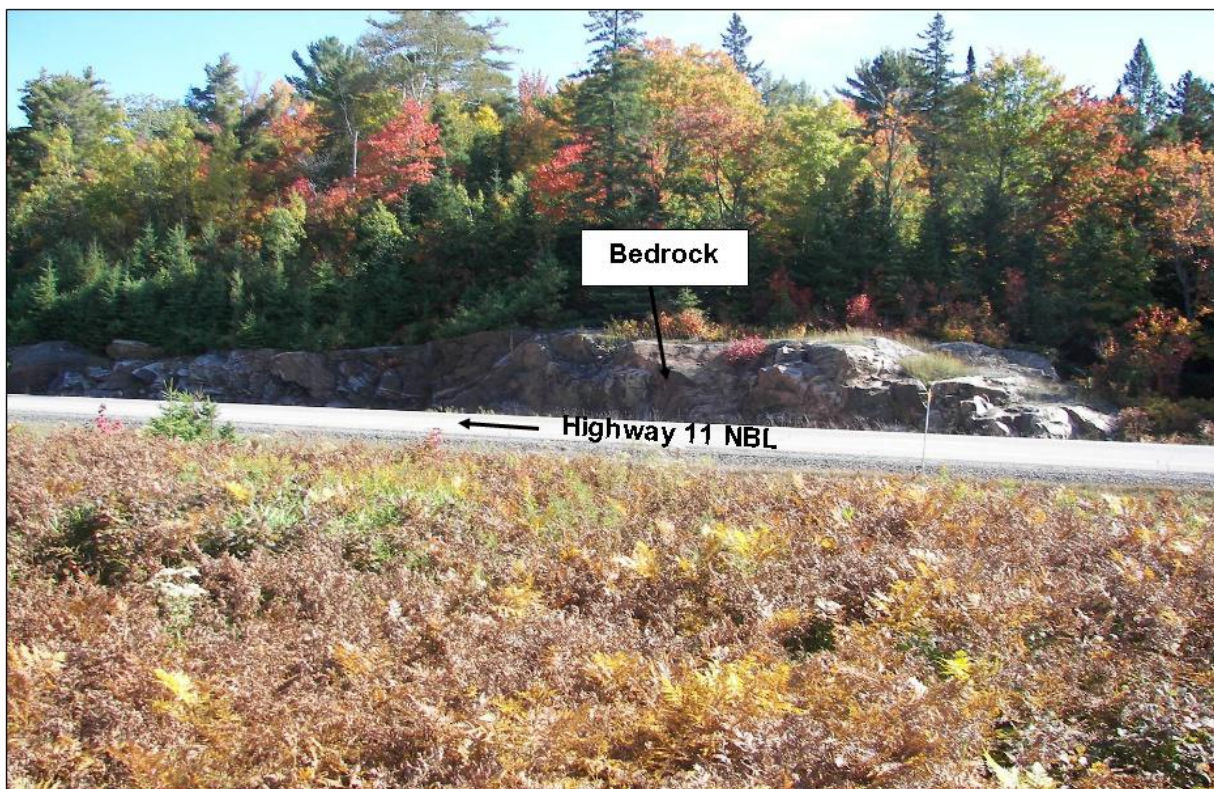
Photograph 10 VIEW: Looking northeasterly from median of Highway 11 at about Sta.19+960. Rock cut in photograph is 1.0 to 3.0 m high and located about 240 m south of I/C Alt. 1A and 1C. (Sept. 26, 2008)
