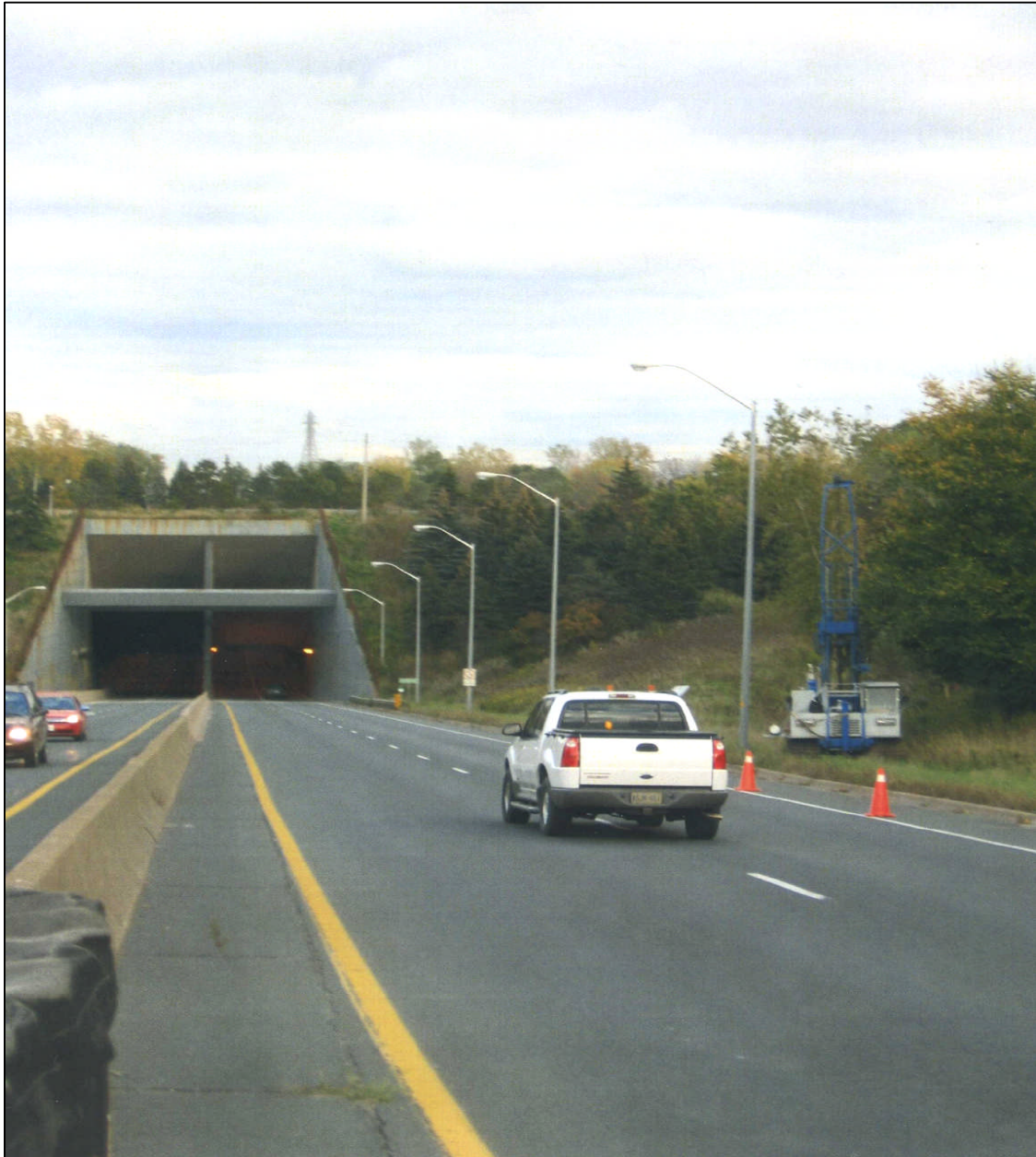
Photograph 1: Viewing towards east at centreline of East Main Street. Note drilling rig setting up on Borehole EM2. West entrance of East Main Street tunnel under the Welland Canal is also shown in photo. (October 16, 2008)
