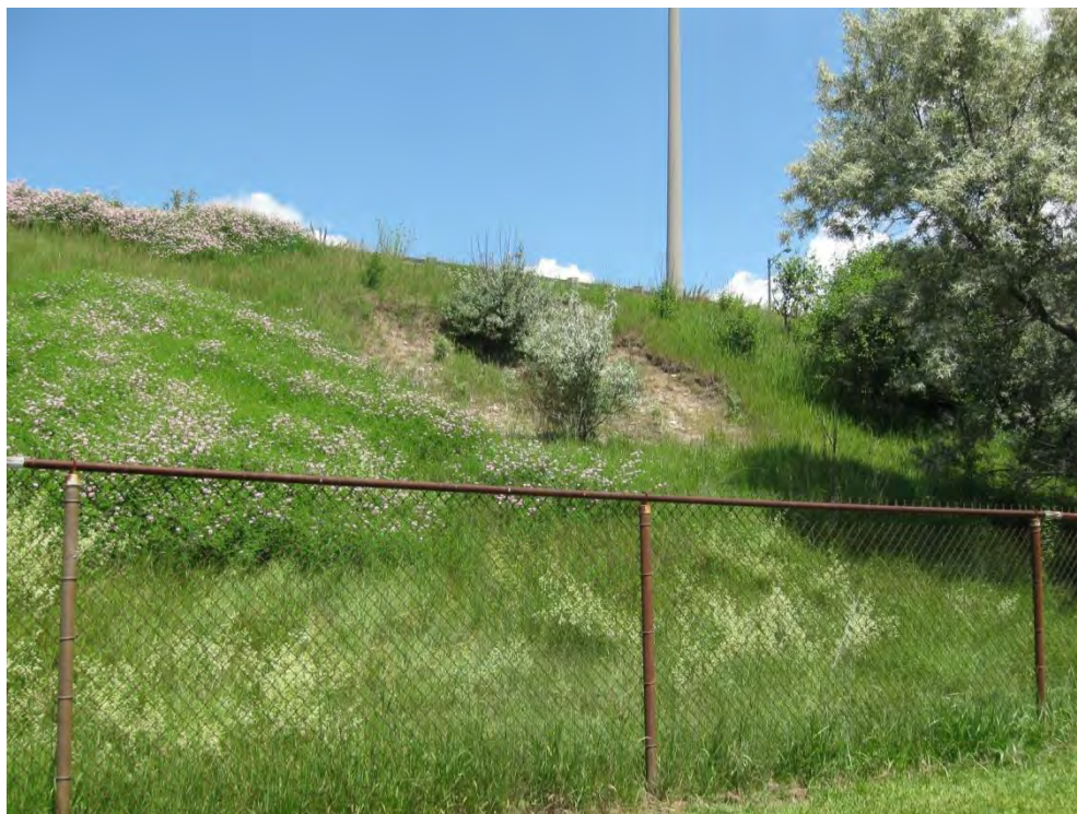
Photograph 1: Slope failure between Stations 16+770 and 16+780 RT, looking north from Overland Drive (June 23, 2009).
