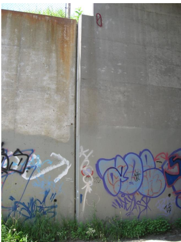
Photograph 4: Expansion joint between Panel 21 and south end of west abutment wall. Displacement of retaining wall relative to west abutment is evident in top part of photograph.
