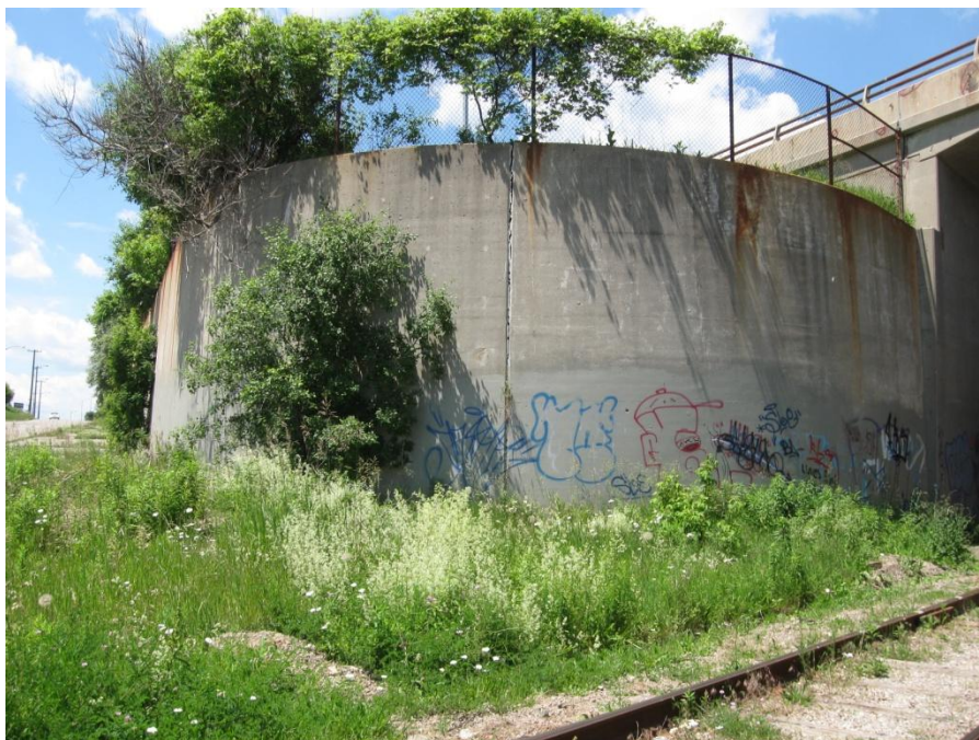
Photograph 2: View of construction joint between panels 20 (left side of photograph) and 21 (right side of photograph).
