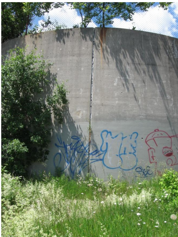
Photograph 3: Joint between Panels 20 and 21 at east end of retaining Wall D. Construction joint appears to be opening up.
