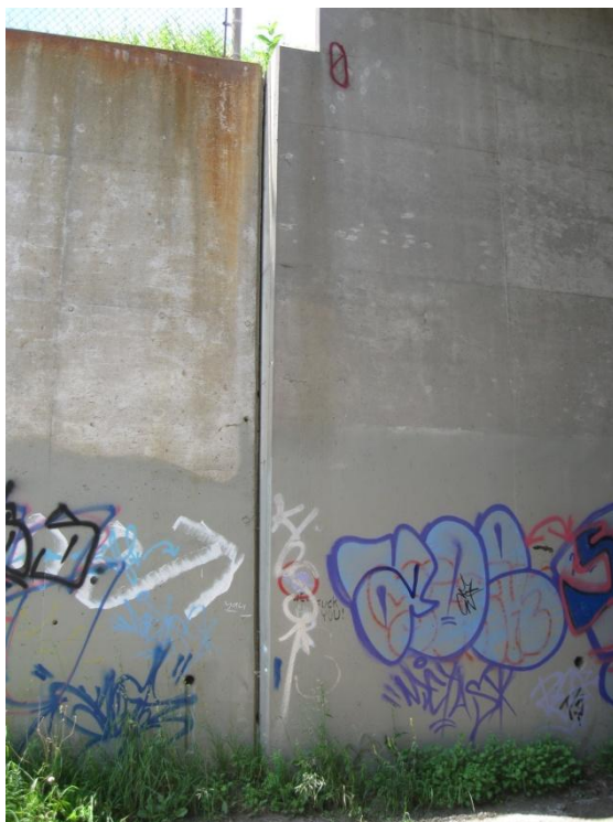
Photograph 6: Rotation of segment of retaining wall 'D'.
