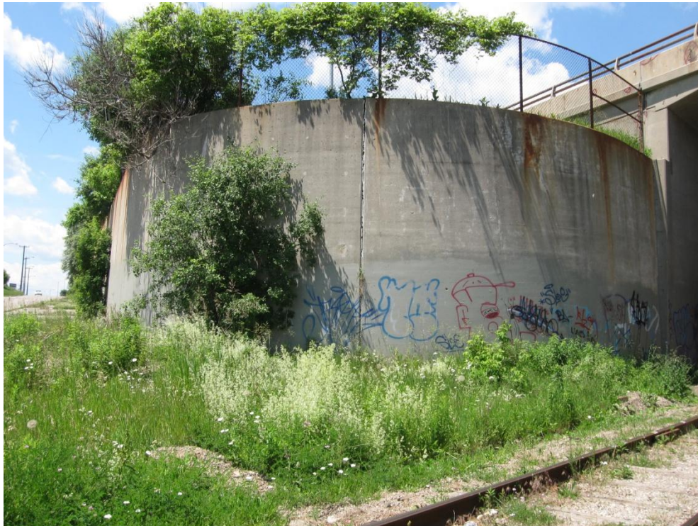
Photograph 5: Movement of joint of retaining wall 'D' at southwest corner of CNR overhead structure.
