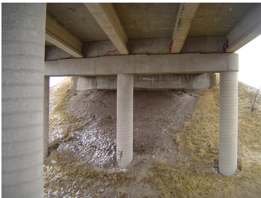
Photograph 5: East abutment foreslope. Loose granular fill is exposed at surface.
