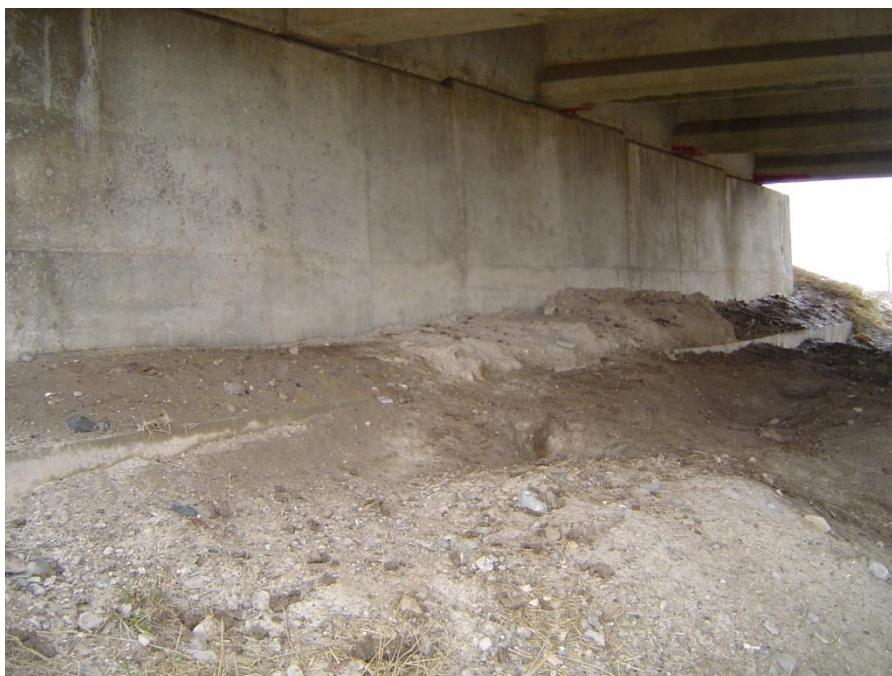
Photograph 4: Area of loose fill at foreslope of west abutment; view from south elevation.
