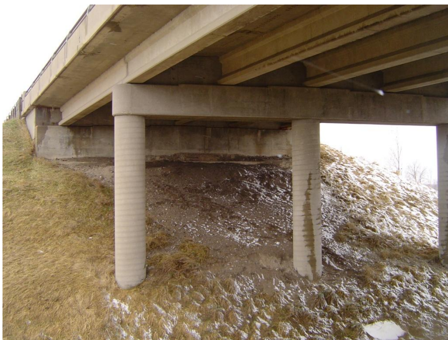
Photograph 3: Loose fill at foreslope of west abutment.
