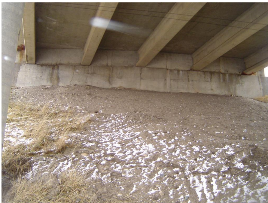
Photograph 6: East abutment. Close up of loose fill on foreslope.
