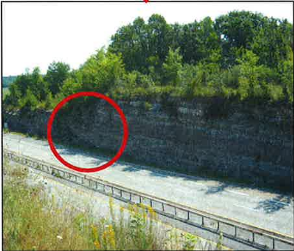
Example of overbreak of the face due to sub-parallel joint sets
