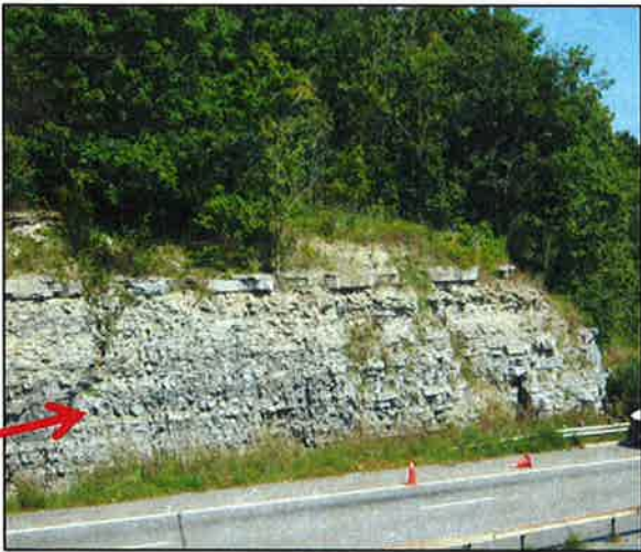
Example of seepage from a layer about 4m above the highway; blocky and ravelling face, minor overhangs.
