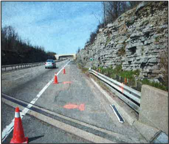
Looking west from east end of cut: Note overhangs due to gravity falls
