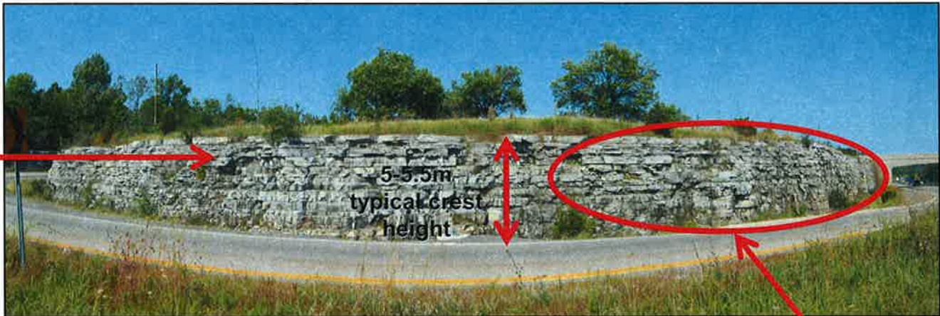
Example of very blocky face, minor ravelling, overhangs < 0.5m
