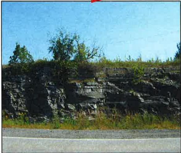
Example of blocky face due to poor blasting practices resulting in ravelling and minor overhangs
