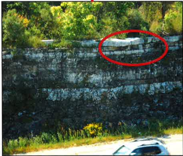
Example of overhangs resulting in gravity falls
