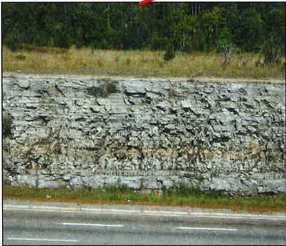
Example of blocky structure and ravelling due to ongoing freeze-thaw processes
