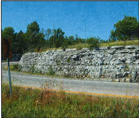
Example of very blocky face, minor ravelling, overhangs < 0.5m
