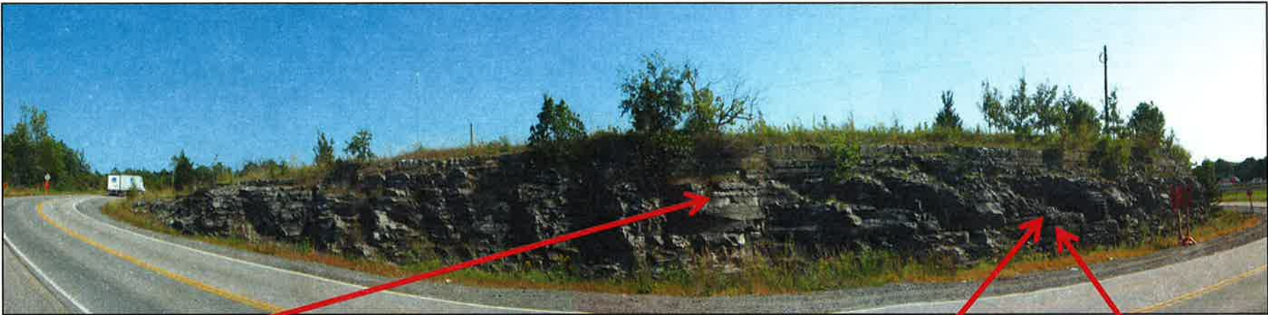
Example of very blocky face, minor ravelling, overhangs < 0.5m
