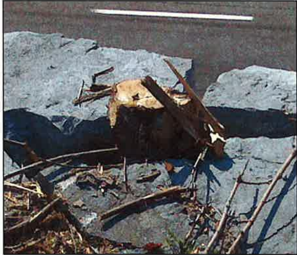
Example of tree stumps jacking blocks open on the crest of the face
