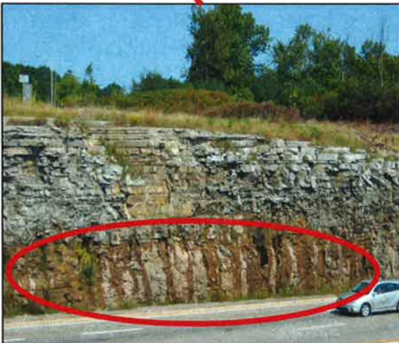
Example of seepage from a layer about 4m above the highway; blocky and ravelling face, minor overhangs.
