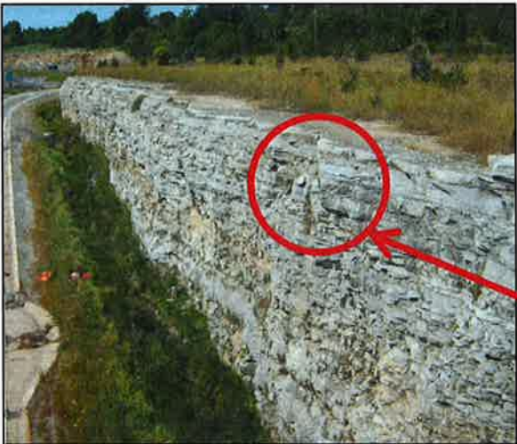
Example of saw tooth profile of rock face due to overbreak along sub-parallel joint sets Minor overhangs
