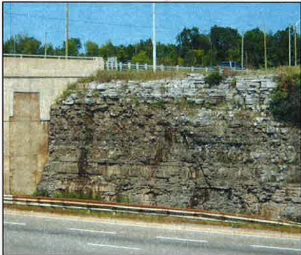
Example of minor seepage and small overhangs
