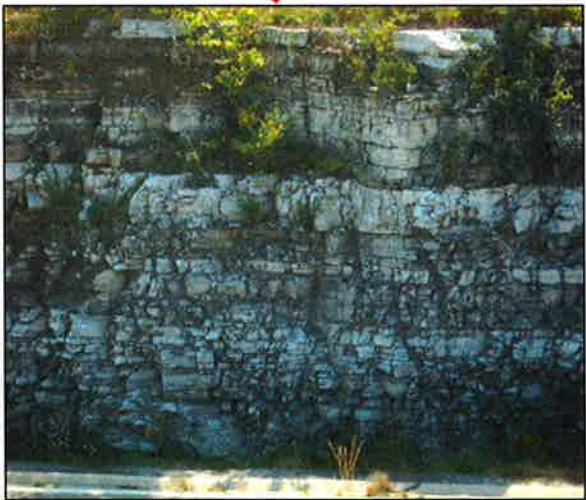
Example of blocky rock face and ravelling failures
