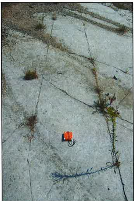
Three near vertical joint sets clearly visible on the crest above the cut. Along with near horizontal bedding, defines the blocky structure of the rock mass.
