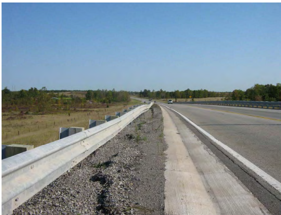
Photo #2: Sloughing of granular inside guide rail, west side of north embankment facing north.
