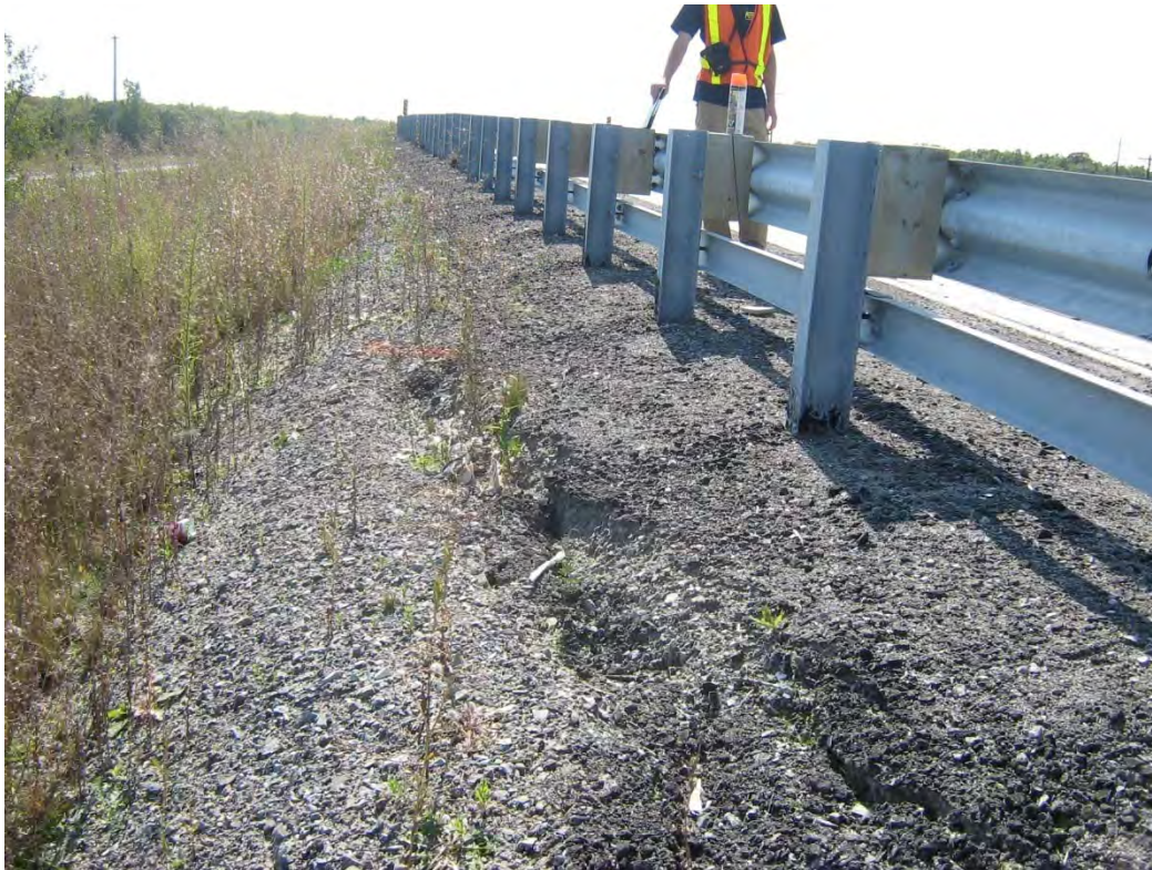
Photo #5: Tension crack along crest of east slope of north embankment, facing south.
