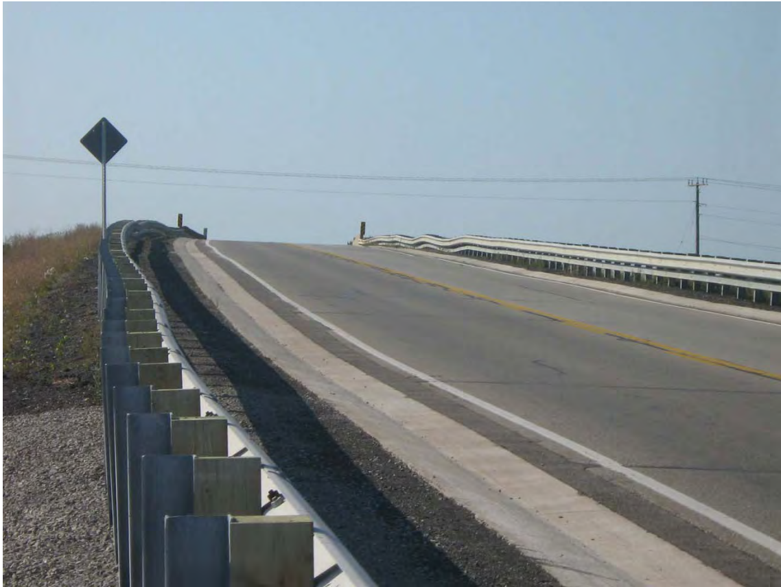
Photo #4: Tilting of guide rail along north embankment, facing south.
