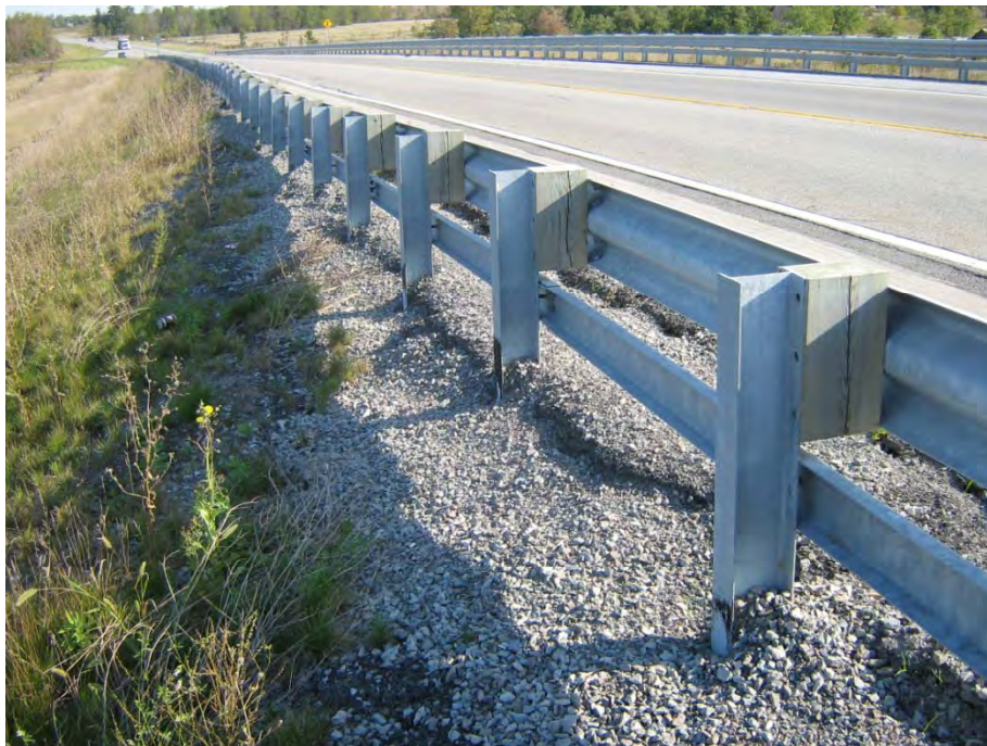
Photo #1: Sloughing of granular at crest of slope, west side of north embankment facing north.
