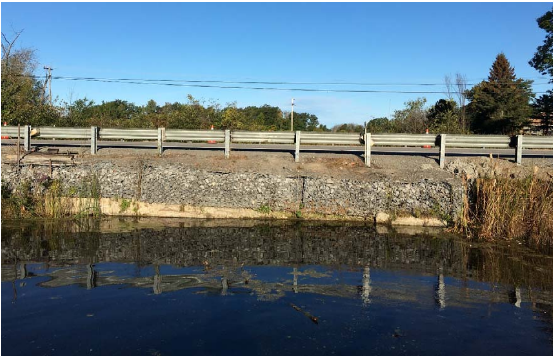
Photograph 2: Looking west towards the existing culvert inlet. Note that right side of culvert has settled more than left side (2017-09-13)
