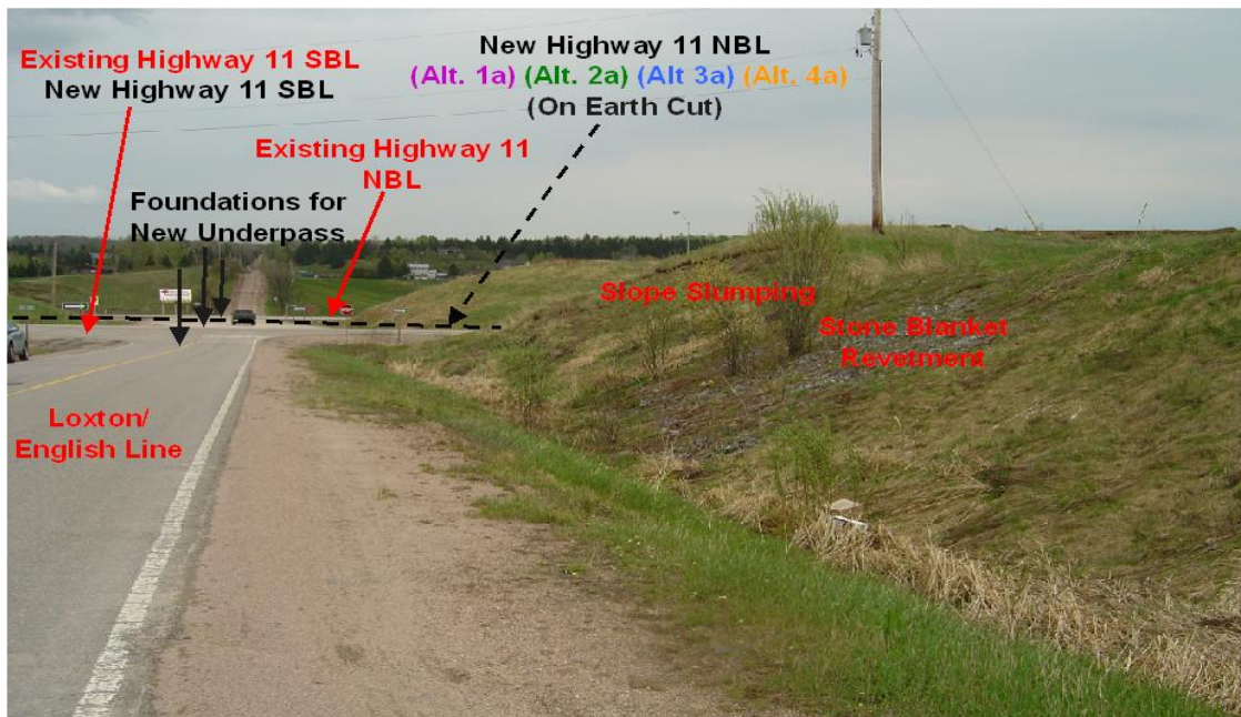
Photograph 20: View looking east from south shoulder of Loxton / English Line about 30 m west of Highway 11 SBL. Active slope slump in 5 m high slope at south west corner of at-grade crossing. (May 8, 2007)
