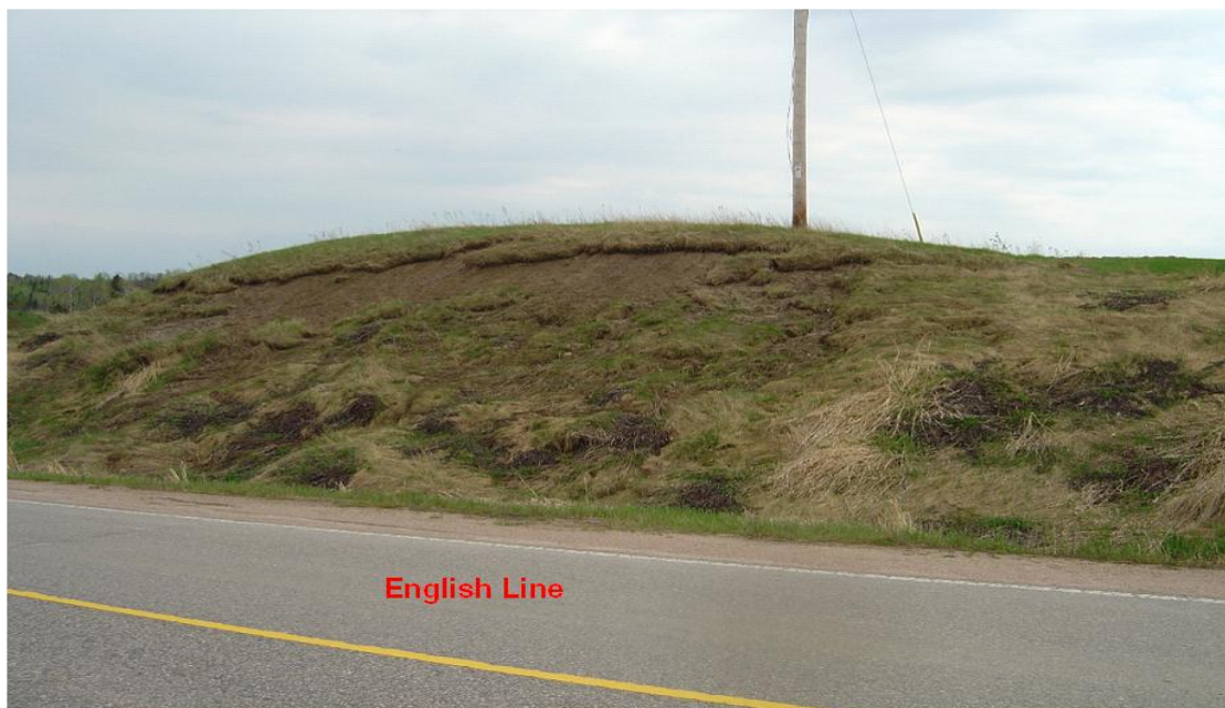
Photograph 21: Close up of slope slump at south west corner of Highway 11 SBL at English Line. (May 8, 2007)
