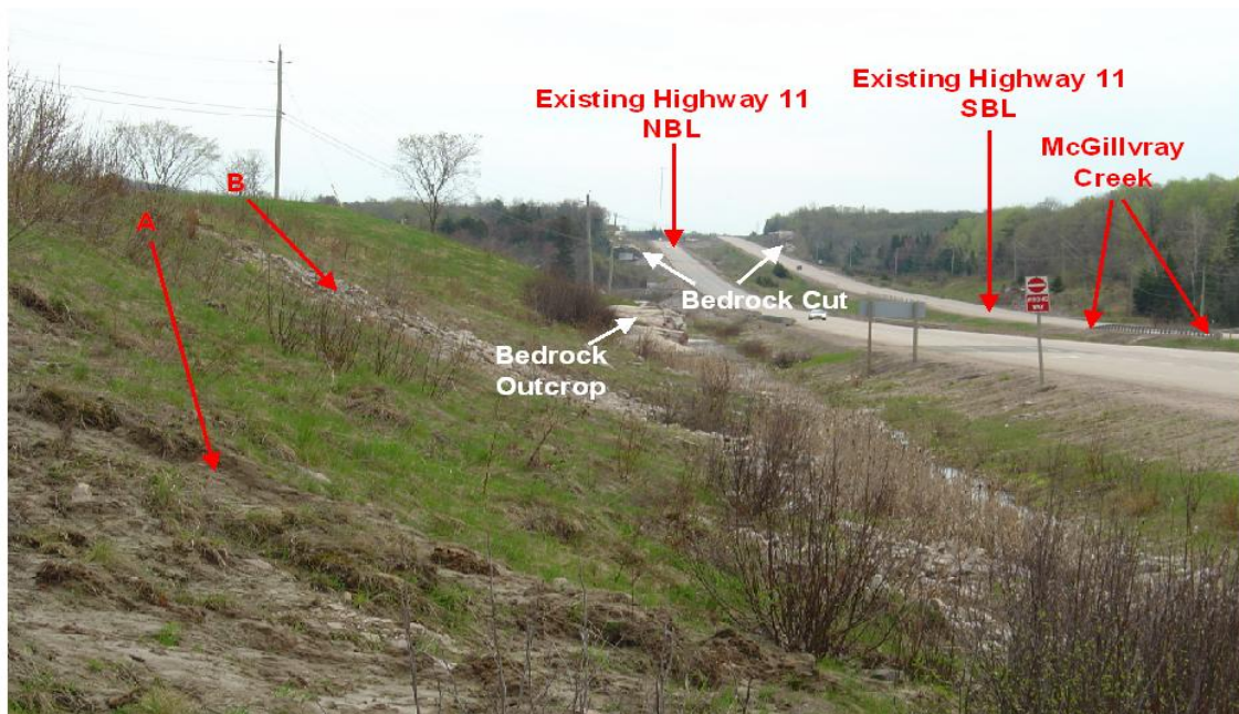
Photograph 5: Looking south from south side of Proudfoot Road along NBL ditch line. Slope slump/erosion in foreground A. Previous erosion area blanketed with stone B. (May 8, 2007)
