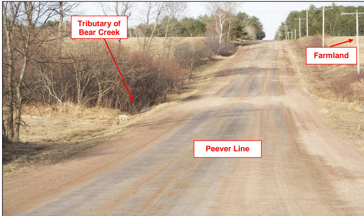
Photograph 15 VIEW: Looking east along Peever Line about 50 m east of Oakwood Road. Grade slopes down to crossing of tributary of Bear Creek at mid photo depth. Note gravel road surface in good condition. (April 17, 2008)
