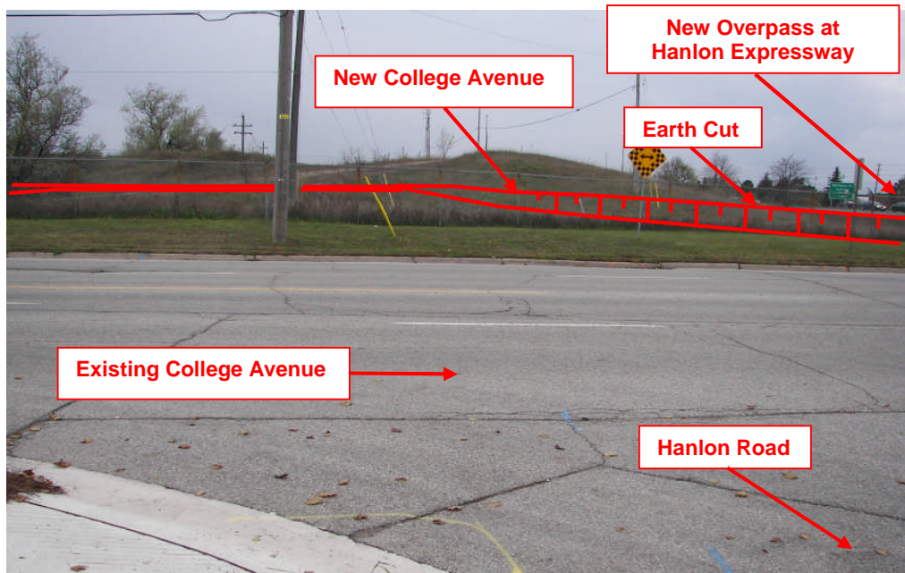
Photograph A-4: Viewing north from west corner of Hanlon Road and College Avenue intersection towards new College Avenue alignment. Note that high ground west of Hanlon Expressway will require earth cut. (Nov. 15, 2007)
