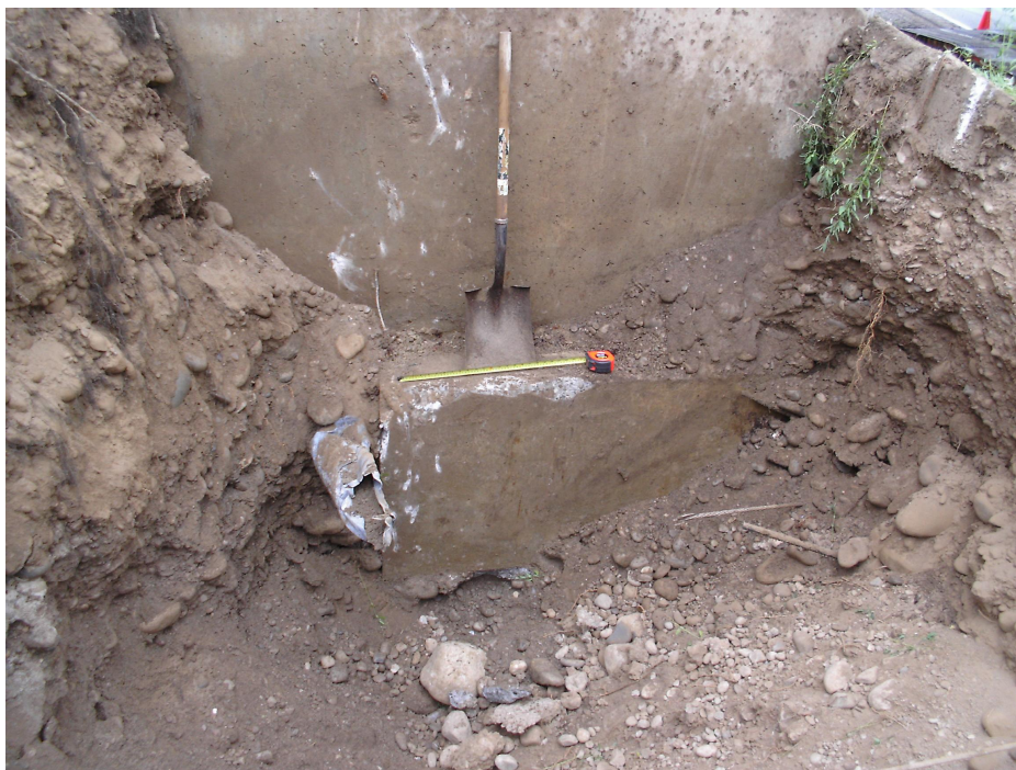
Photo 3: North Abutment Footing – West Side (Test Pit 101).
