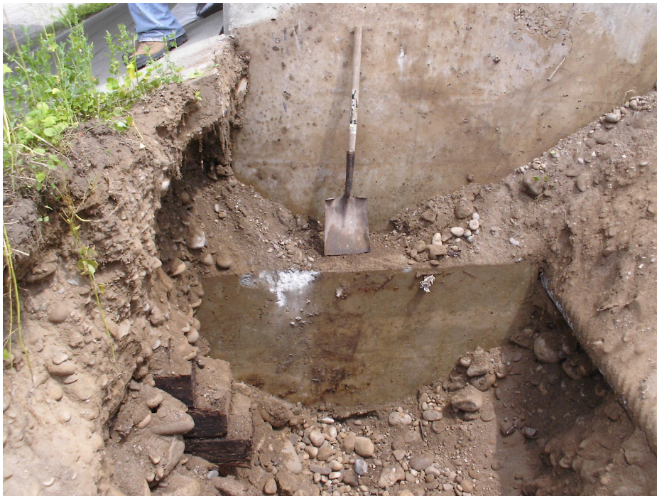
Photo 6: South Abutment Footing – West Side (Test Pit 104).
