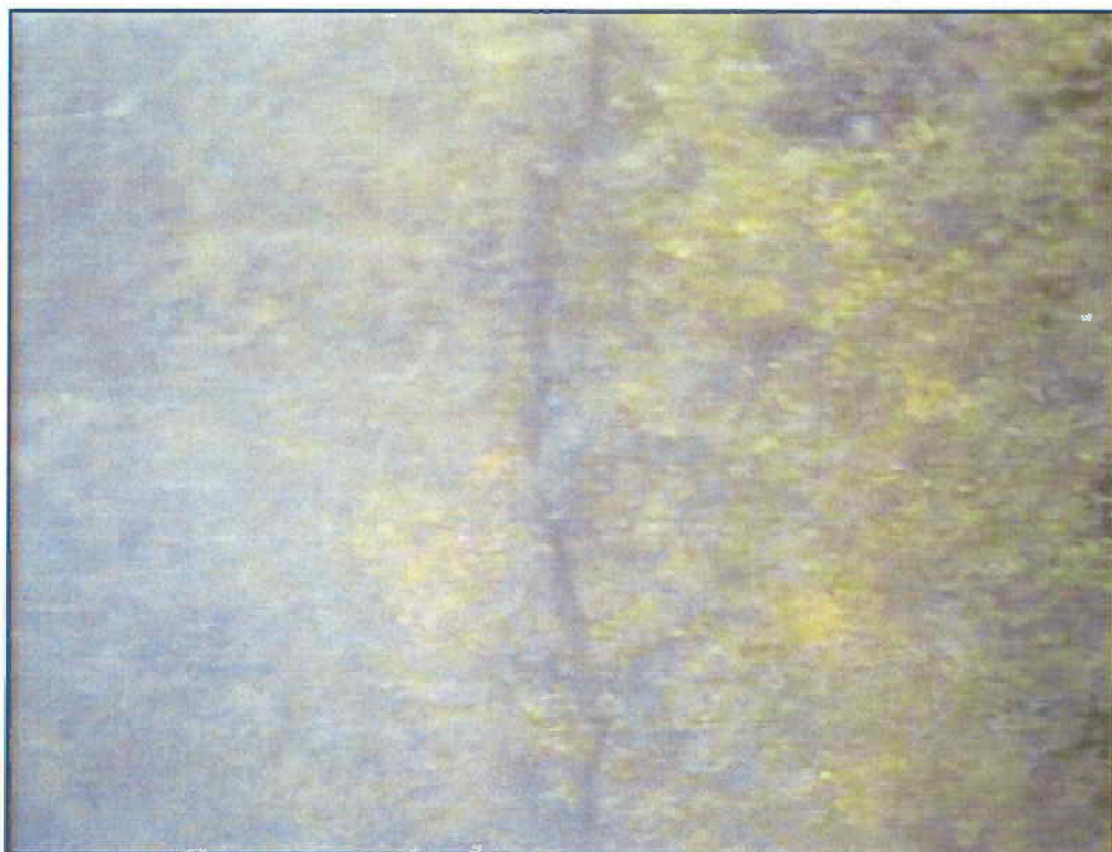
Photograph 1-10: Pier C - Crack 2 mm on Centre Line of East Face
