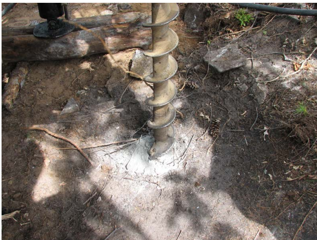
Image 4. Collaring the core hole using a corundum-tipped auger bit.
