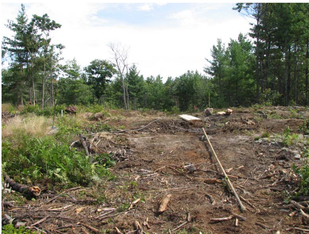
Image 2. Looking south along the proposed Hwy 69 alignment. Note drill rods with clay core orientation device affixed to end.
