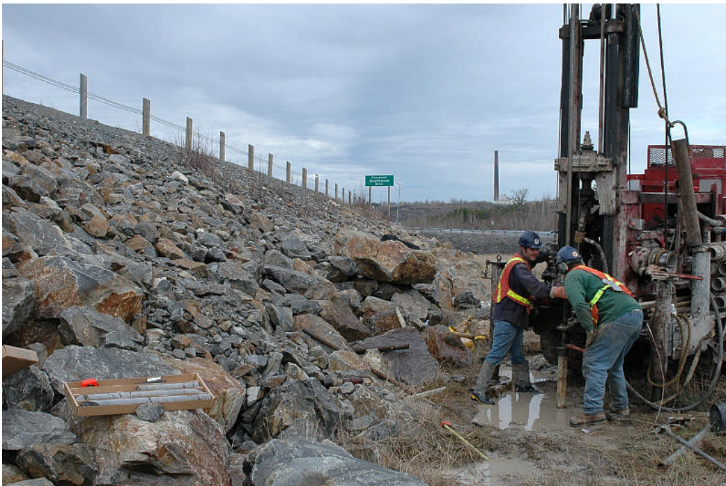
Photograph 1: Looking west from toe of embankment north of Highway 17 at about Sta. 11+882, borehole L5-1, 170 m east of Southview Drive and Highway 17 intersection. About 6 m high rockfill embankment of the existing Highway 17 is in view. Drillers are rock coring in borehole L5-1. (April 30, 2007)
