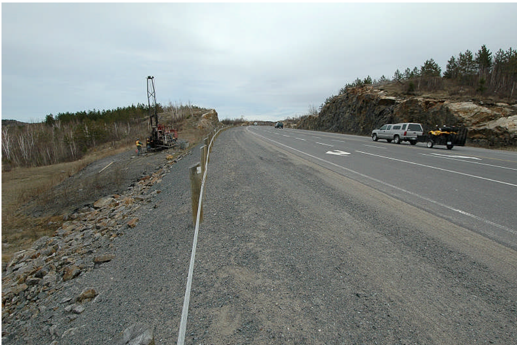
Photograph 2: Looking east from the shoulder of Highway 17, Drill rig is at about Sta. 11+906, on borehole L5-3. Rock cut of about 8 m high in view at right side of the photograph. (May 1, 2007)
