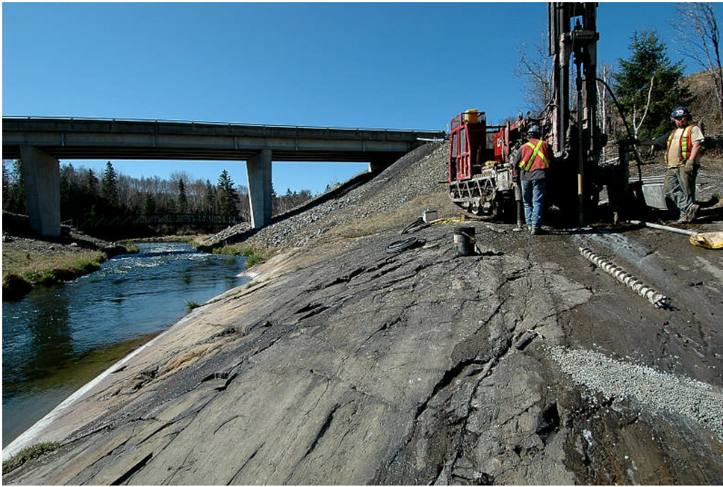
Photograph 3: Looking south from west pier of structure site. Drill rig is at borehole L1-1. Note bedrock outcrop sloping (about 19°) towards the Junction Creek, from west to east. (May 3, 2007)
