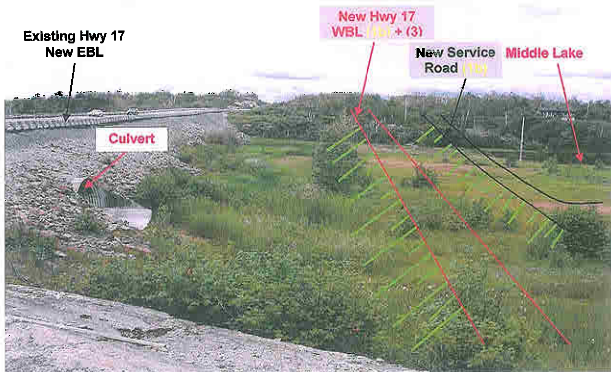
Photograph 12 VIEW: Looking west from bedrock outcrop on north side of Highway 17 at about STA. 14+550 across 200 m wide Swamp L-7 at south end of Middle Lake. Existing rockfill embankment is 12 m high. (July 5, 2006)
