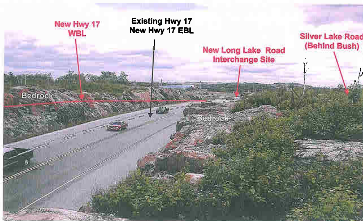
Photograph 2 VIEW: Looking east from bedrock outcrop on south side of Highway 17 at STA. 15+430, some 370 m west of the Highway 17/Sudbury MR80 (Long Lake Road) intersection. Extensive 4 m high rock cuts both sides of highway. (July 5, 2006)
