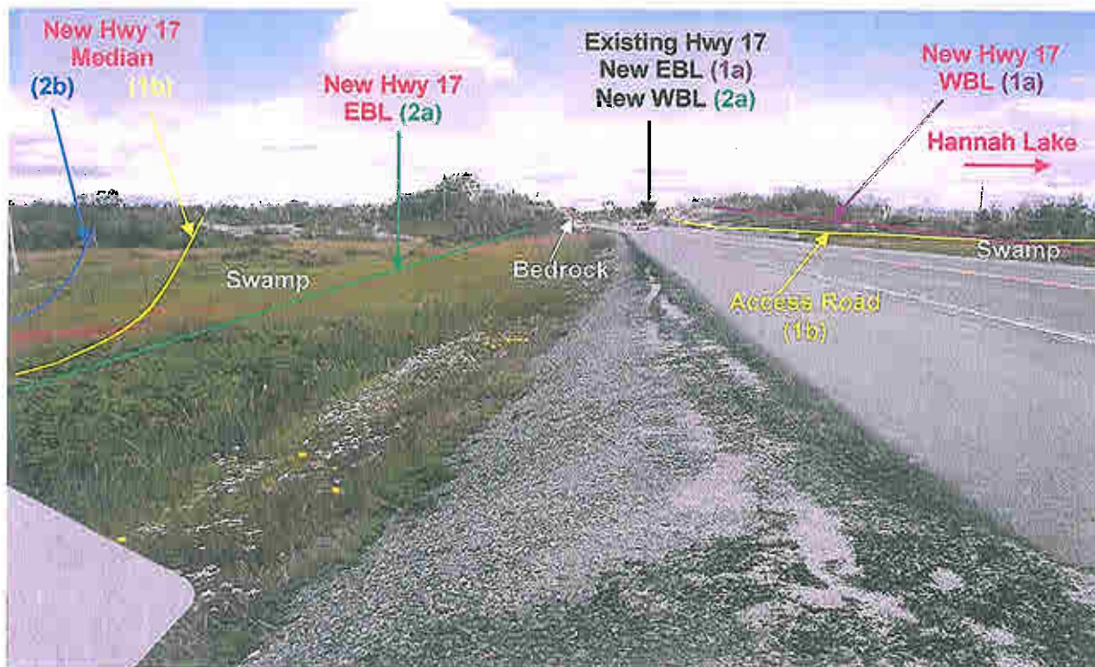
Photograph 22 VIEW: Looking west from south shoulder of Highway 17 at about STA. 12+680 at south end of extension of Hannah Lake swamp area. Bedrock outcrop in 4 to 5 m high cut in distance at STA. 12+400. (July 5, 2006)
