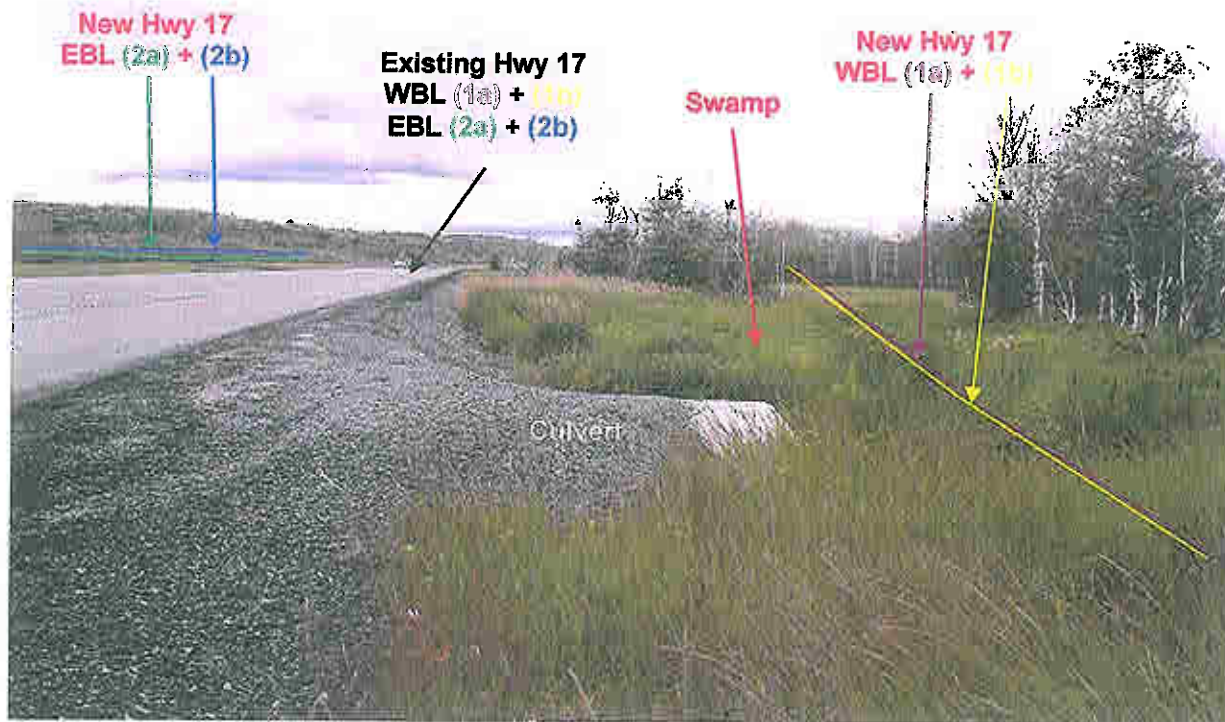
Photograph 46 VIEW: Looking west from north shoulder of Highway 17 at about STA. 18+350. Swamp L-3 exists on both sides of Highway 17. Bedrock outcrops 150 m to the north (right) at margin of Kelly Lake. (July 5, 2006)
