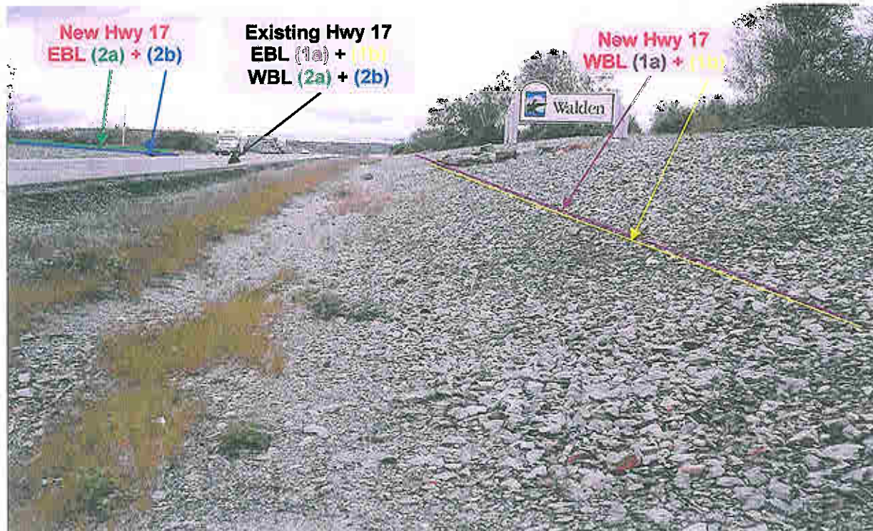
Photograph 39 VIEW: Looking west from north ditch area of Highway 17 at about STA. 10+020, near Twp Waters/Twp Broder boundary. Earth slope typically 2 to 3 m high covered with stone riprap. (July 5, 2006)
