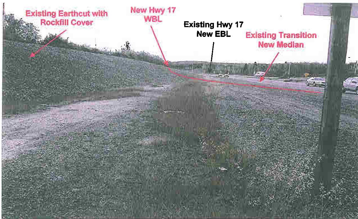
Photograph 62 VIEW: Looking east from north ditch line existing Highway 17 WBL at about STA. 15+600 some 400 m east of Highway 17/Sudbury MR 55 interchange. Existing 6 m high earth slope with stone riprap visible to north (left) of photo. (July 5, 2006)
