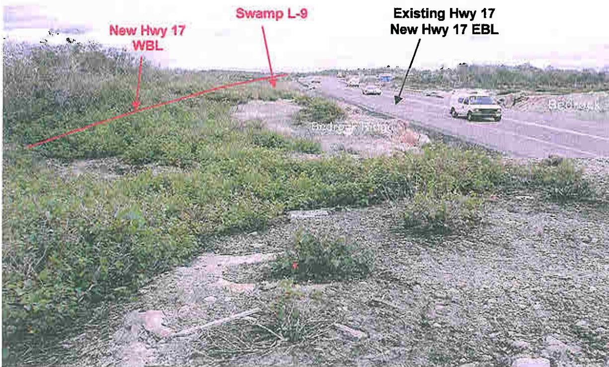
Photograph 6 VIEW: Looking east from bedrock ridge on north side of Highway 17 at about STA. 14+850. Bedrock cuts on both sides of highway. Swamp L-9 in distance at curve in road. (July 5, 2006)
