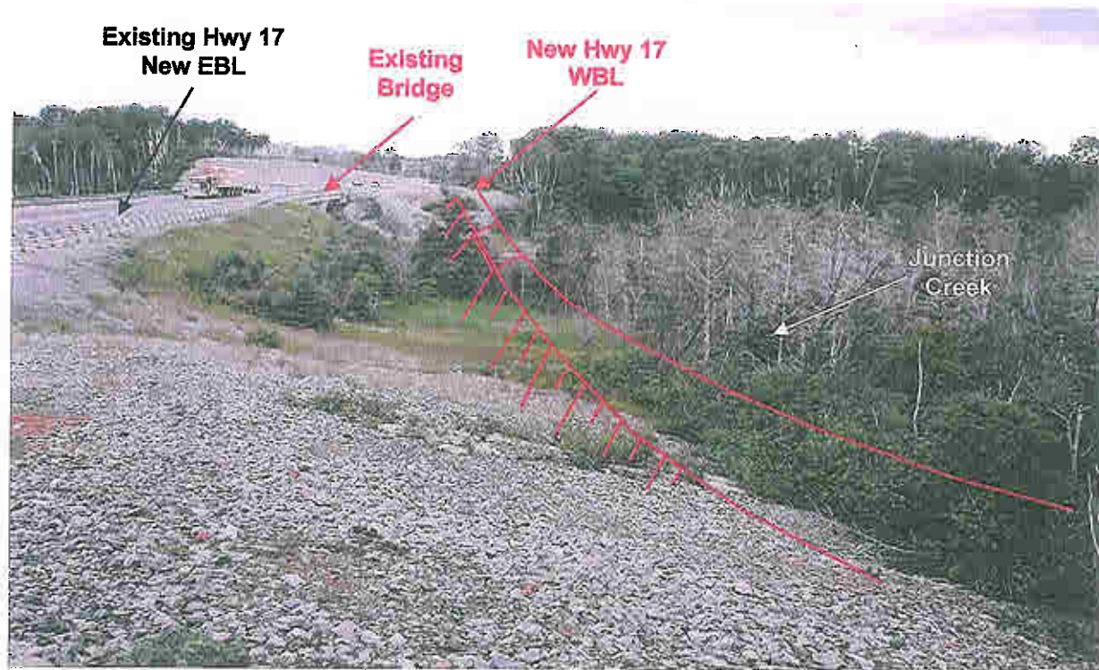
Photograph 60 VIEW: Looking west along alignment new WBL Highway 17, at about STA. 16+600, some 150 m, east of the existing Junction Creek bridge. Bedrock exposed in creek bed (west side) some 10 m below bridge deck level. (July 5, 2006)
