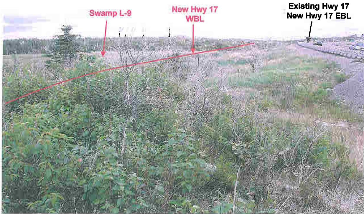
Photograph 5 VIEW: Looking east from north side of Highway 17, at about STA. 14+940, near west end of Swamp L-9. Existing highway crosses swamp via 3 to 4 m high rockfill embankment. (July 5, 2006)
