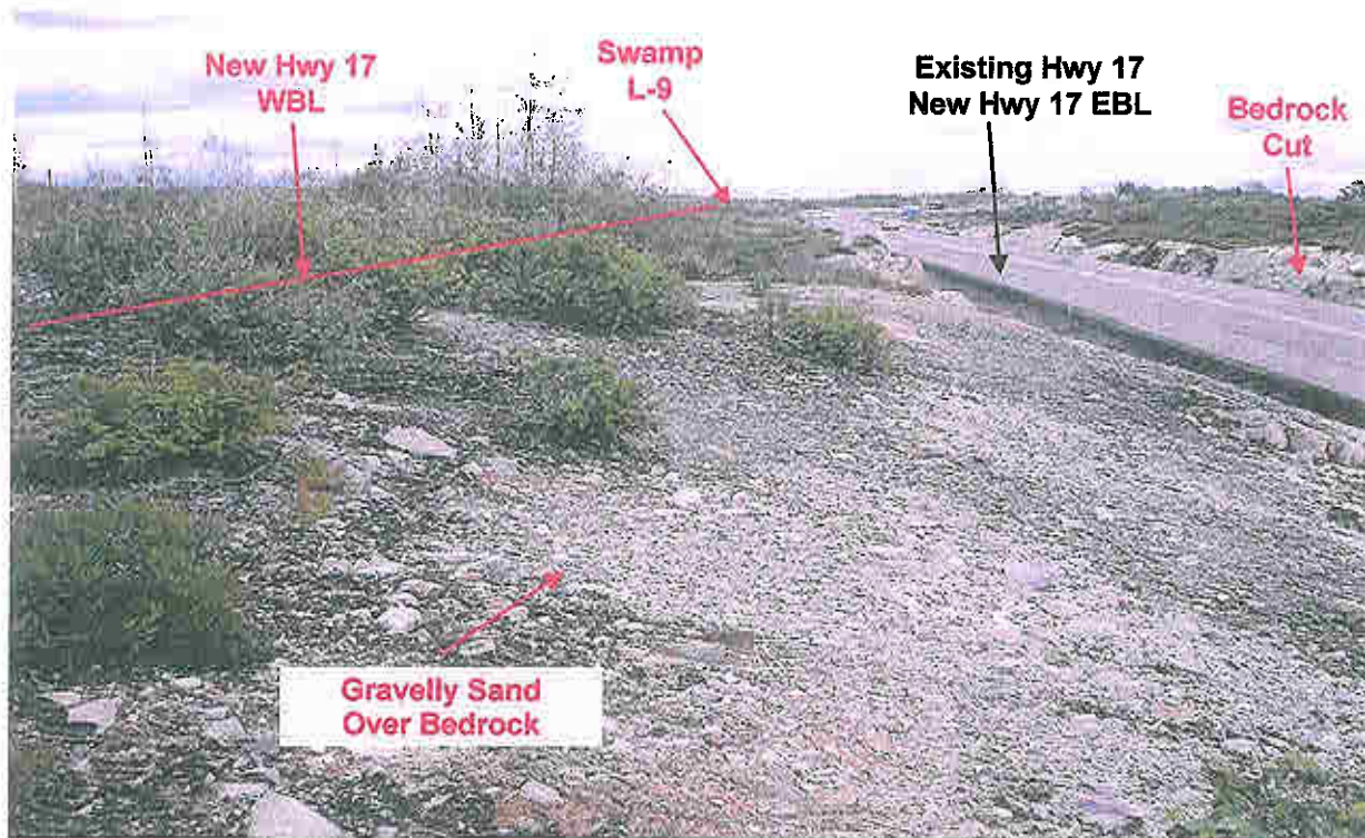
Photograph 9 VIEW: Looking east from north side of Highway 17 at about STA. 14+700. Bedrock cuts visible on both sides of highway, low bedrock ridge and swamp terrain to left side photo typical of Swamp L-7. Gravelly sand overburden mantles bedrock in foreground. (July 5, 2006)
