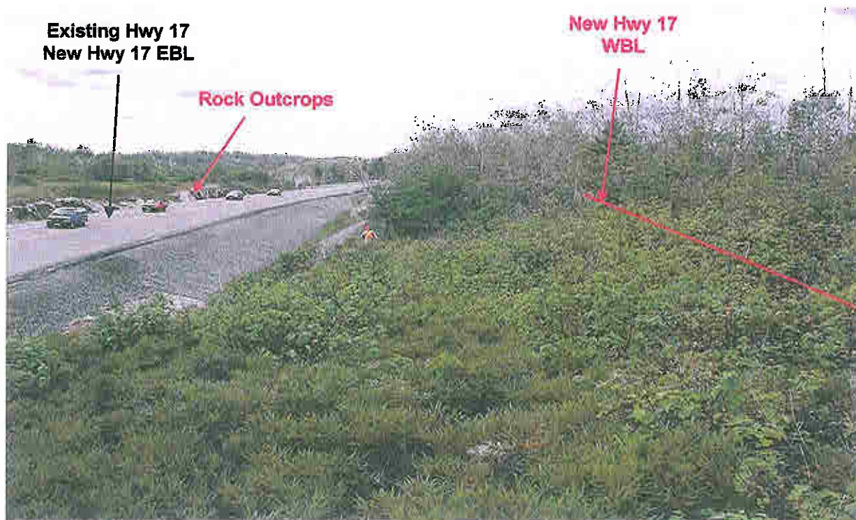
Photograph 10 VIEW: Looking to west from north side of Highway 17 at about STA. 14+700. Bedrock cuts visible both sides of highway, low bedrock ridge and swamp terrain to right side photo typical of Swamp L-8. (July 5, 2006)
