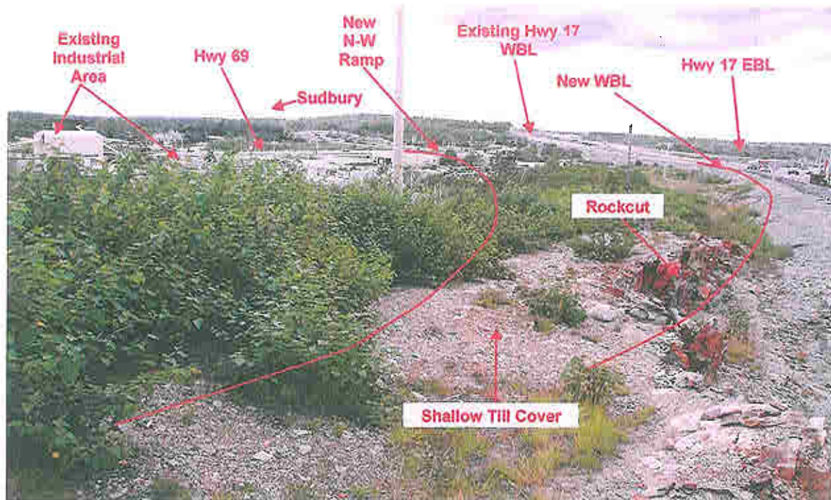
Photograph 74 VIEW: Looking easterly from STA. 18+700, top of rock cut/outcrop on north side of Highway 17. Note rock outcrop in foreground, new N-W ramp from Highway 69 through industrial area on low ground in centre of photograph and start of new WBL from existing WBL at Highway 69 crossing. (July 05, 2006)
