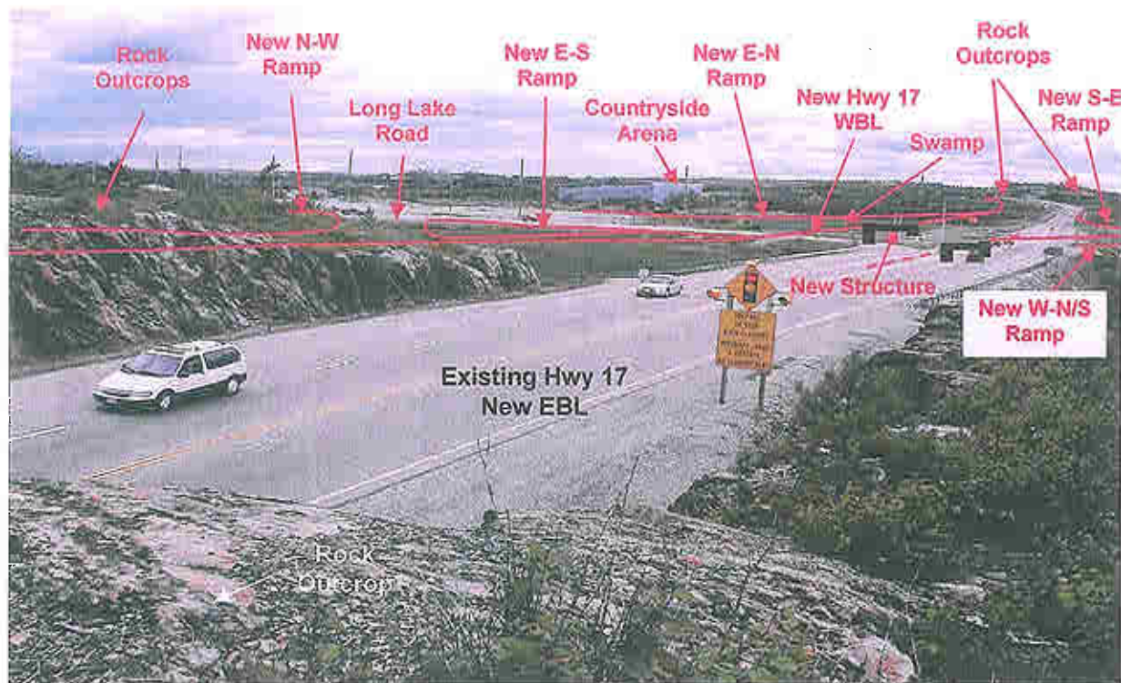
Photograph 64 VIEW: Looking east from top of rock cut on south side of Highway 17 at about STA. 15+600, 200 m west of Highway 17/Long Lake Road intersection. Note the alignment of new Highway 17 North twinning through swamp and rock outcrop. (July 5, 2006)
