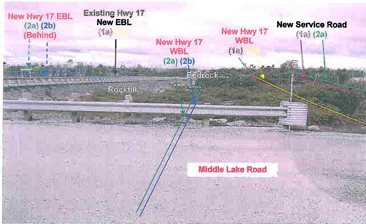
Photograph 14 VIEW: Looking west from east side of Middle lake Road about 10 m north of Highway 17. Low bedrock ridge and shallow swamp terrain in middle of photo. Bedrock outcrop exposed in 6 to 8 m cut on both sides of road in distance at about STA. 13+050. (July 5, 2006)
