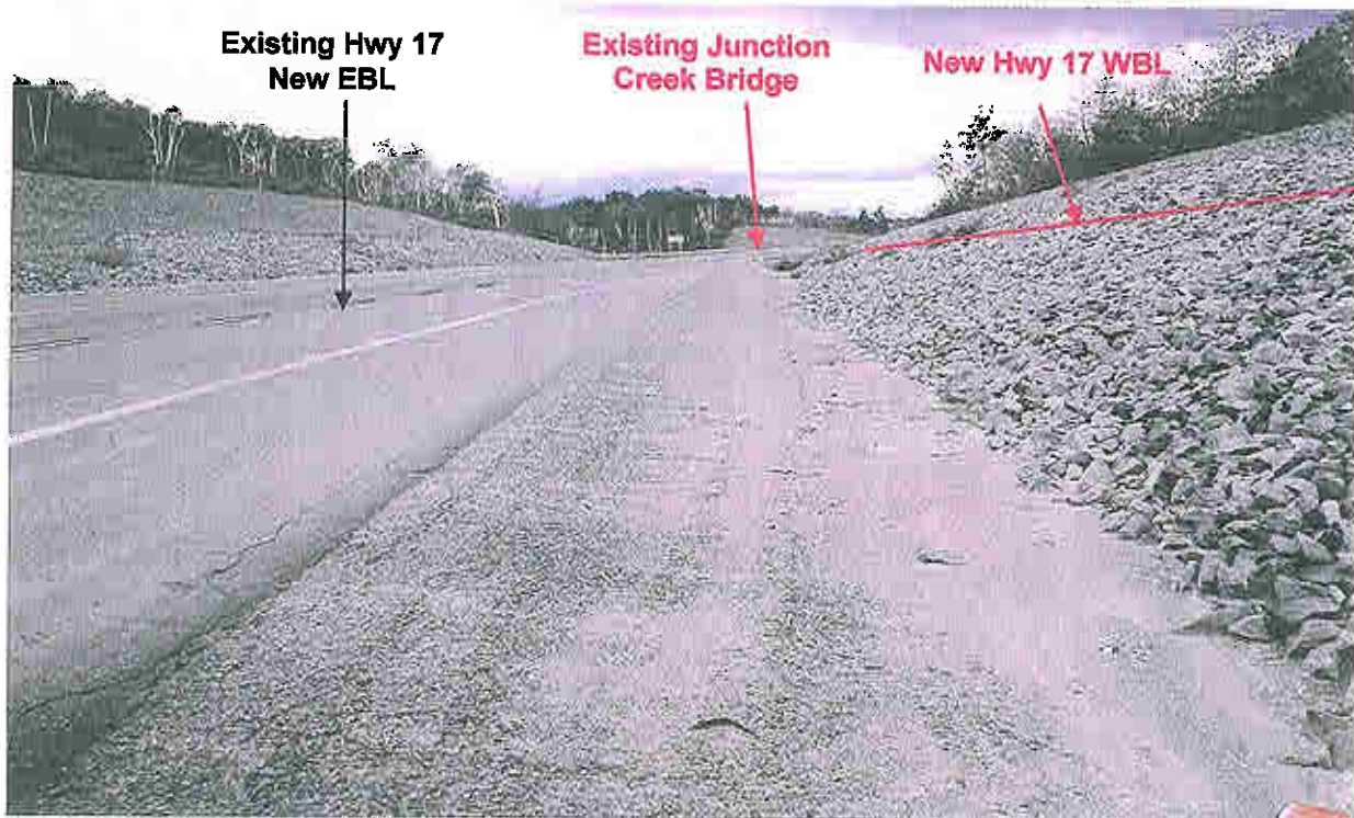
Photograph 59 VIEW: Looking west from north shoulder of Highway 17 at STA. 16+800, at about 350 m east of the existing Junction Creek bridge. No bedrock exposures in view. Existing 6 m high earthslopes with stone riprap visible both sides of highway. (July 5, 2006)
