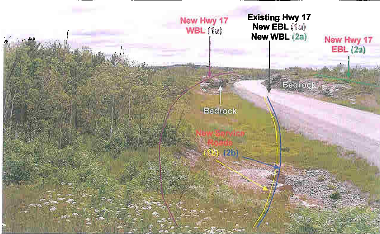
Photograph 23 VIEW: Looking east from bedrock outcrop on north side of Highway 17, at about STA. 12+050. Extensive bedrock exposures readily visible in 4 m high rock cuts at STA. 12+200 to 12+300 mid photo. (July 5, 2006)
