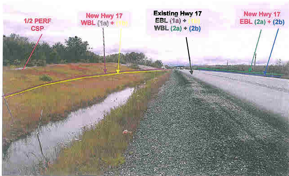
Photograph 41 VIEW: Looking east along north ditch line of Highway 17 at about STA. 18+750. North earth slope grassed then provided with stone riprap. Bedrock outcrops to north (left) beyond R.O.W. limits. Swamp area exists on south side of Highway 17. (July 5, 2006)
