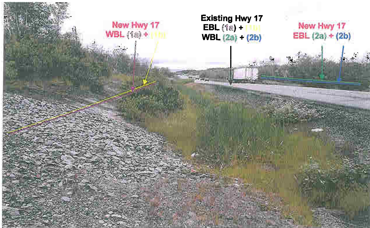
Photograph 38 VIEW: Looking east from north ditch area of Highway 17 at about STA. 10+020. Earth slope and stone riprap visible in foreground left. Swamp area for twinning to the south beyond truck in photo. (July 5, 2006)
