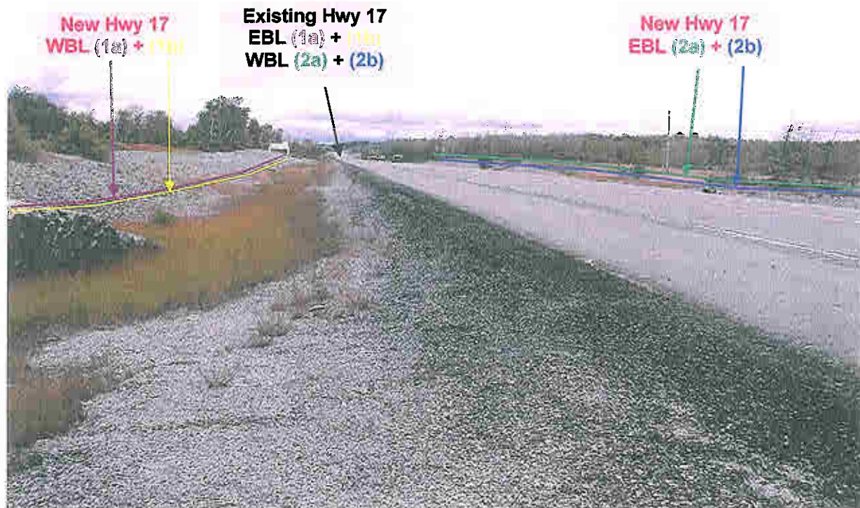
Photograph 40 VIEW: Looking east from north ditch of Highway 17 at about STA. 18+950. Earth slopes typically 2 to 3 m high covered with stone riprap. Bedrock outcrop to north (left) beyond R.O.W. limit. (July 5, 2006)
