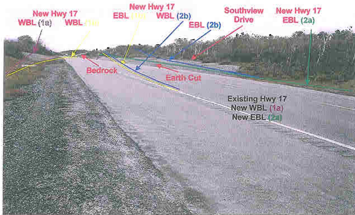
Photograph 36 VIEW: Looking east from north shoulder of Highway 17 at about STA. 10+475. Earth slope covered with stone riprap on south side of highway. Bedrock outcrop visible on distance at Sta. 11+000. (July 5, 2006)
