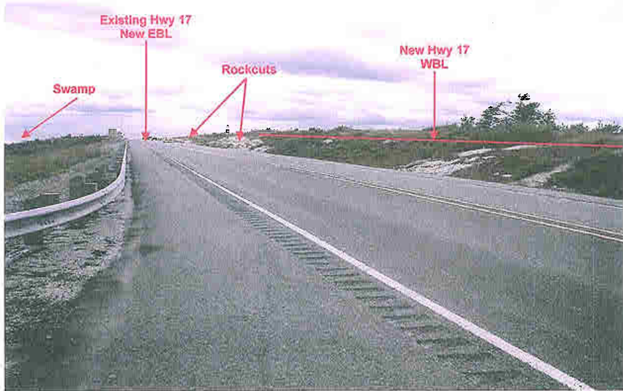
Photograph 70 VIEW: Looking westerly from STA. 18+120, south shoulder of Highway 17. Note new Highway 17 WBL alignment over a rock outcrop, swamp exist 40 to 80m beyond guardrail along south side of existing Highway. (July 05, 2006)
