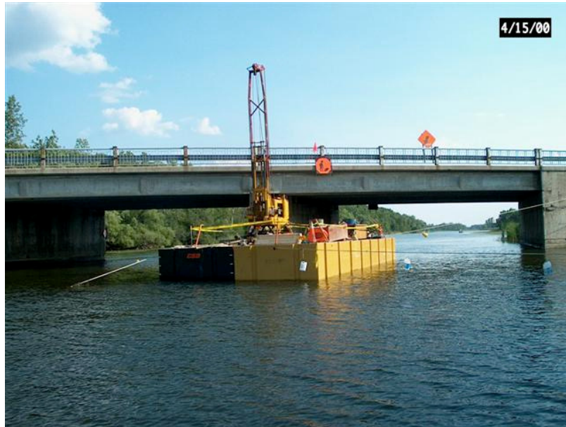
Photograph 7 – Drill and barge setup prior to drilling at east pier.
