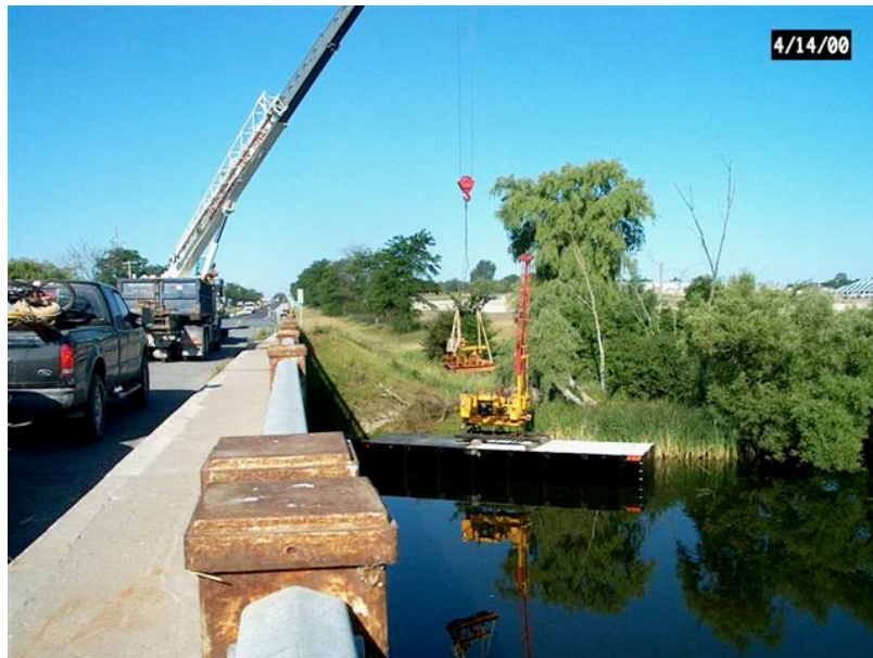
Photograph 6 – View of drill and barge set up in the river.
