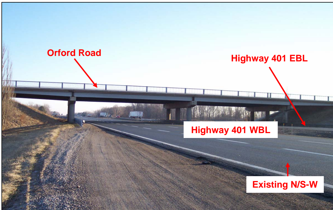
PHOTOGRAPH 5-16: Orford Road I/C. Looking east at Orford Road underpass structure. Note typical 4-span steel girder structure and N/S-W on ramp. (January 27, 2006)
