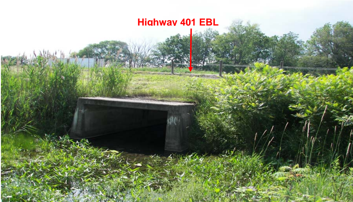
PHOTOGRAPH 5-27: Culvert Site 13-422. Looking northwesterly at south end of culvert. Note shallow embankment over top of culvert. (June 29, 2006)
