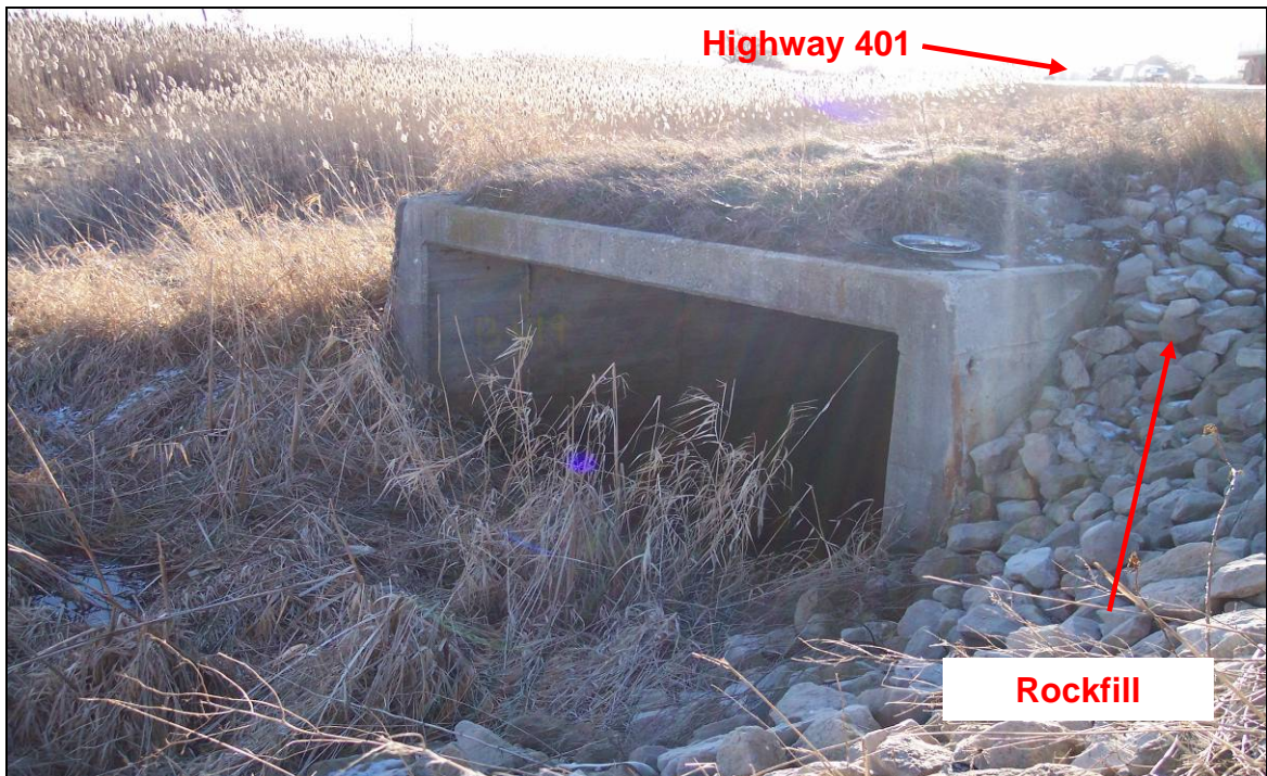
PHOTOGRAPH 5-10: Culvert Site 13-419. Looking north-westerly at south end of culvert. Note erosion controlled with rockfill cover. (January 26, 2006)
