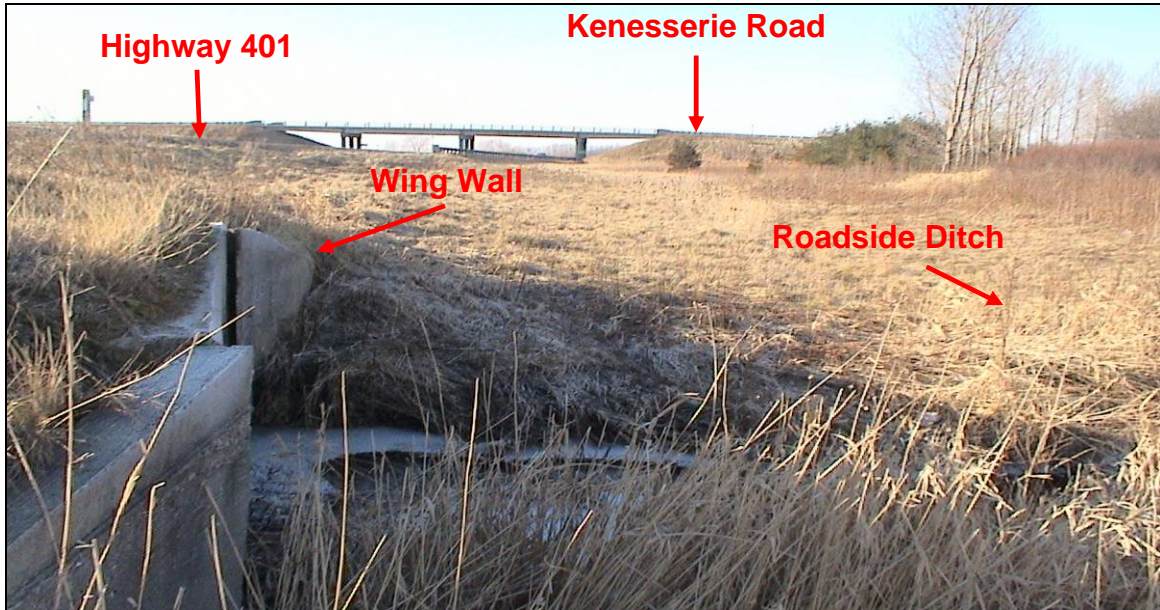
PHOTOGRAPH 5-7: Culvert Site 13-418. Looking west across top of north end of culvert and wing walls. Kenesserie Road Underpass in the distance. Note flat roadside ditch beyond channel. Note displacement of wing walls. (January 27, 2006)
