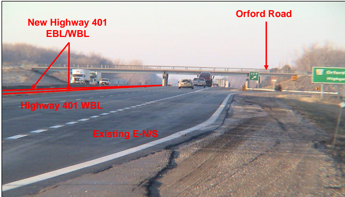
PHOTOGRAPH 5-15: Orford Road I/C. Looking west at interchange from the E-N/S exit ramp. Note high approach embankment fills and generally level terrain. Preferred Option: Future Highway 401 EBL and WBL depicted. (January 27, 2006)
