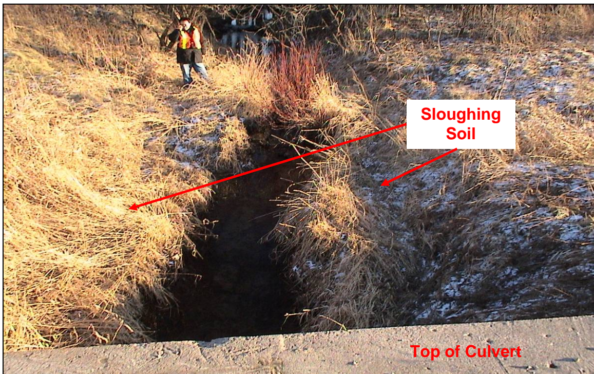
PHOTOGRAPH 5-14: Culvert Site 13-421. Looking south across top of south end of culvert. Note silted-in channel and possible sloughing of west bank. (January 26, 2006)
