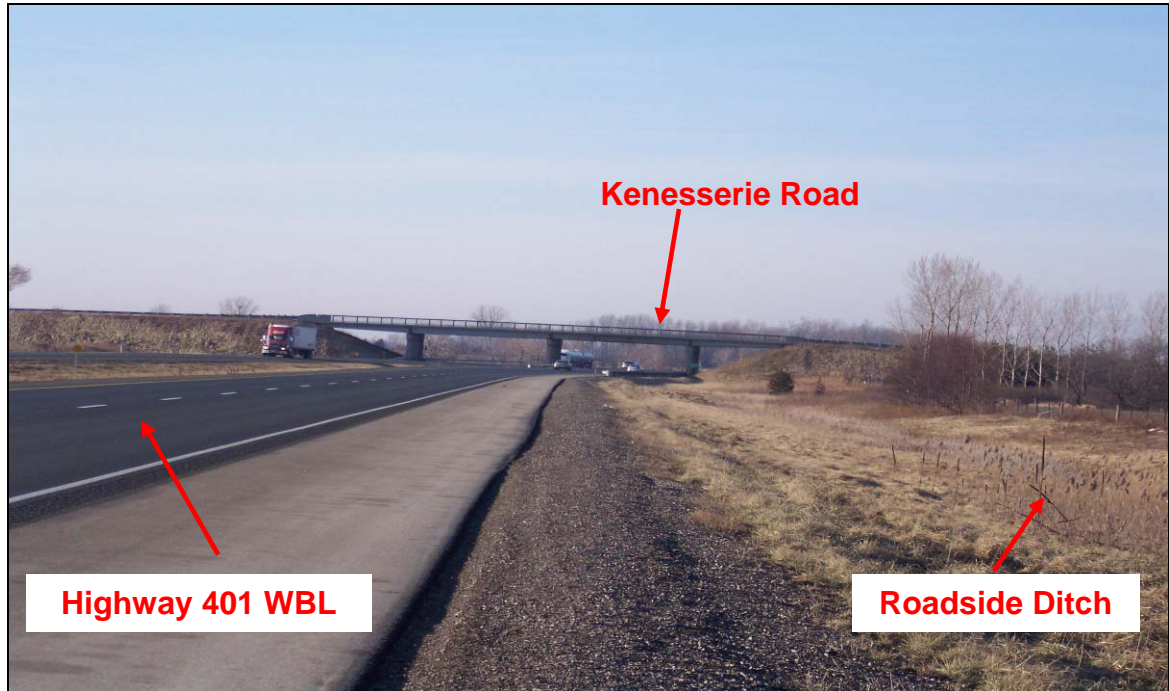
PHOTOGRAPH 5-1: Kenesserie Road Underpass. Looking west from north shoulder of Highway 401. Note both approach embankments built on fill over nearly flat terrain. (January 27, 2006)
