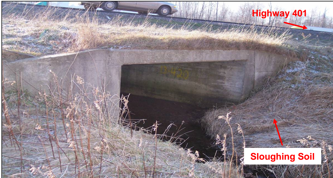
PHOTOGRAPH 5-11: Culvert Site 13-420. Looking southwesterly at north end of culvert. Note siltation of channel possibly caused by sloughing of west side of earth channel. (January 27, 2006)
