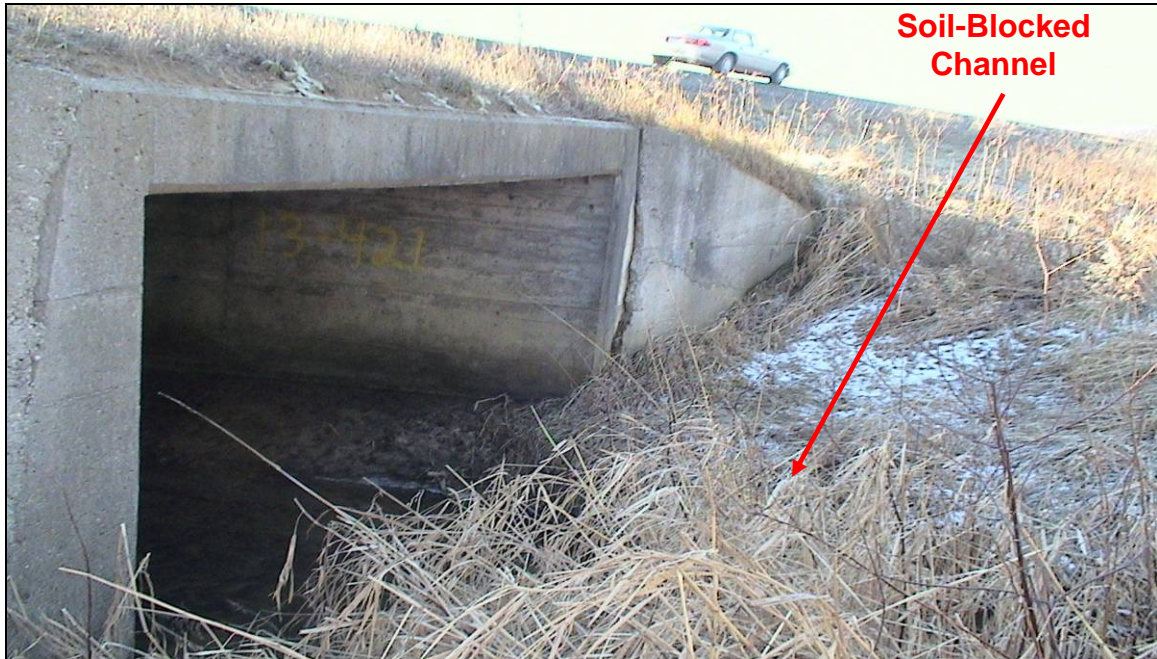
PHOTOGRAPH 5-13: Culvert Site 13-421. Looking south-westerly at north end of culvert. Note partly blocked channel. (January 27, 2006)
