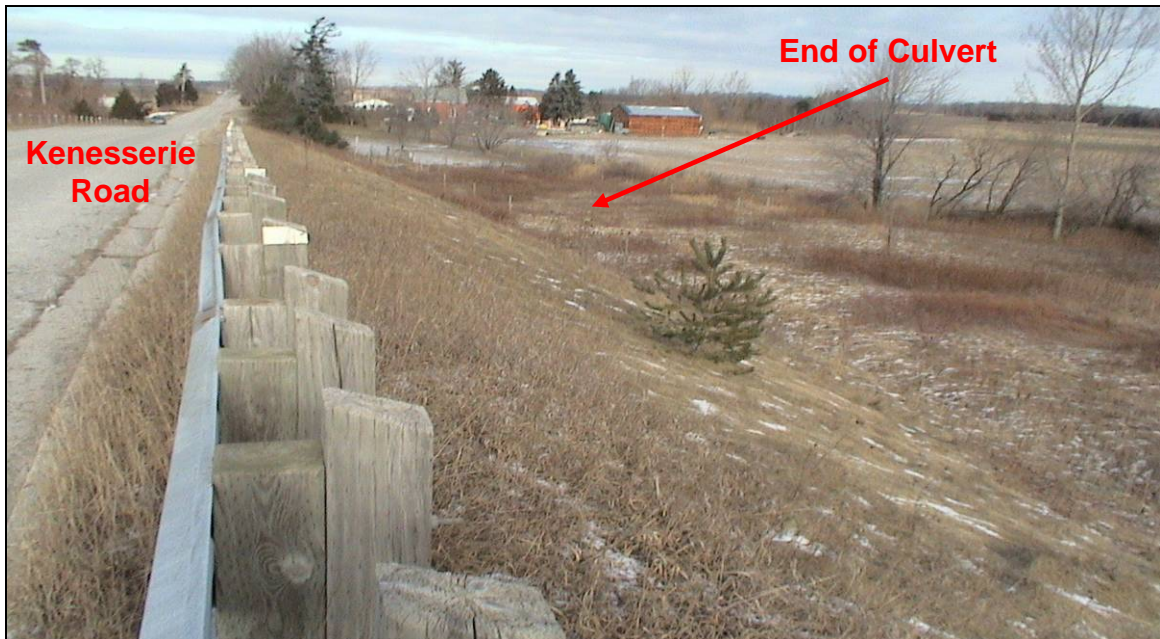
PHOTOGRAPH 5-4: Kenesserie Road Underpass. Looking north from top of north approach embankment, east side. Note farm buildings and gently rolling terrain. End of culvert crossing road is visible at toe of slope. (January 26, 2006)
