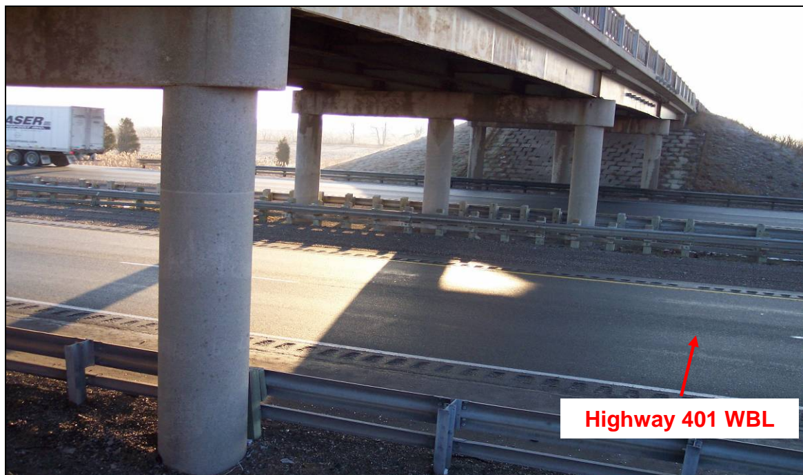
PHOTOGRAPH 5-22: Duart Road Underpass. Looking south across Highway 401 from north abutment. Note wide median shoulder and four-span structure type. (January 27, 2006)
