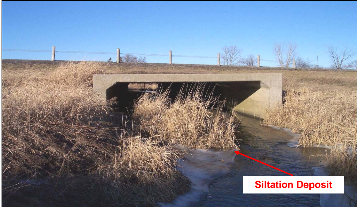
PHOTOGRAPH 4-39: Culvert 13-415. Looking northeasterly at south end of culvert. Note partially blocked channel due to siltation at end of culvert. (January 26, 2006)
