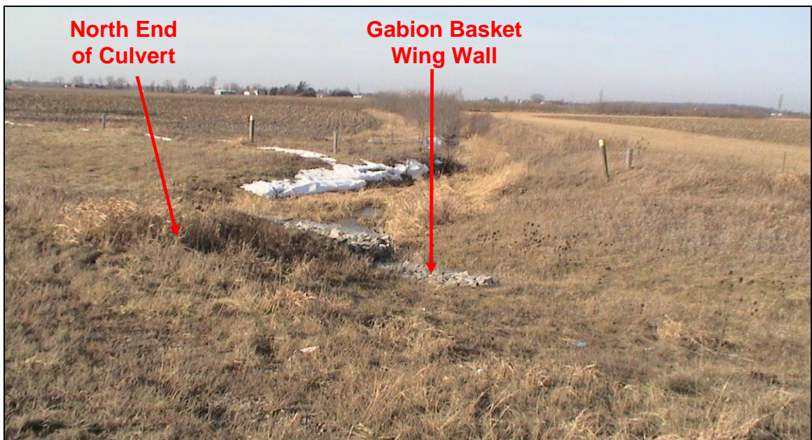
PHOTOGRAPH 4-14: Culvert 13-409. Looking north across top of north end of culvert. Note gabion basket used for east wing wall (same for west side). Note gently undulating terrain beyond Highway 401 R.O.W. and farming land use. (January 27, 2006)
