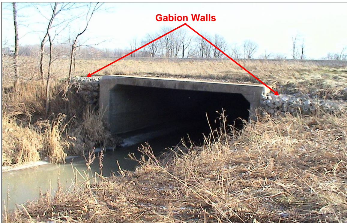
PHOTOGRAPH 4-28: Culvert 13-413. Looking southeasterly at north end of culvert. Note gabion basket wing walls. (January 27, 2006)
