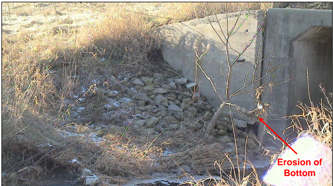
PHOTOGRAPH 4-16: Culvert 13-410. Looking west at west wing wall of south end of culvert. Note leaning wall, erosion at bottom of wall and rock fill cover placed for erosion protection. (January 26, 2006)
