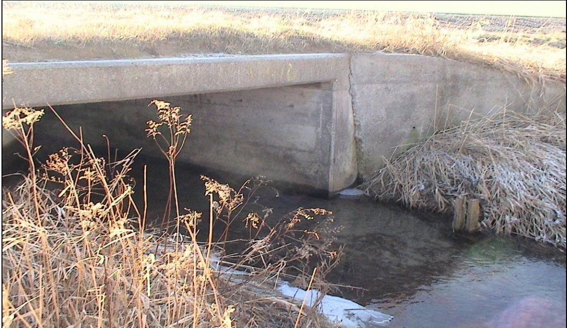
PHOTOGRAPH 4-41: Culvert 13-416. Looking westerly at north end of culvert. Note minor sloughing of bank in foreground. (January 27, 2006)
