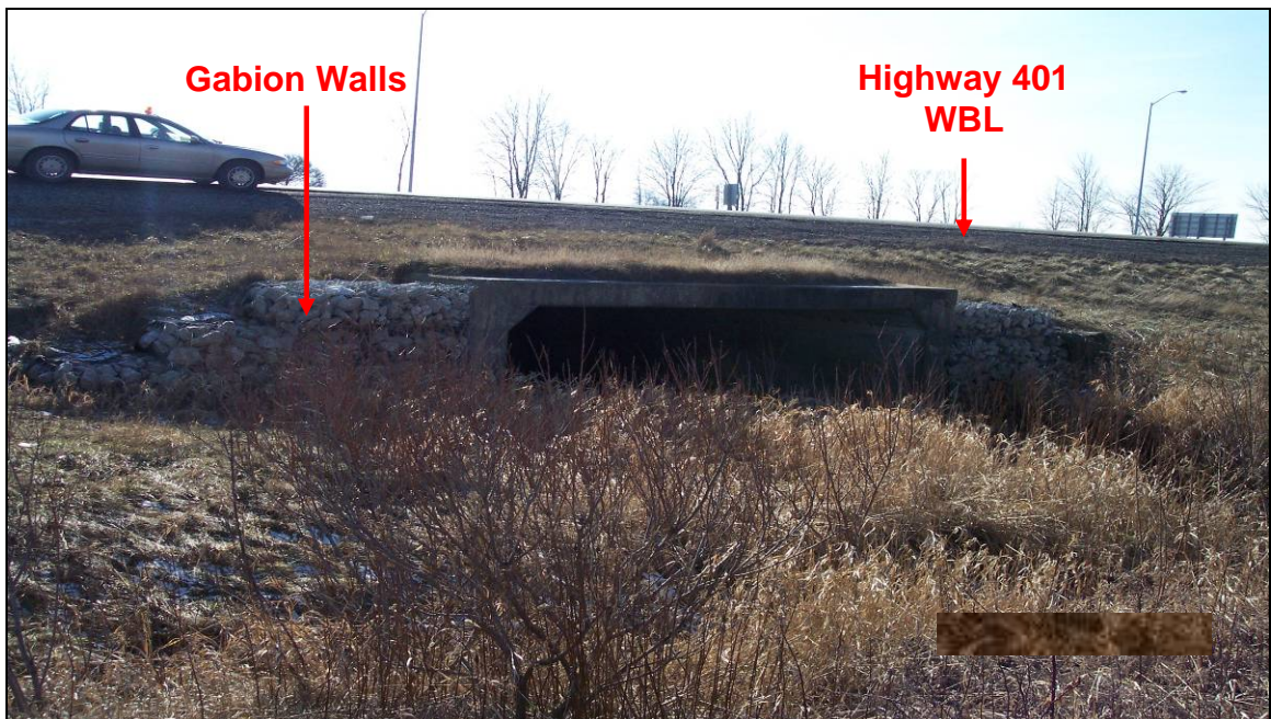
PHOTOGRAPH 4-30: Culvert 13-414. Looking southerly at north end of culvert. Note gabion basket detail and low Highway 401 embankment over top of culvert. (January 27, 2006)
