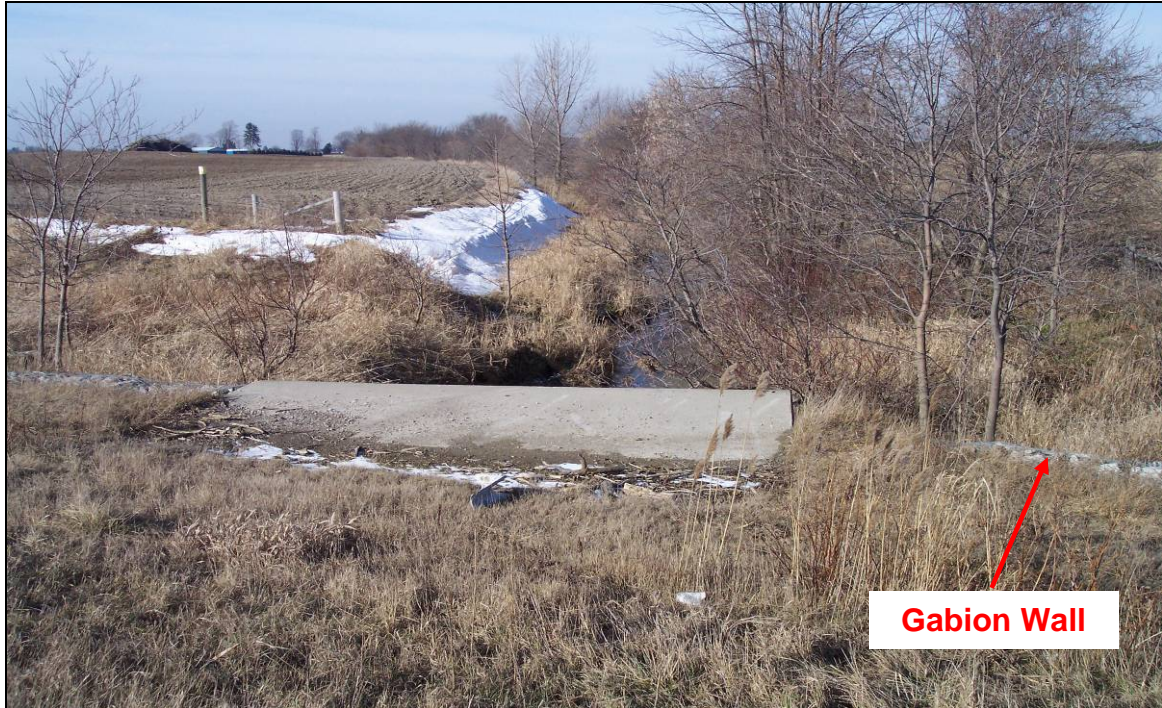
PHOTOGRAPH 4-17: Culvert 13-410. Looking north across top of north end of culvert. Note gabion baskets used for wing walls, deep drainage channel. (January 27, 2006)
