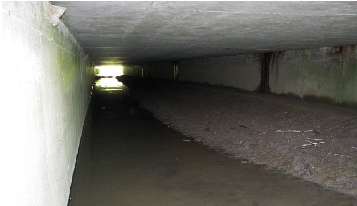
PHOTOGRAPH 4-10: Culvert 13-407. View through culvert from south end. Note continuous construction. (June 29, 2006)
