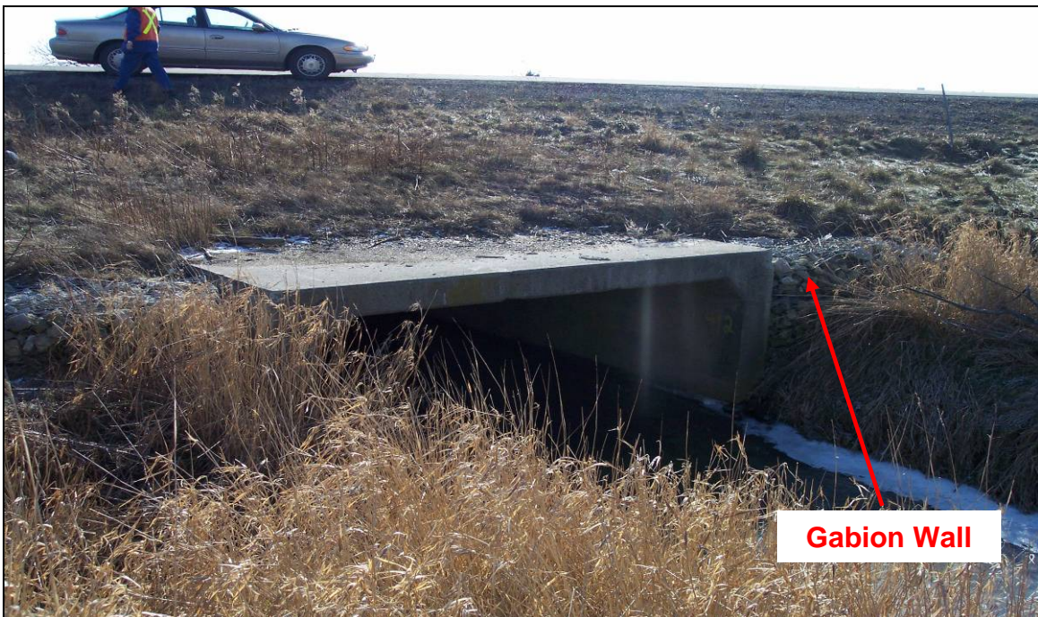
PHOTOGRAPH 4-26: Culvert 13-412. Looking southeasterly at north end of culvert. Note wing walls made up of gabion basket walls. (January 27, 2006)
