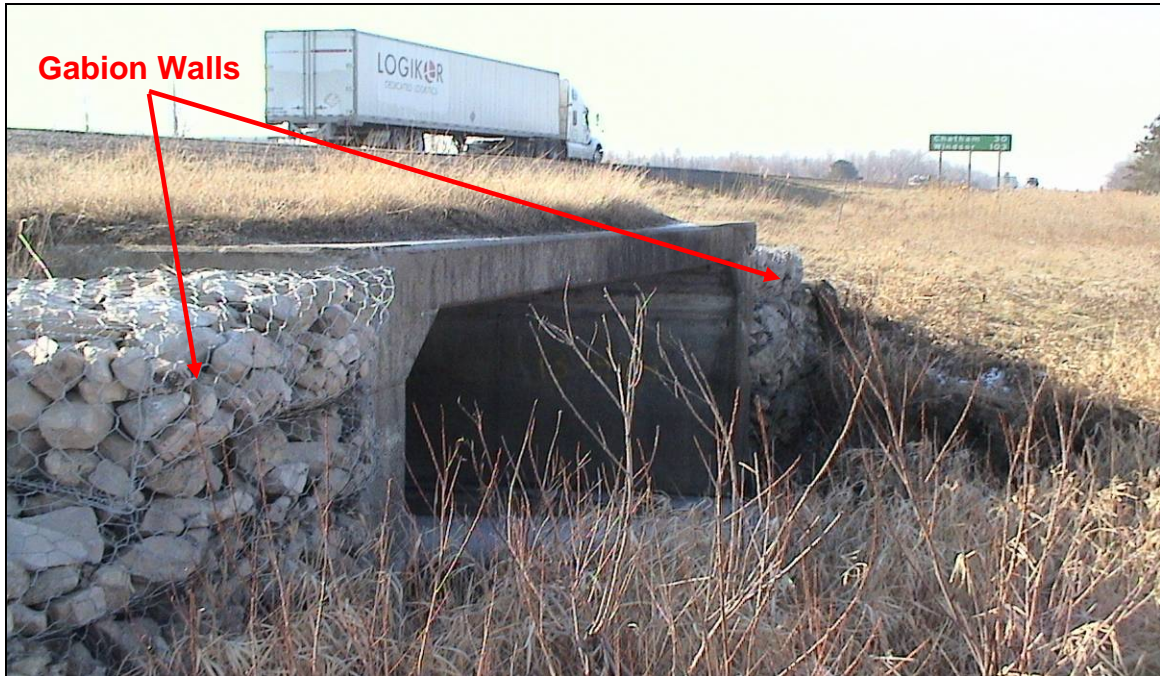
PHOTOGRAPH 4-29: Culvert 13-414. Looking southwesterly at north end of culvert. Note gabion basket used for wing walls. (January 27, 2006)
