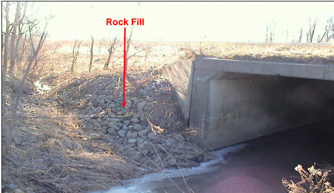
PHOTOGRAPH 4-27: Culvert 13-413. Looking northwesterly at south end of culvert. Note rock fill cover placed on roadside ditch and beside culvert to control erosion. (January 26, 2006)
