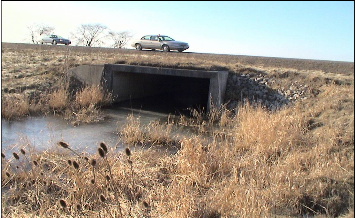
PHOTOGRAPH 4-13: Culvert 13-409. Looking north at south end of culvert. Note east wing wall replaced with rock fill cover. Shallow road embankment over top of culvert, grass covered roadside ditches. (January 26, 2006)
