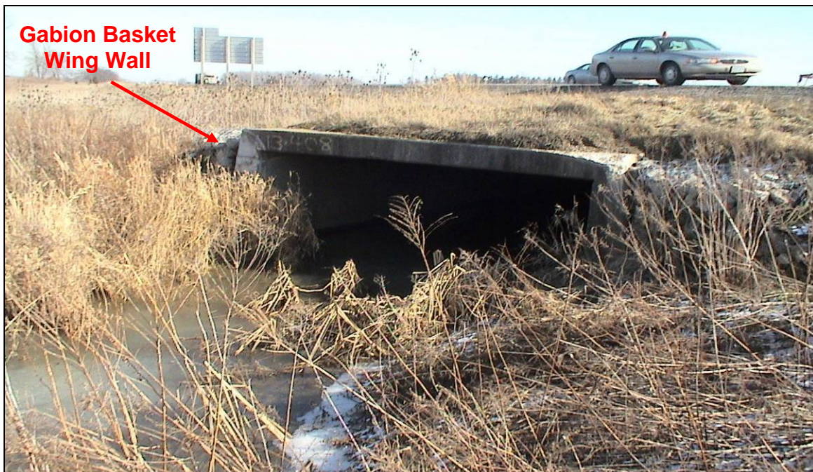
PHOTOGRAPH 4-12: Culvert 13-408. Looking southeasterly at north end of culvert. Note wide channel and gabion baskets used for wing walls. (January 27, 2006)
