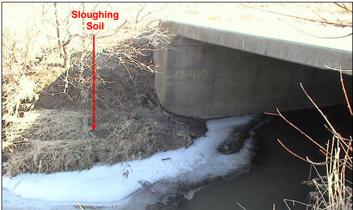
PHOTOGRAPH 4-18: Culvert 13-410. Looking east at north end of culvert. Note sloughing soil partially blocking the drainage channel. (January 27, 2006)
