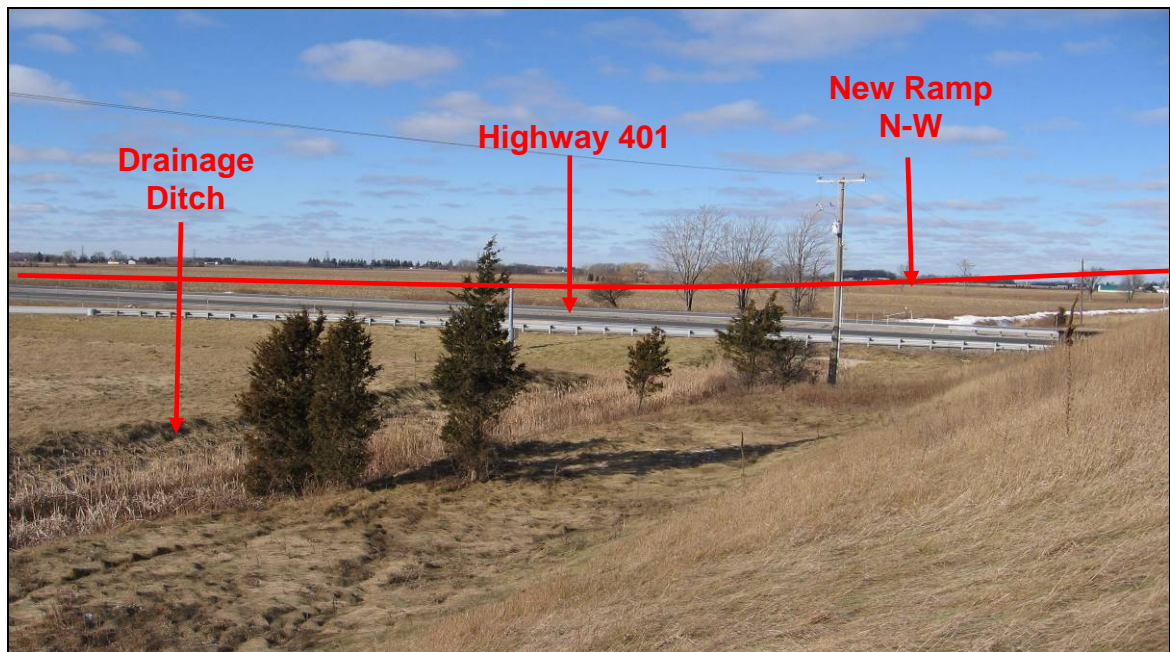
PHOTOGRAPH 4-4: Kent Bridge Road Interchange. Looking northwesterly from mid slope of south approach embankment. Note flat terrain, drainage ditch along evergreens south of Highway 401. Snow demarks drainage ditch north of highway. Preferred Option: Future N-W ramp is depicted. (January 26, 2006)
