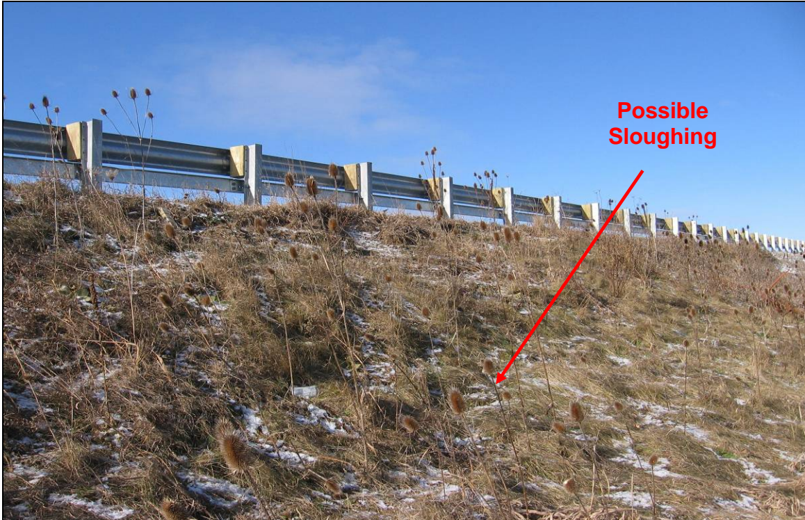
PHOTOGRAPH 4-23: Scane Road Underpass. Looking at east slope of south approach embankment. Note rough appearance indicating possible surficial sloughing. (January 26, 2006)
