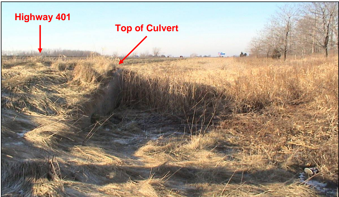
PHOTOGRAPH 4-42: Culvert 13-416. Looking west along sideroad ditch. Note heavy grass cover of ditches, flat terrain in background. (January 27, 2006)
