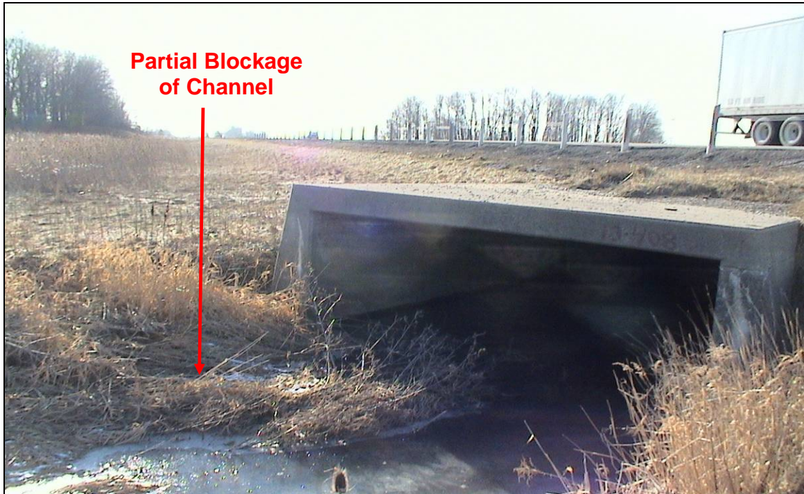
PHOTOGRAPH 4-11: Culvert 13-408. Looking northwesterly at south end of culvert. Note partial blockage of channel on west side. (January 26, 2006)
