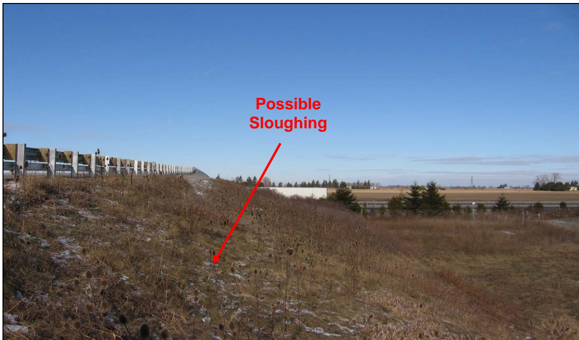
PHOTOGRAPH 4-22: Scane Road Underpass. Looking north at east slope of south approach embankment. Note possible surficial soil sloughing in foreground. (January 26, 2006)
