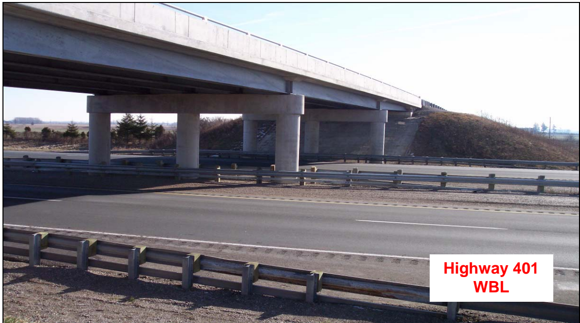
PHOTOGRAPH 4-20: Scane Road Underpass. Looking southeasterly from north shoulder of Highway 401. Note good condition of foundations, typically flat terrain in background. (January 27, 2006)
