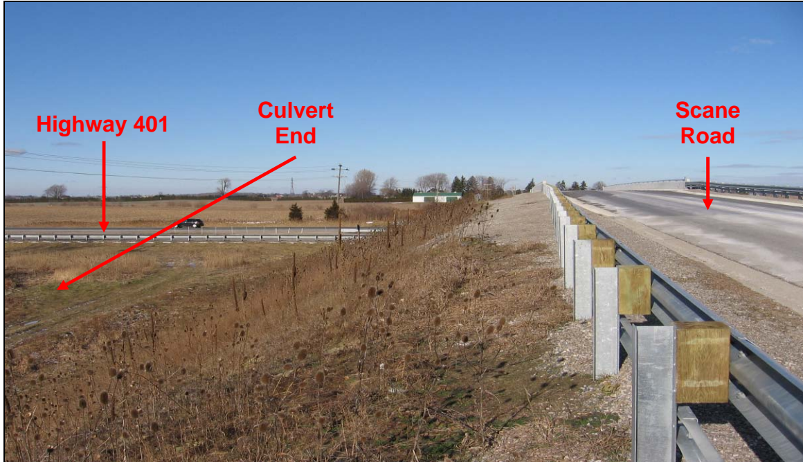
PHOTOGRAPH 4-21: Scane Road Underpass. Looking north along west side of south approach embankment. Note gravel cover on top of slope from 2005 bridge rehabilitation work in foreground. Note flat terrain beyond bridge and culvert end at left centre of photograph. (January 26, 2006)
