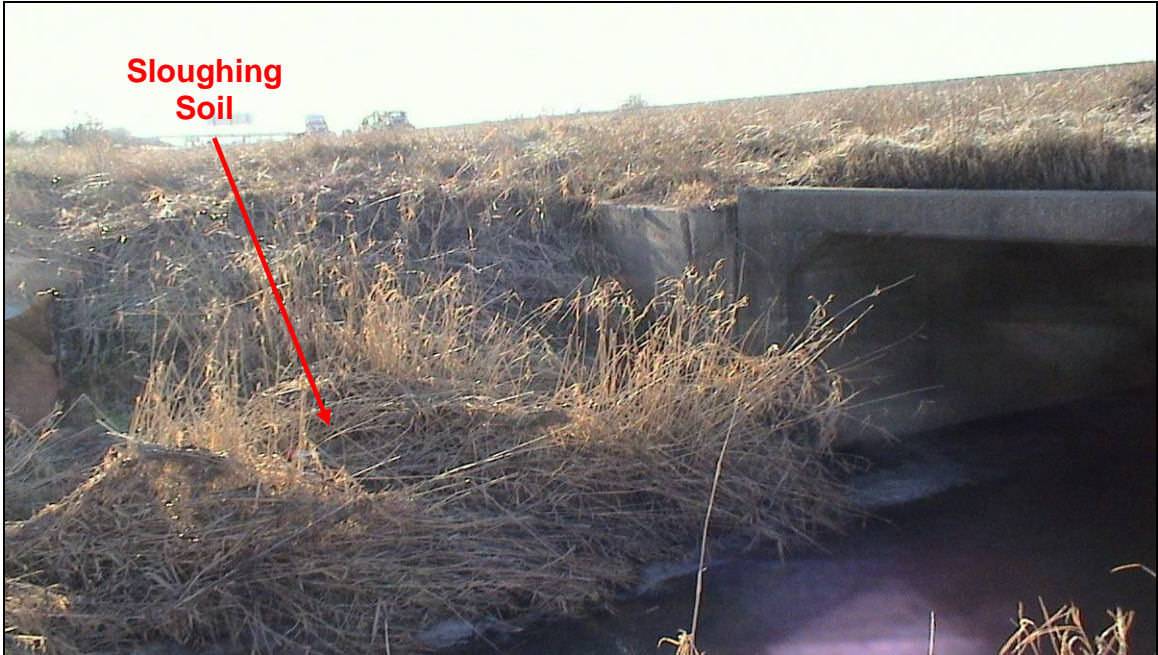
PHOTOGRAPH 4-25: Culvert 13-412. Looking west at south end of culvert. Note leaning west wing wall and soil sloughing into channel. (January 26, 2006)
