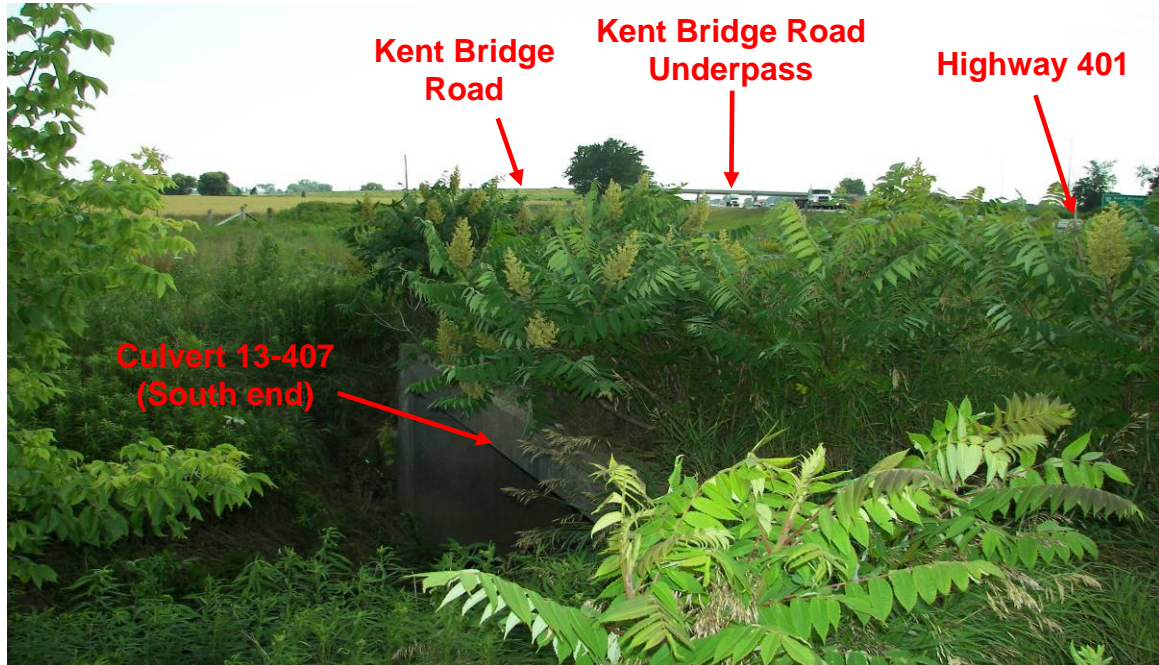
PHOTOGRAPH 4-9: Culvert 13-407. Looking westerly at south end of culvert 13-407. Note flat terrain beyond culvert ditch and south approach embankment to Kent Bridge Road underpass. (June 29, 2006)
