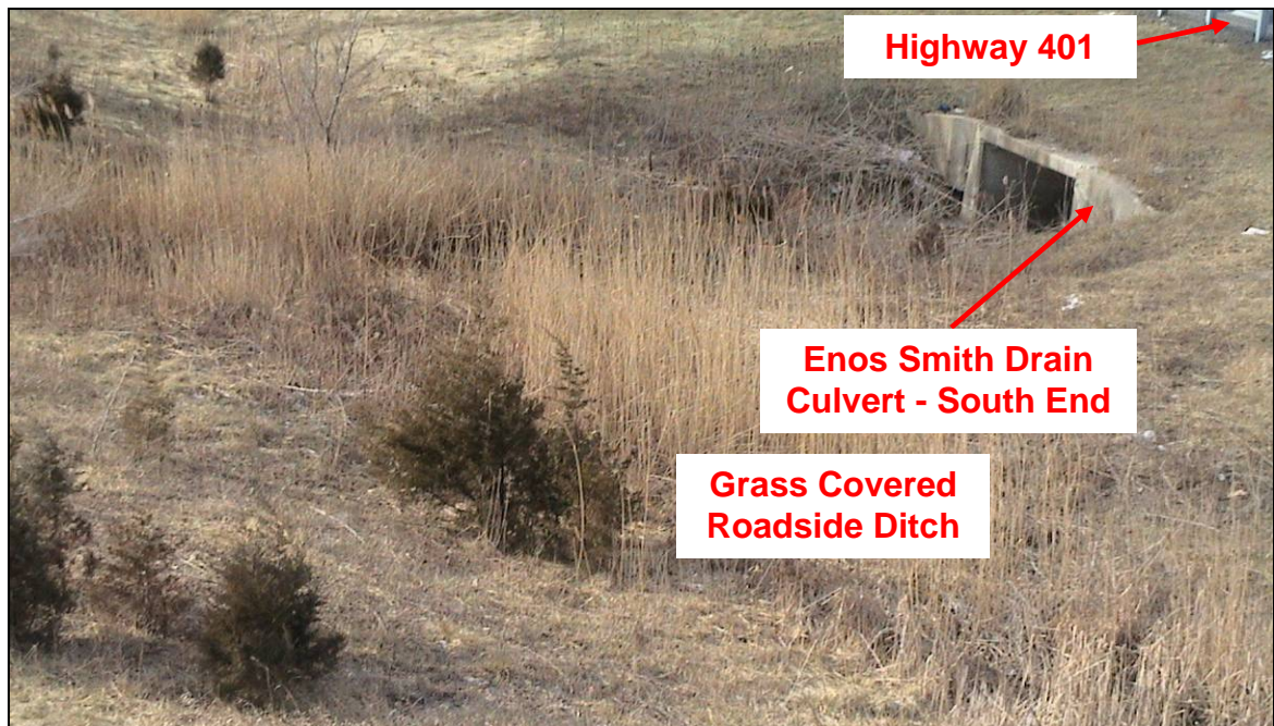
PHOTOGRAPH 3-36: Enos Smith Drain Culvert. Looking westerly at south end of Enos Smith Drain Culvert from south approach embankment of Mull Road Underpass. Note concrete wing walls and grass covered roadside ditch. (January 27, 2006)
