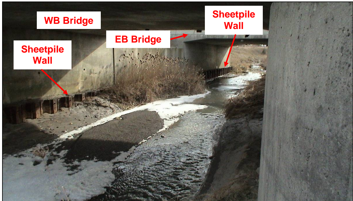
PHOTOGRAPH 3-15: McGregor Creek Bridges. Close-up of McGregor Creek EB and WB bridges. Note top of sheet-pile wall in front of abutment foundations. (January 27, 2006)
