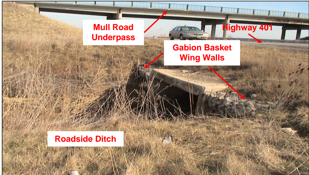
PHOTOGRAPH 3-35: Enos Smith Drain Culvert. Looking easterly at north end of Enos Smith Drain Culvert with Mull Road underpass in the background. Note gabion basket wing walls, grass covered roadside ditch. (January 27, 2006)
