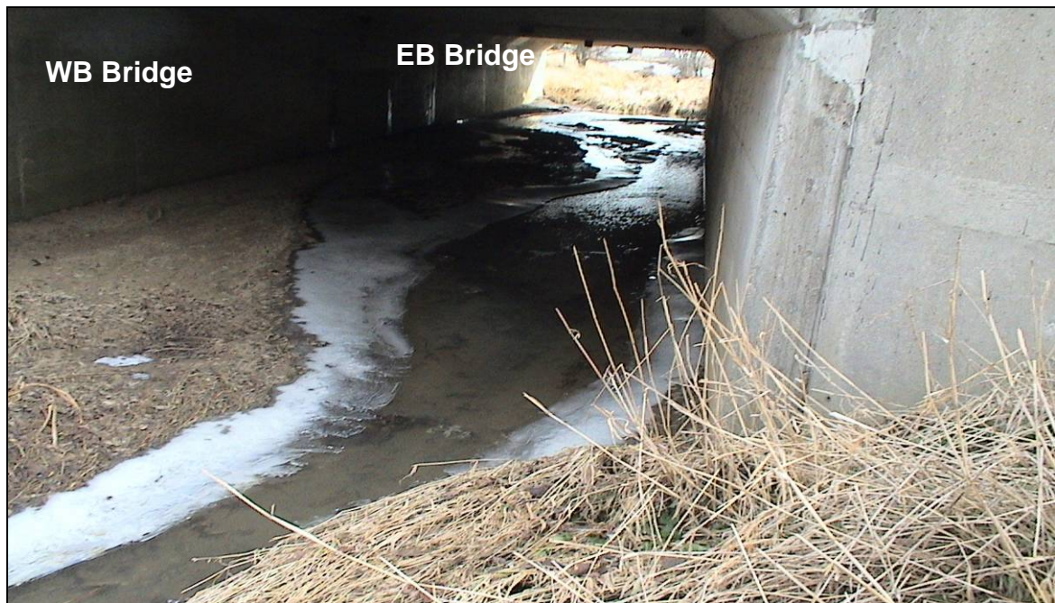
PHOTOGRAPH 3-18: Proctor Drain Bridges. Looking south along WB and EB Bridges crossing the Proctor Drain. Note continuous roof slab and meandering channel of drain. (January 27, 2006)
