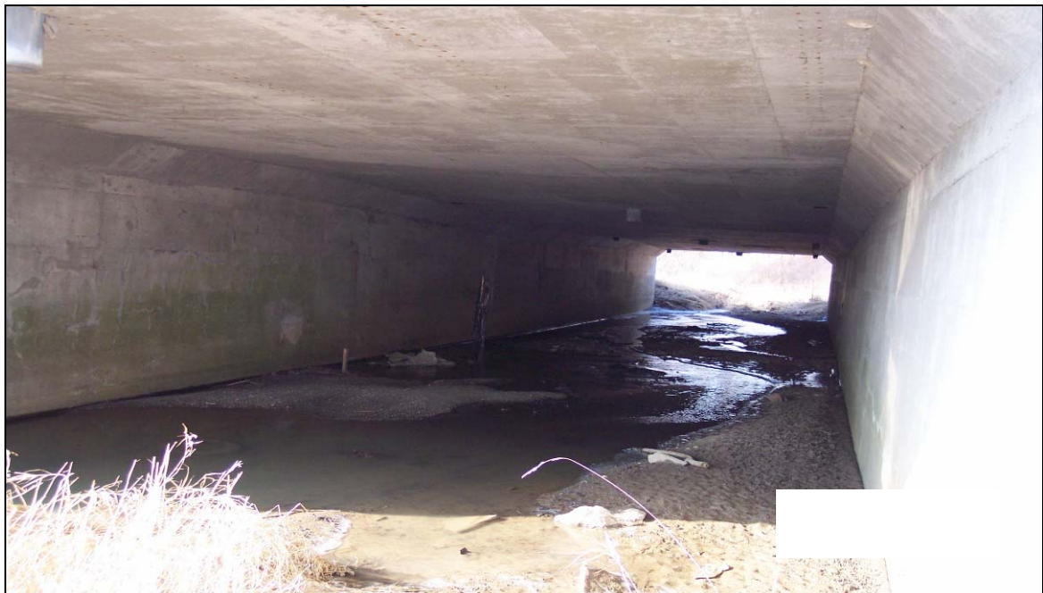
PHOTOGRAPH 3-20: Proctor Drain Bridges. Looking north from south end of EB Bridge crossing Proctor Drain. Note single roof slab construction. Note meandering channel of drain under and north of bridges. (January 26, 2006)
