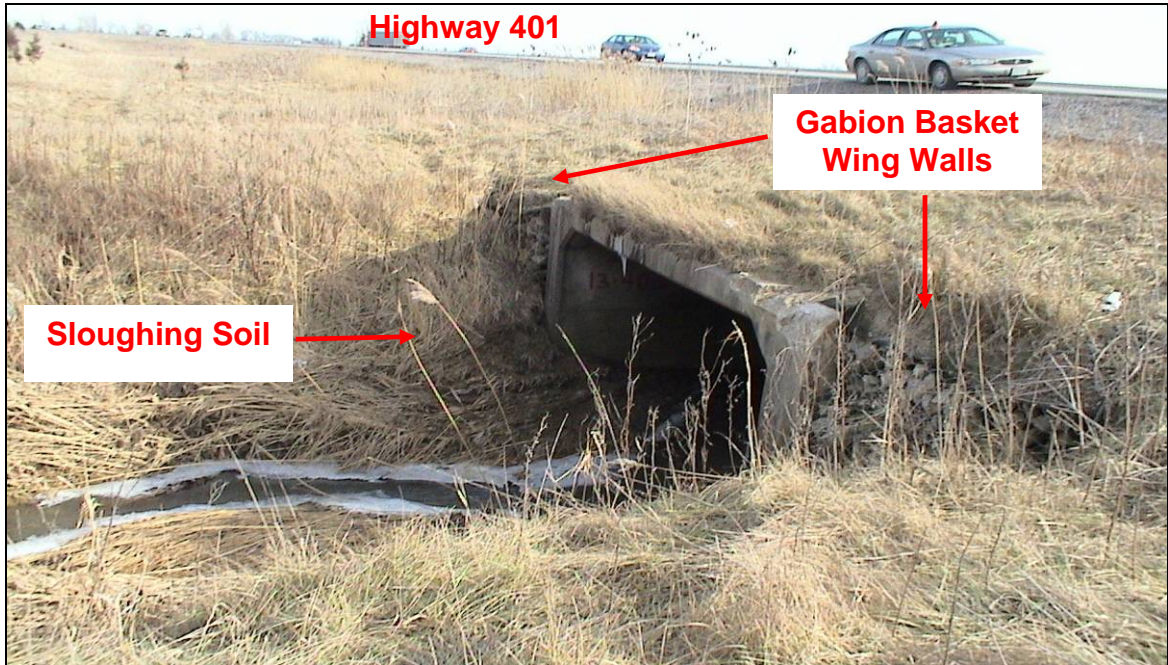
PHOTOGRAPH 3-31: Tedford Drain Culvert. Looking southeasterly at north end of Tedford Drain Culvert. Note grassed roadside ditch, gabion basket wing walls, sloughing of soil into channel. (January 27, 2006)
