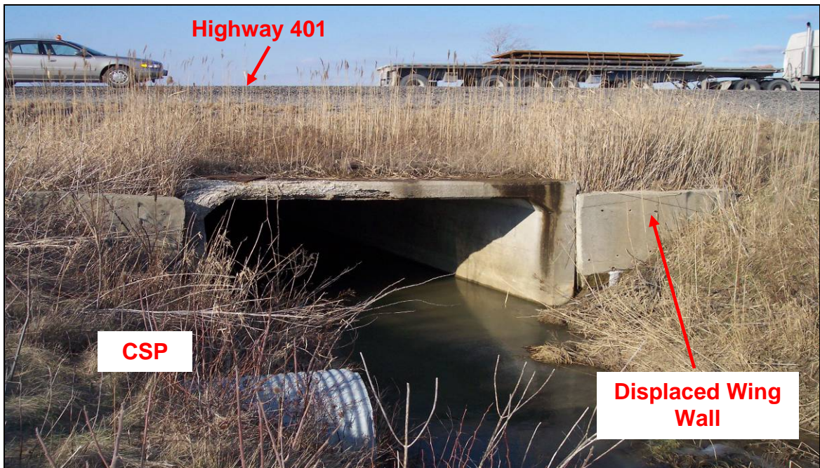
PHOTOGRAPH 3-32: Tedford Drain Culvert. Looking northerly at south end of Tedford Drain Culvert. Note displaced concrete wing walls, open channel, CSP for control of drain/roadside ditch flow. (January 26, 2006)
