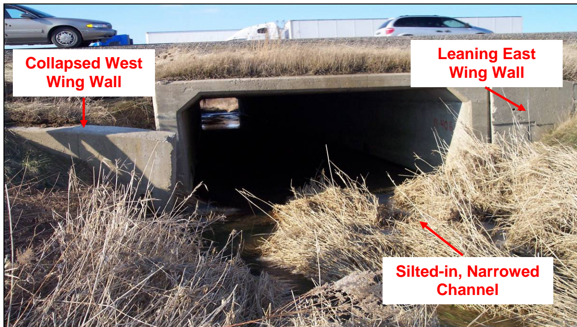
PHOTOGRAPH 3-42: Culvert Site 13-406. Looking north through south end of 13-406 culvert. Note leaning east concrete wing wall and collapsed west wing wall. Note silted-in narrowed channel with grass growth. (January 26, 2006)
