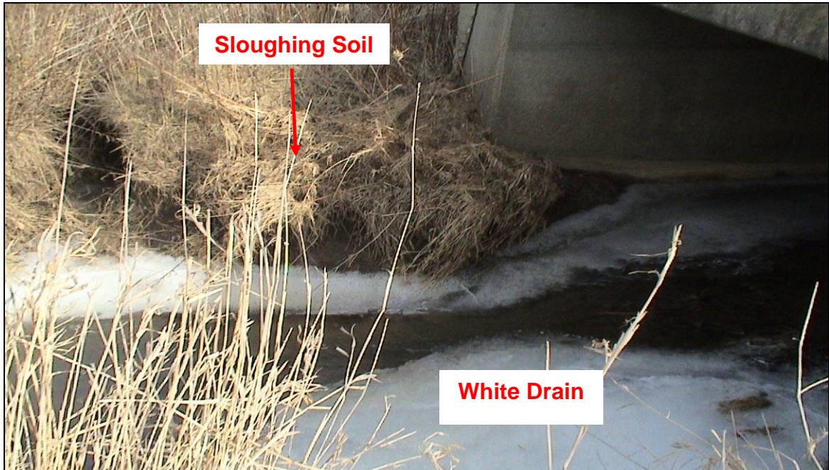
PHOTOGRAPH 3-23: White Drain Culvert. Looking east from west bank of White Drain channel to the north of Highway 401. Note narrowing of channel due to sloughing of soil into channel. (January 27, 2006)
