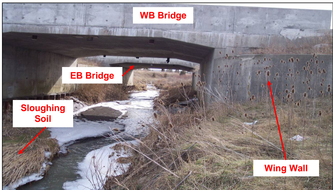
PHOTOGRAPH 3-16: McGregor Creek Bridges. Looking south along WB and EB Bridges over the McGregor Creek, from north roadside ditch. Note sloughing soil in creek in foreground left, potential erosion of channel under bridges. (January 27, 2006)
