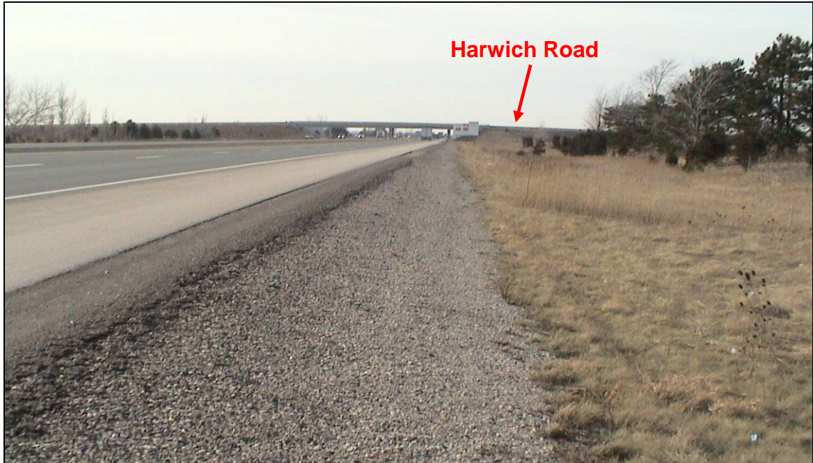
PHOTOGRAPH 3-25: Harwich Road Underpass. Looking west from north of shoulder of Highway 401 WBL, about 300 m east of structure. Note generally flat terrain and built-up approach embankments to the underpass structure. (January 27, 2006)
