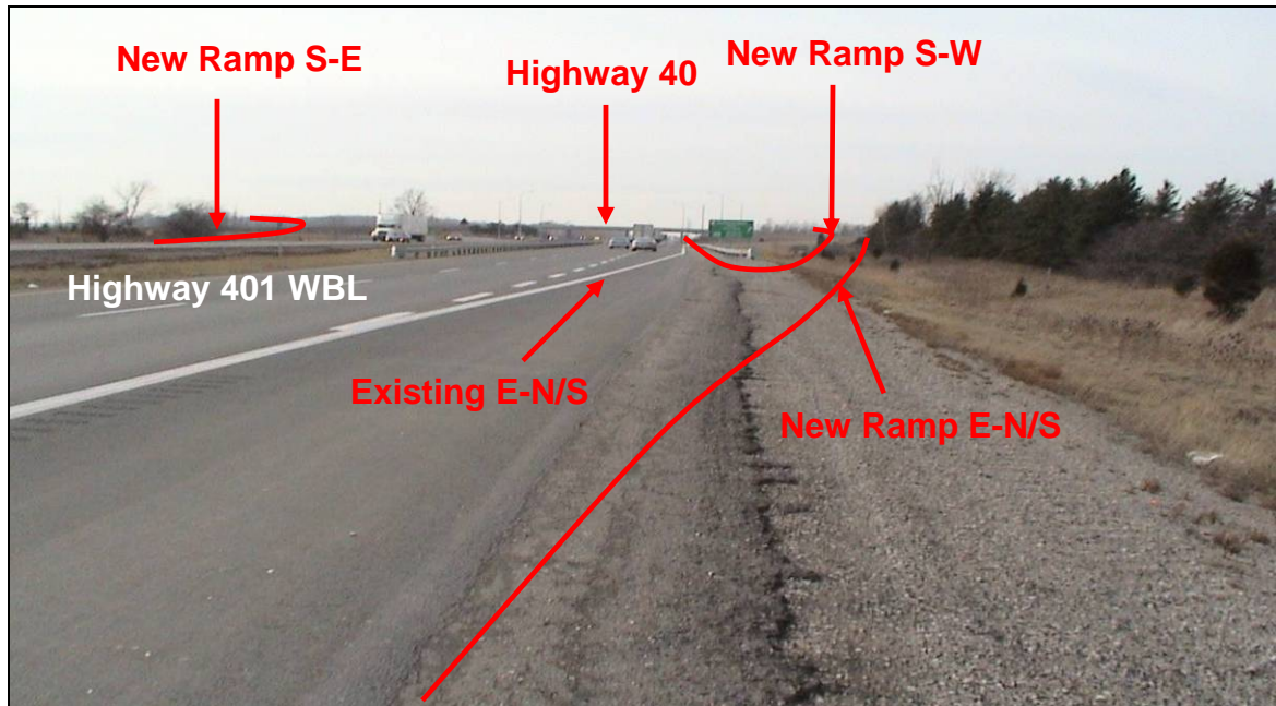
PHOTOGRAPH 3-5: Highway 40 I/C. Looking west at typically flat terrain at Highway 40 underpass from north shoulder of Highway 401. Start of E-N/S ramp in foreground. Note flat terrain beyond highway embankment. Preferred Option: Future S-E, S-W and E-N/S ramps are illustrated. (January 27, 2006)
