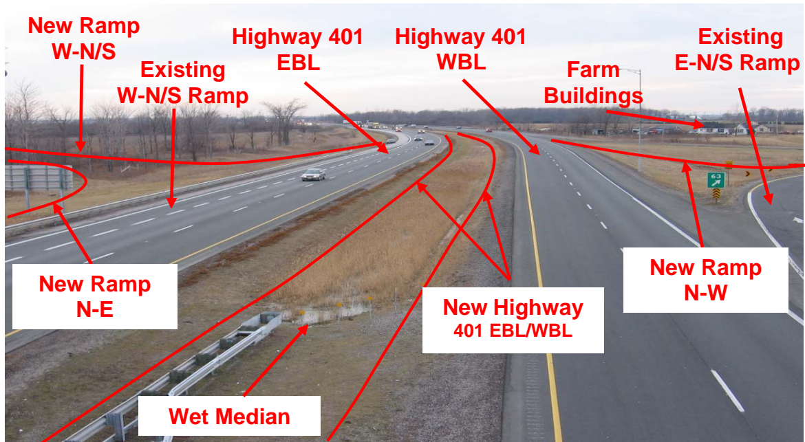
PHOTOGRAPH 1-27: Queen's Line Interchange. Looking northwesterly from top of deck of underpass structure. Note flat terrain with farm buildings, locally wet median and low embankments of Highway 401 and interchange ramps. Preferred option: Future Highway 401 EBL and WBL and W-N/S, N-E and N-W ramps are depicted in the photograph. (January 27, 2006)
