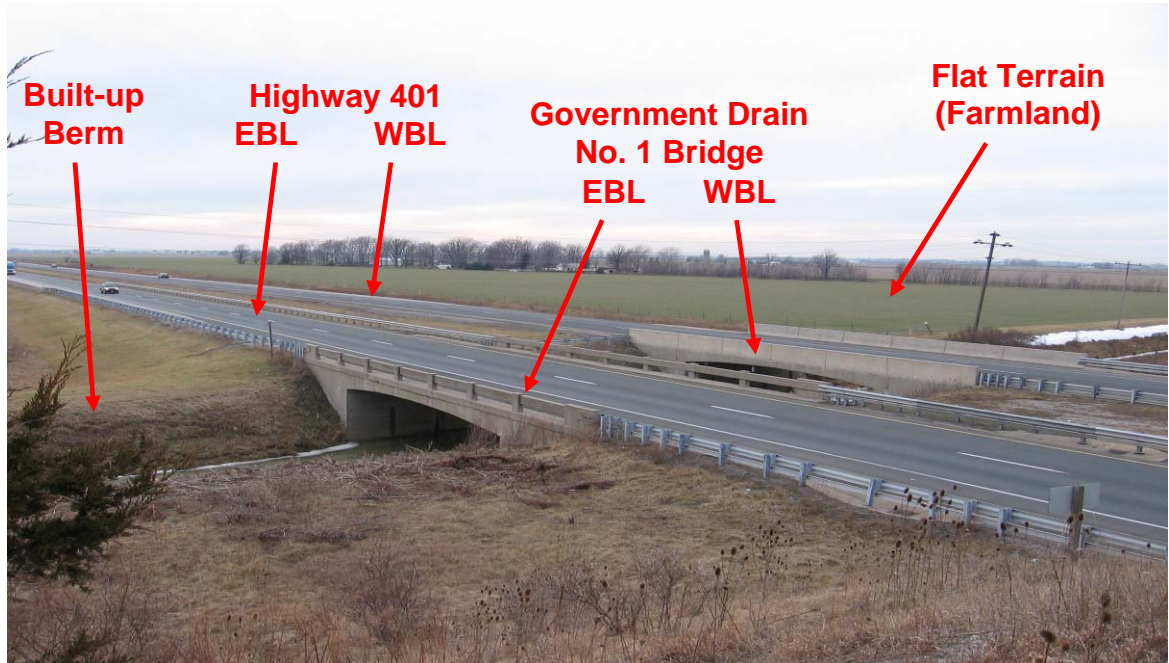
PHOTOGRAPH 1-35: Government Drain No. 1 Bridges. Looking northwesterly from south embankment of Merlin Road Underpass structure. Note flat terrain of the St. Clair Clay Plain, built-up berm south of EBL Bridge for water flow control in roadside ditch. (January 27, 2006)
