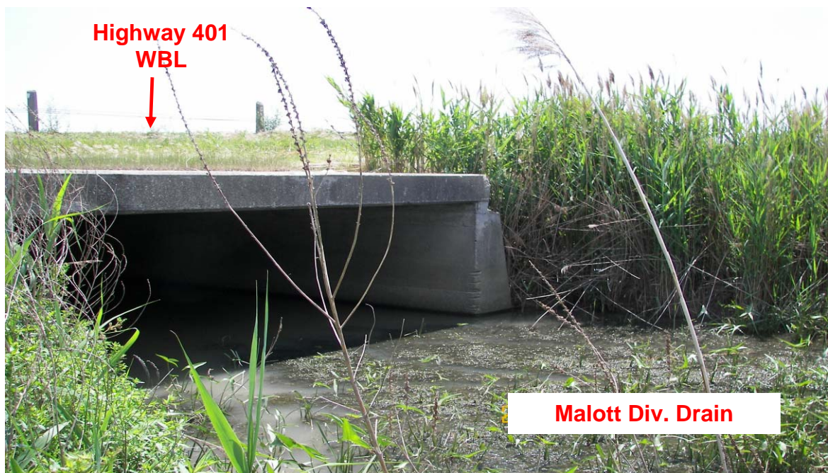
PHOTOGRAPH 1-12: Malott Division Drain Culvert. Looking southwesterly at north end of culvert from east bank of channel. Note well-vegetated banks of drain channel, low embankment of Highway 401 over top of culvert, vegetation growth in drain channel. (June 28, 2006)
