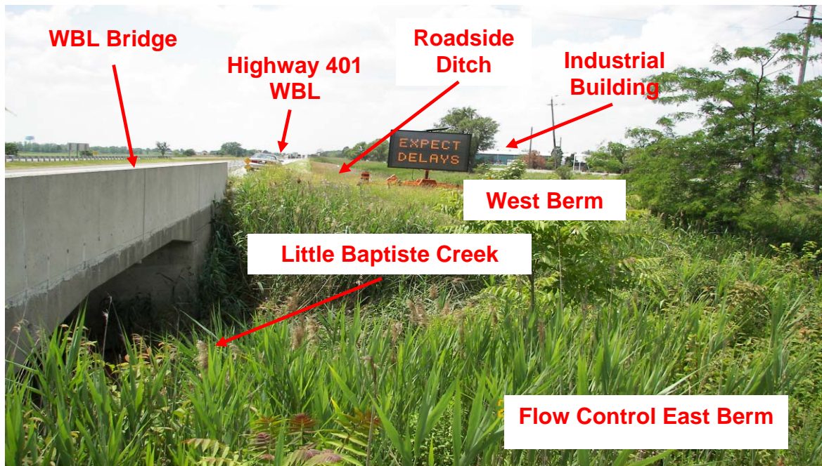
PHOTOGRAPH 1-13: Little Baptiste Creek Bridges. Looking westerly from top of east bank of Little Baptiste Creek along north of WBL Bridge. Note well-vegetated roadside ditches, industrial land use in background, warning sign atop flow control west berm, and flow control east berm in foreground. (June 28, 2006)
