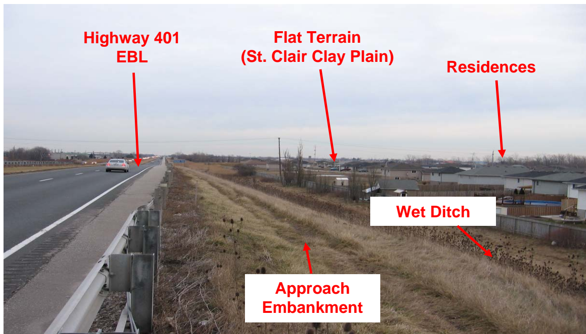
PHOTOGRAPH 1-6: Queen Street Overpass. Looking easterly from south shoulder of Highway 401 east of EBL structure. Note flat terrain in background, well-grassed built-up approach embankment and residential area of the Town of Tilbury. (January 27, 2006)
