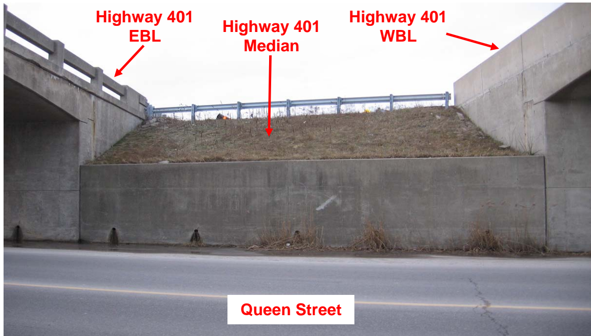
PHOTOGRAPH 1-9: Queen Street Overpass. Looking west at retaining wall between west abutments of overpass structures, grassed median of Highway 401 and crash barrier atop the slope. Note good condition of wall showing no significant lateral movement, water seeping through weep holes at base. (January 27, 2006)
