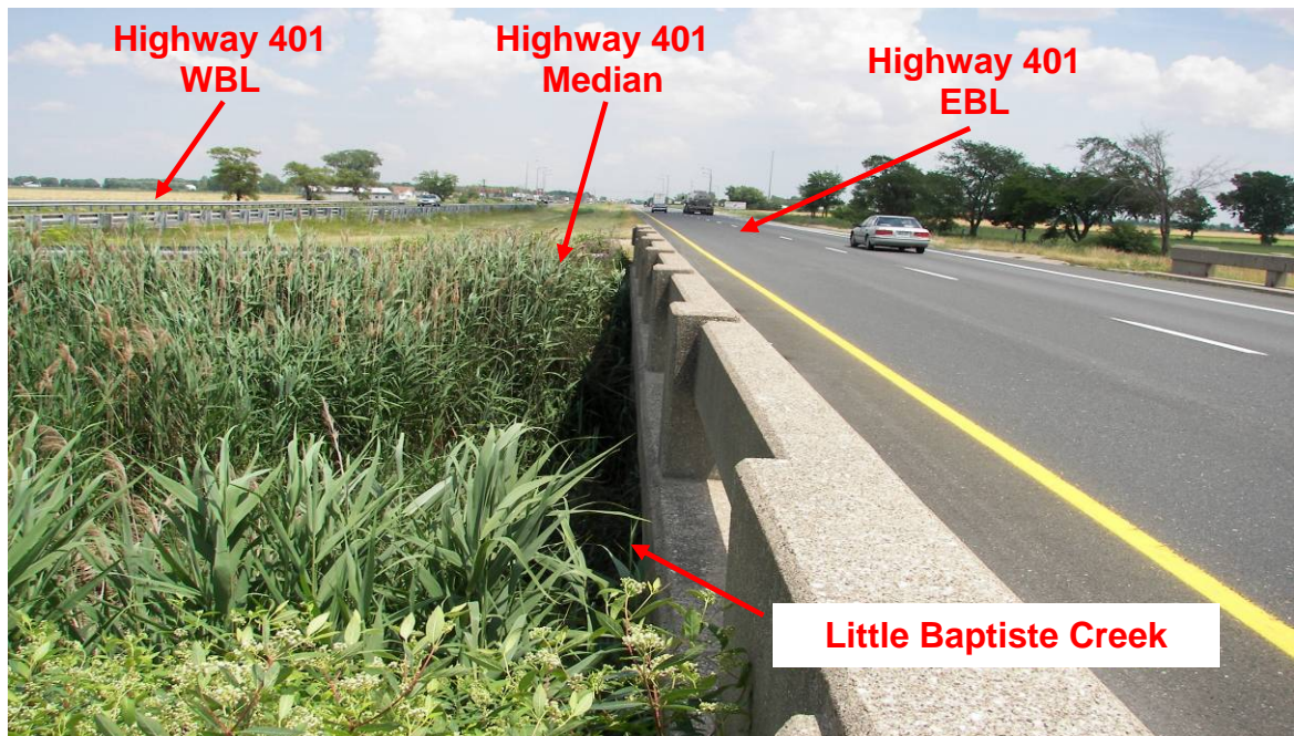
PHOTOGRAPH 1-16: Little Baptiste Creek Bridge. Looking east from west of creek at median of Highway 401 and along north side of EBL bridge. Note well-vegetated condition of median, generally flat terrain, low embankment of Highway 401. (June 28, 2006)
