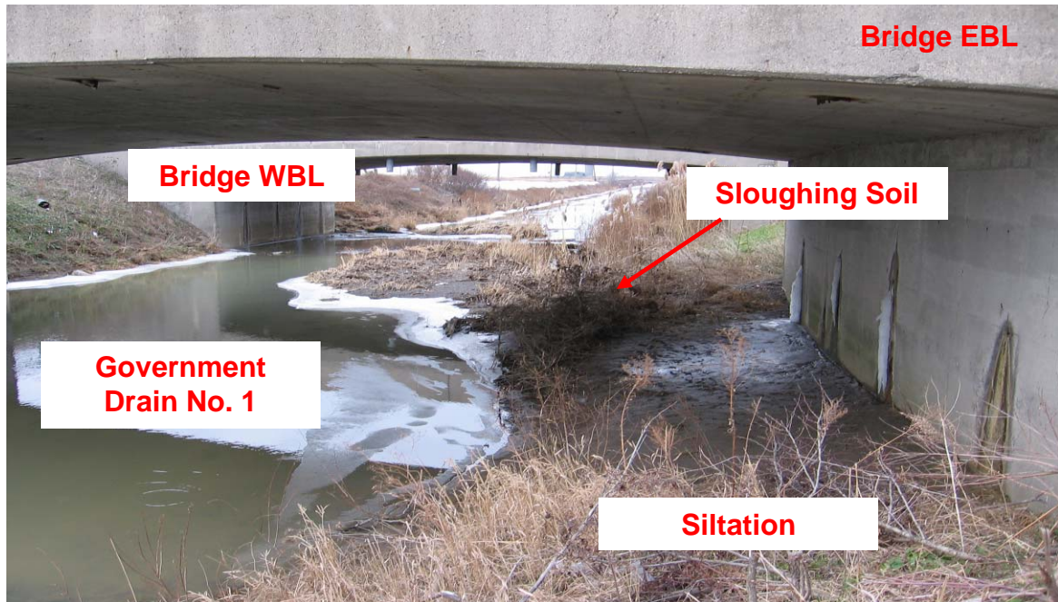
PHOTOGRAPH 1-37: Government Drain No. 1 Bridges. Looking north from the southeast bank of the EBL Bridge. Note narrowing of drainage channel due to sloughing of soil from Highway 401 median and siltation against the east abutments. (January 27, 2006)
