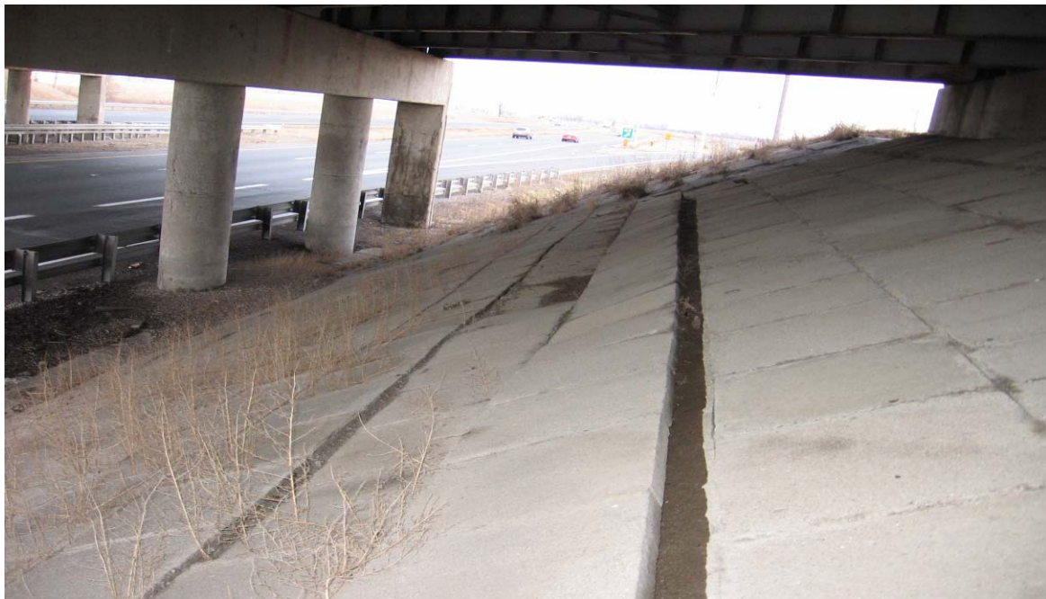
PHOTOGRAPH 1-22: Queen's Line Interchange. Looking southeasterly at foreslope of west approach embankment. Note separation in panels of concrete revetment. (January 27, 2006)
