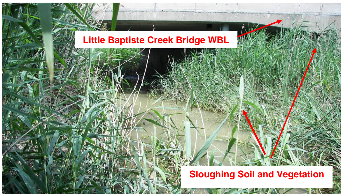
PHOTOGRAPH 1-14: Little Baptiste Creek Bridge. Looking northerly from west side of Little Baptiste Creek bank at Highway 401 median. View under WBL bridge. Note well-vegetated bank and soil sloughing into Creek channel. Note creek carrying high silt content indicating soil erosion. (June 28, 2006)
