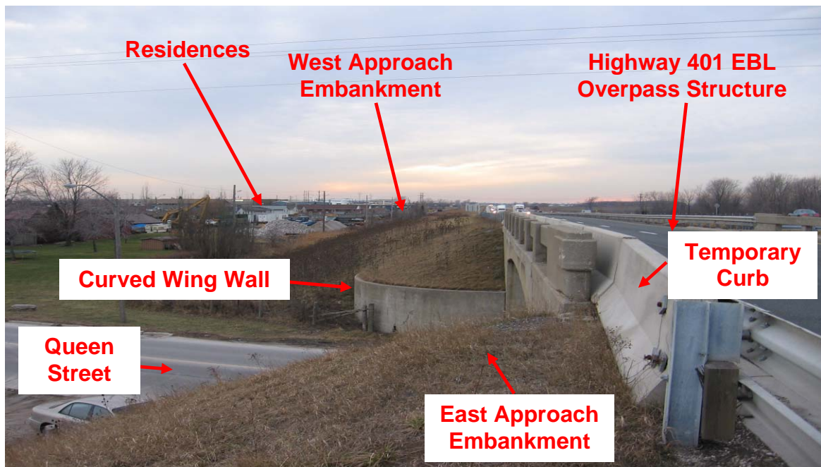
PHOTOGRAPH 1-8: Queen Street Overpass. Looking west from south shoulder of Highway 401 east of EBL structure. Note flat terrain, built-up approach embankments, temporary curbs on bridge deck of EBL structure, curved wing retaining wall at toe of slope. Residential area in background. (January 27, 2006)
