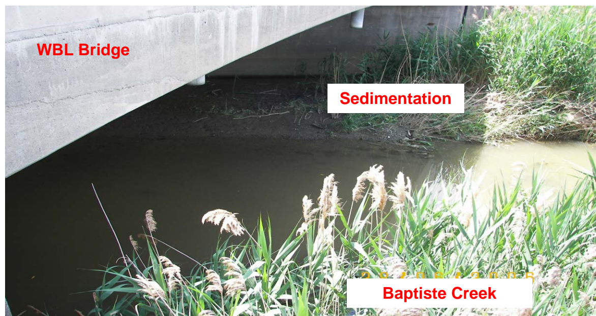
PHOTOGRAPH 1-18: Baptiste Creek Bridge. Looking northeasterly from top of Highway 401 median at east abutment of WBL bridge. Note local sedimentation with vegetation growth in front of abutment. (June 28, 2006)
