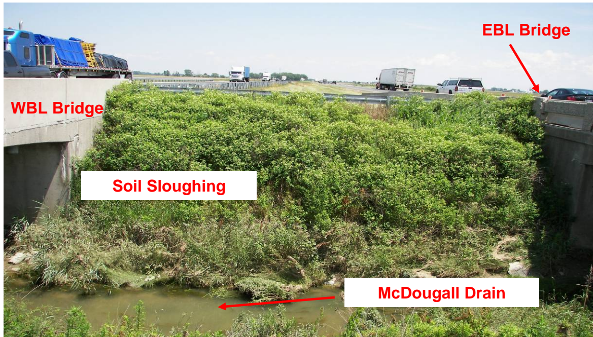
PHOTOGRAPH 1-33: McDougall Drain Bridges. Looking east from Highway 401 median west of McDougall Drain channel. Note flat terrain, shallow median ditch and well vegetated side slope of median at channel, soil sloughing at toe of median slope into channel. (June 28, 2006)
