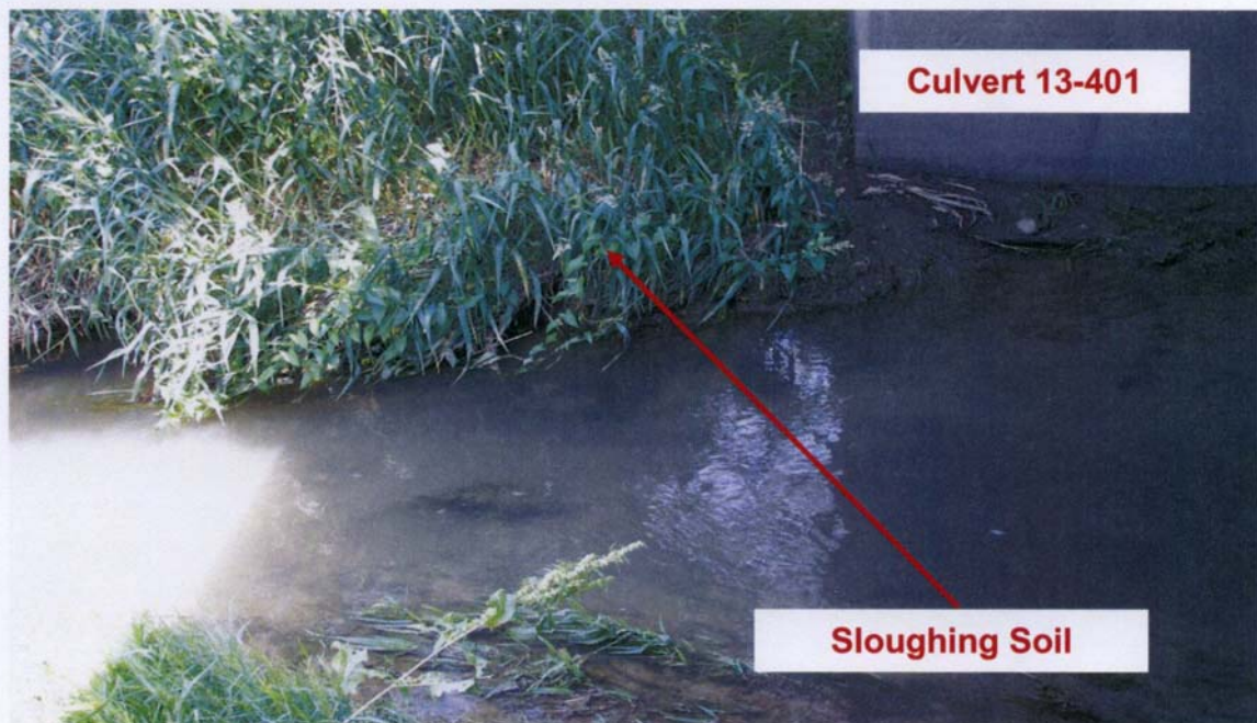
PHOTOGRAPH 2-44: Culvert Site 13-401. Looking easterly from west bank of drainage channel at north end of culvert. Close-up view of sloughing of soil at end of culvert. Note suspended silt in water indicating erosion. (June 28, 2006)
