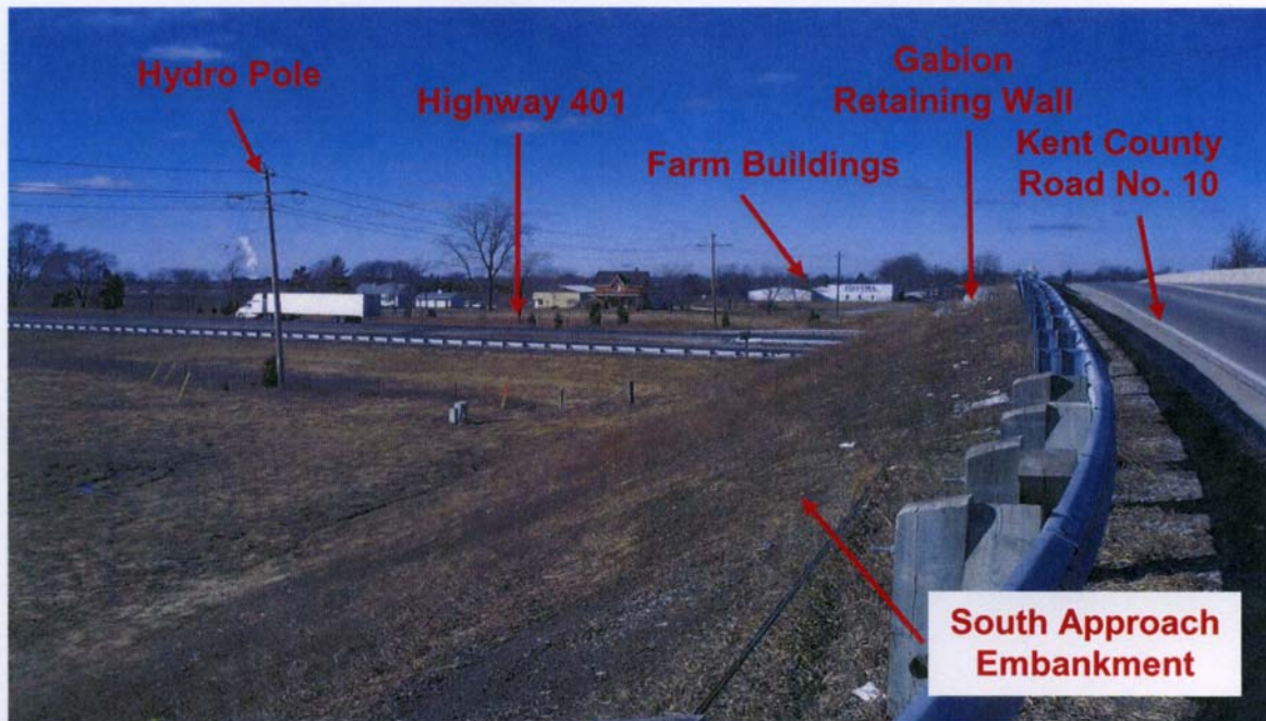
PHOTOGRAPH 2-47: Kent County Road No. 10 Underpass. Looking north from middle of south approach embankment. Note flat terrain, built-up south approach embankment in good condition, gabion basket retaining wall at structure and farming land use.
