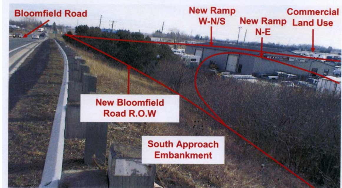
PHOTOGRAPH 2-40: Bloomfield Road Interchange. Looking south westerly from top of south approach embankment. Note well vegetated embankment slope and commercial land use near toe of slope. Preferred Option: Future Bloomfield Road R.O.W, W-N/S and N-E ramps are depicted. (January 27, 2006)
