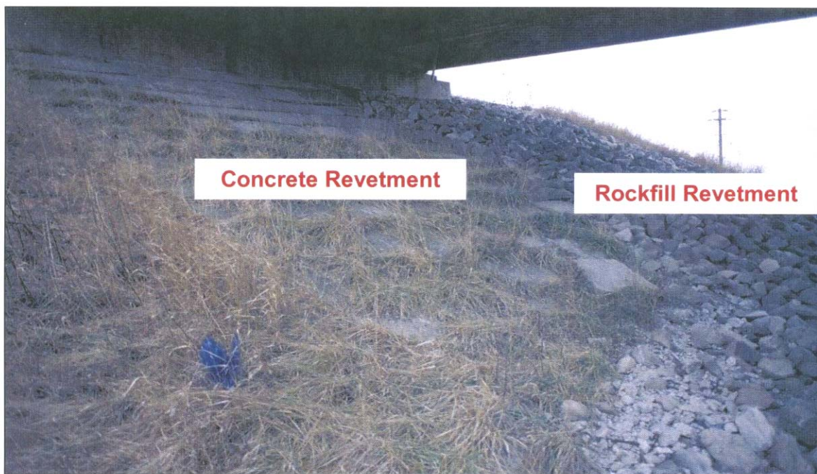
PHOTOGRAPH 2-4: Merlin Road Underpass. Looking west at revetment of south foreslope of structure. Note old concrete revetment partially replaced with crushed rockfill. (January 27, 2006)
