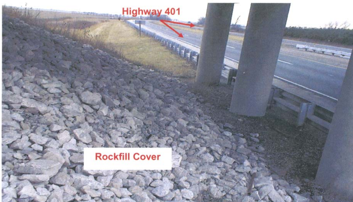
PHOTOGRAPH 2-10: Drake Road Underpass. Looking west across foreslope of south pier. Note flat terrain in distance and rockfill covering embankment foreslope. (January 27, 2006)
