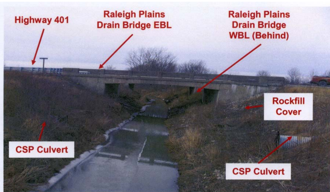
PHOTOGRAPH 2-27: Raleigh Plains Drain Bridges. Looking north at Raleigh Plains Drain Bridge EBL with Bridge WBL behind. Photograph taken from south service road. Note grassed side slopes of drainage channel, CSP culvert with one-way valve covers, rockfill over east bank. (January 27, 2006)
