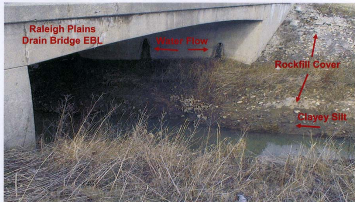
PHOTOGRAPH 2-28: Raleigh Plains Drain Bridge EBL. Looking easterly at east bank of Raleigh Plains Drain south of Bridge for Highway 401 EBL. Note clayey silt subgrade with rockfill cover, water flow through weeping holes on east abutment. (January 27, 2006)
