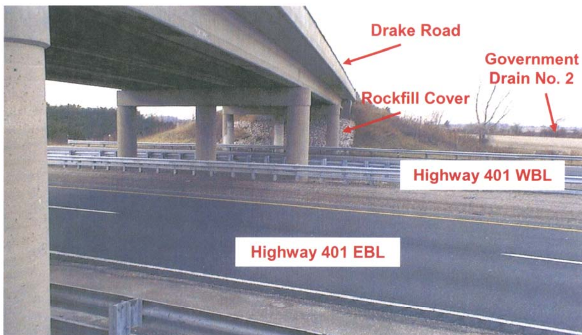
PHOTOGRAPH 2-9: Drake Road Underpass. Looking north from south shoulder of Highway 401 at south pier. Note flat terrain beyond approach embankment, Government Drain No. 2 at tree line in the background and rockfill cover on north foreslope. (January 27, 2006)
