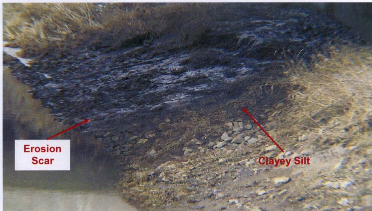
PHOTOGRAPH 2-30: Raleigh Plains Drain Bridges. Close-up of typical erosion scar under Raleigh Plains Drain Bridge EBL. Note clayey silt type subsoil. (January 27, 2006)
