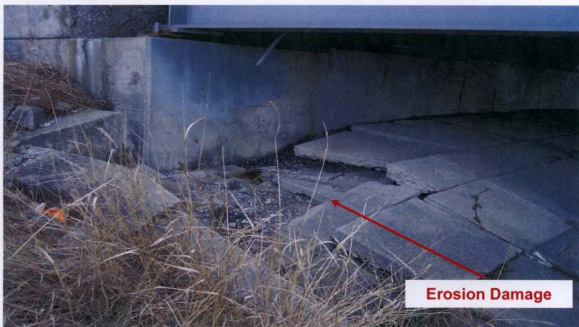
PHOTOGRAPH 2-36: Bloomfield Road Interchange. Close-up of local condition of concrete revetment of fore slope of south approach embankment. (January 27, 2006)
