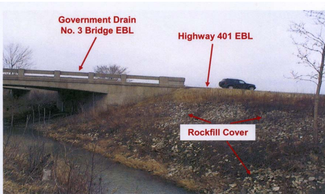
PHOTOGRAPH 2-25: Government Drain No. 3 Bridges. Looking northeasterly at east sideslope of Government Drain No. 3. Note rockfill cover south of east abutment of bridge for Highway 401 EBL. (January 27, 2006)
