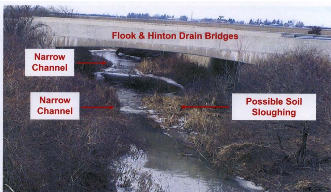
PHOTOGRAPH 2-33: Flook & Hinton Drain Bridges. Looking north at Flook & Hinton Drain Bridges EBL and WBL. (WBL Bridge located behind EBL Bridge). Note possible soil sloughing or sedimentation and narrowing of drainage channel under bridges. (January 27, 2006)
