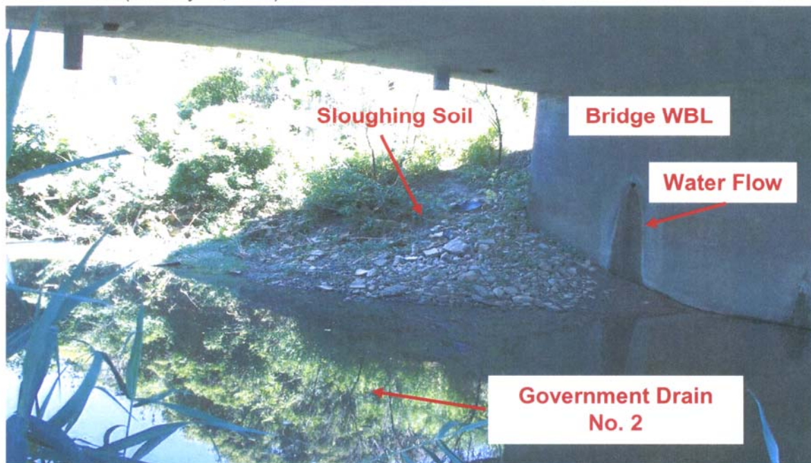
PHOTOGRAPH 2-14: Government Drain No. 2 Bridges. Looking northeasterly from base of median at west bank of channel. View under Government Drain No. 2 WBL. Note narrowed channel due to sloughing of fill soil and water flow through weephole. (June 28, 2006)
