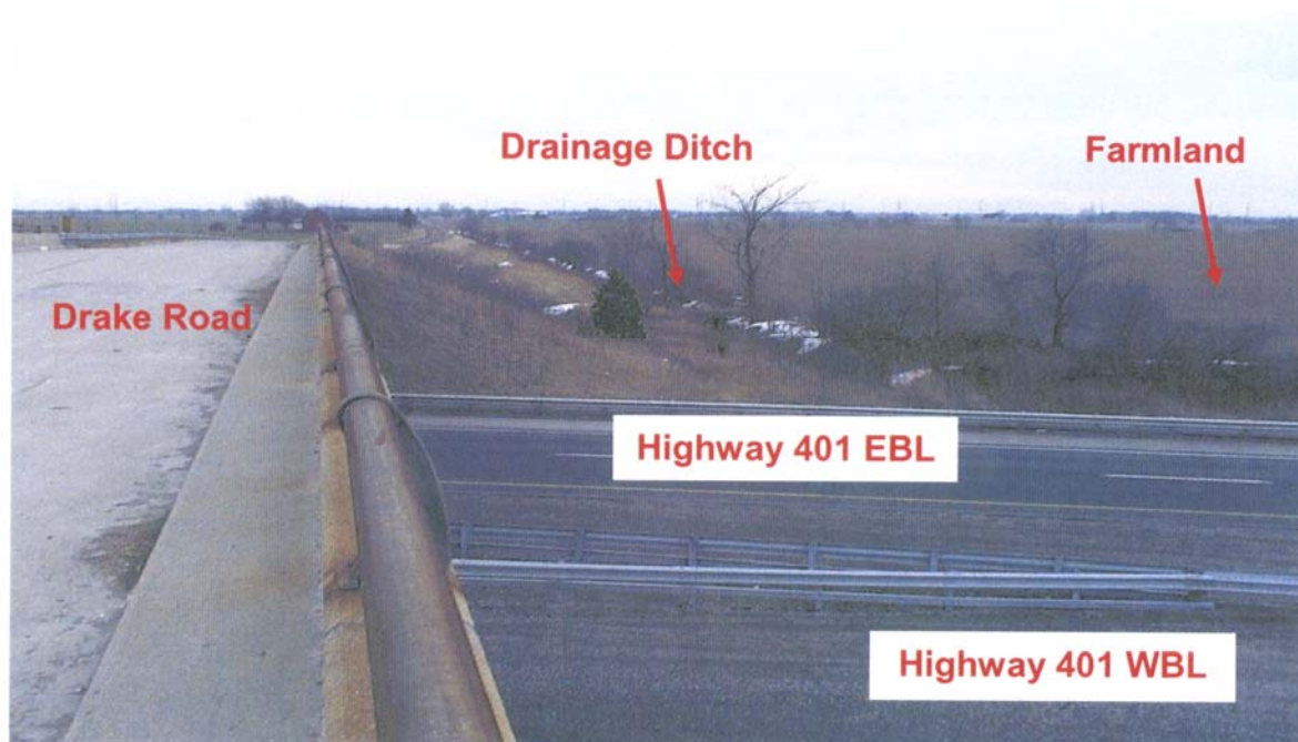
PHOTOGRAPH 2-11: Drake Road Underpass. Looking southwesterly from northwest corner of deck of structure. Note farmland in middle of photograph, drainage ditch along west toe of slope of south approach embankment, typically flat terrain. (January 27, 2006)
