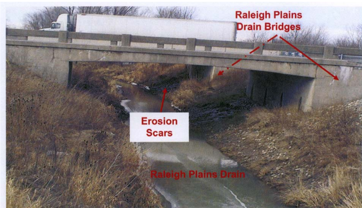
PHOTOGRAPH 2-29: Raleigh Plains Drain Bridges. Looking north easterly at Raleigh Plains Drain Bridges EBL and WBL (under white truck). Note erosion scars under each bridge accentuated by dark colour. Refer to following photograph for close-up. (January 27, 2006)
