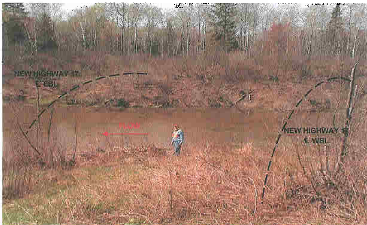
Photograph 20 VIEW: Looking west along new Highway 17 alignment of Alt. 4 and 5 (Sta. 17+020) through pond of beaver dam on Rocha's property. Side slopes of ponded water consist of clayey silt. B.R. Gray standing on centreline median. Potential culverts required through 30 to 40 m wide crossing. (May 1, 2006)
