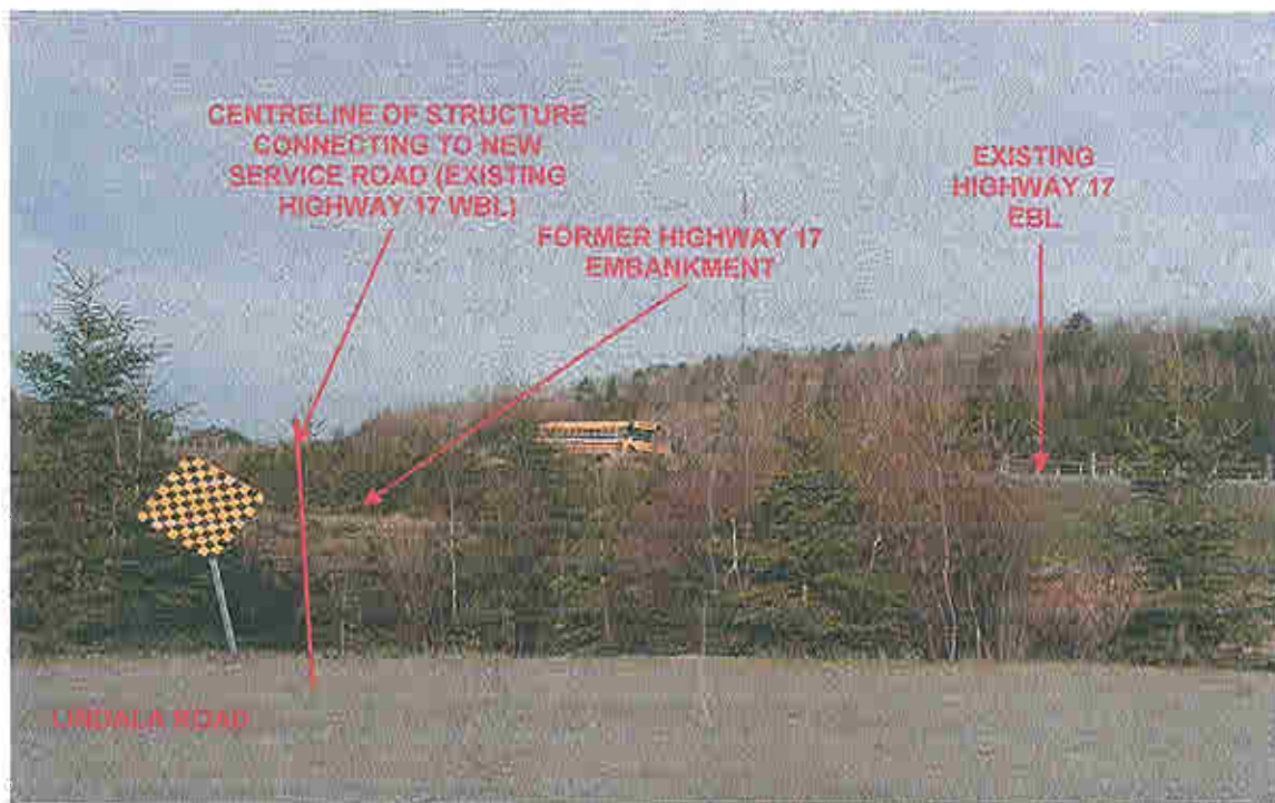
Photograph 14 VIEW: Looking west from end of Lindala Road. Bus travelling on EBL of Highway 17. New structure alternative to connect New Service Road (existing Highway 17 WBL) to Lindala Road. Applicable to Alternatives 4 to 9. Old Highway 17 constructed on swamp lands. Depth to bedrock over 19 m. Depth to firm bottom 14 to 17 m. (May 1, 2006)
