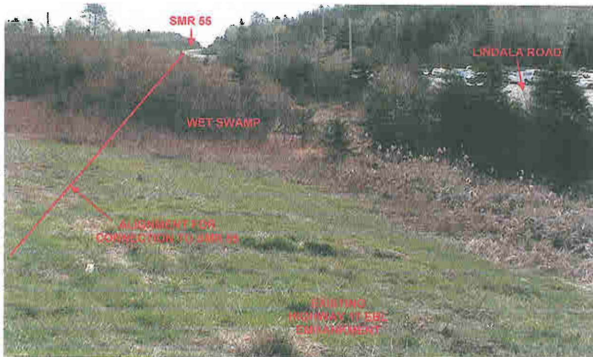
Photograph 10 VIEW: Looking southerly along alignment of alternative connection to SMR 55. Embankment on wet swamp between Highway 17 eastbound embankment in foreground and SMR 55 in background. Depth to firm bottom is about 14 to 17 m. (May 1, 2006)
