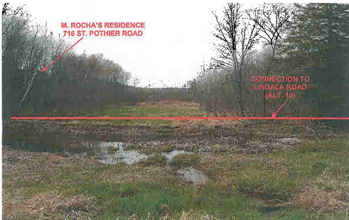
Photograph 24 VIEW: Looking south at connecting road to Lindala Road for Alt. 10 New Highway 17. Embankment through swamp will require a culvert. (May 1, 2006)
