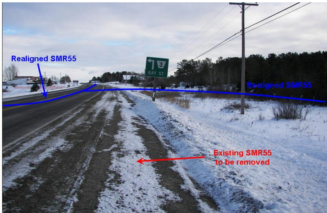
Photograph 105 VIEW: Looking east from south shoulder of SMR55 at new intersection of Realigned SMR55 and connection with existing SMR55. Note commercial and residential structures of Whitefish visible in distance. (Dec. 6, 2007)
