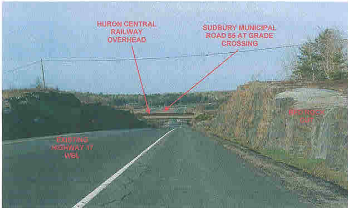
Photograph 1 VIEW: Highway 17 looking west from north shoulder of WBL about 350 m east of railway overhead. (Limit of project). Note 6 m high rock cut, low laying terrain beyond in Fairbank Creek floodplain. (May 1, 2006)
