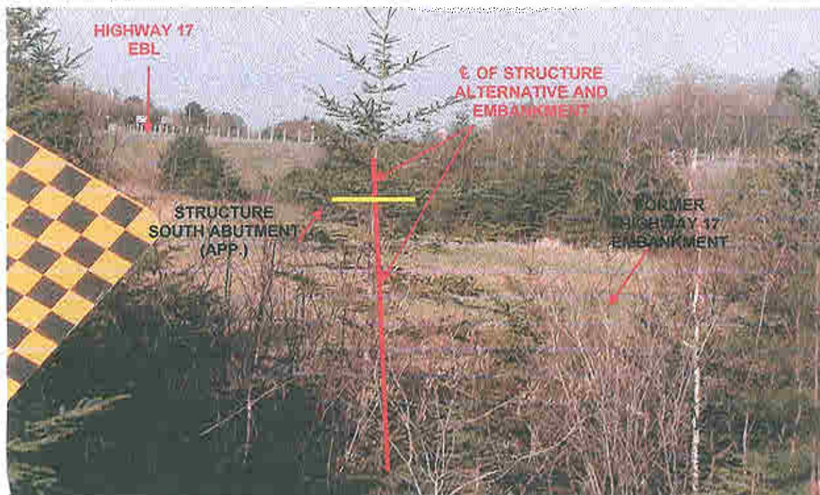
Photograph 15 VIEW: At end of Lindala Road looking westerly from west end of Lindala Road along centreline of alternative flyover structure to connect to new Service Road (existing Highway 17 WBL). Applicable to Alternatives 4 to 9. Depth to rock is over 19 m. Depth to firm bottom 14 to 17 m. Foreground is former Highway 17 embankment. (May 1, 2006)
