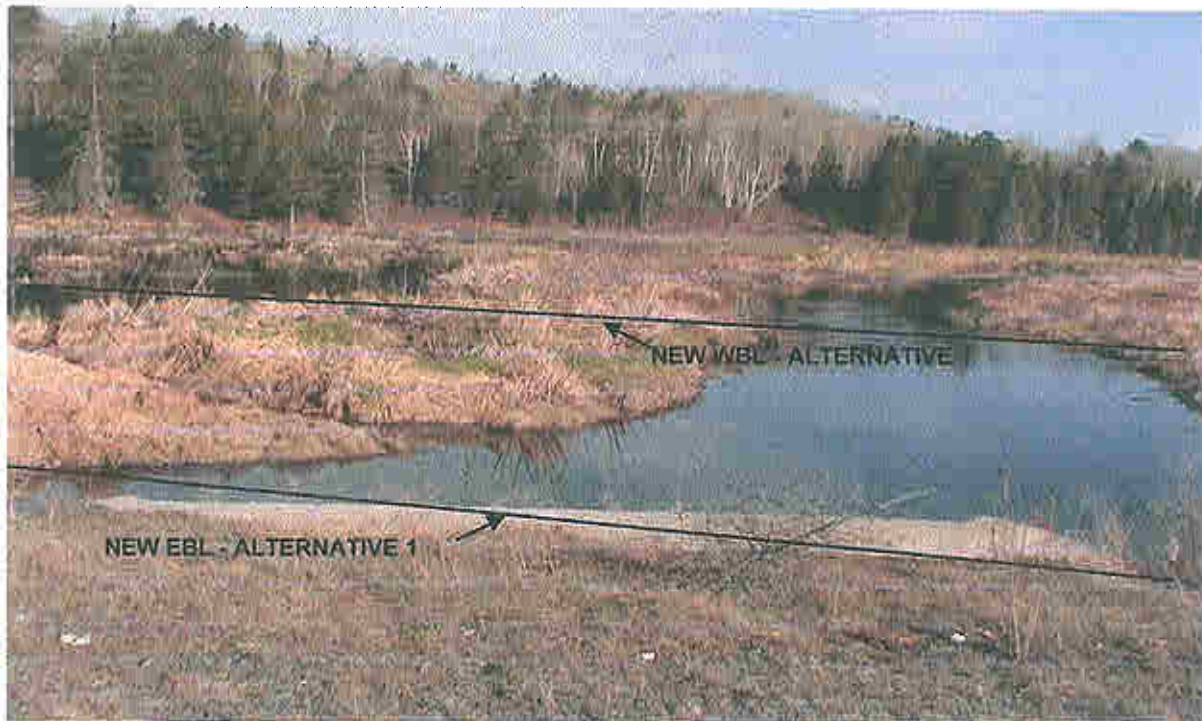
Photograph 4 VIEW: Highway 17 Sta. 17+750 (Alt. 1). Looking north across top of Fairbank Creek culvert. Note open water and swamp. Depth to firm bottom is about 15 m, Artesian conditions exist. (May 1, 2006)
