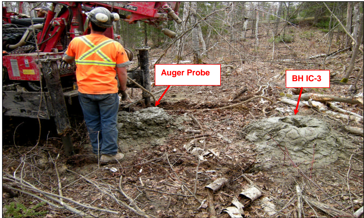
Photograph 3: Looking southerly at BH IC-3 while drilling auger probe to refusal near borehole to confirm inferred bedrock. (May 4, 2008)
