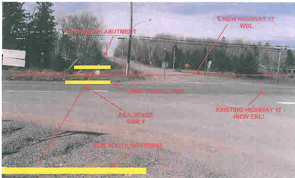
Photograph 41 VIEW: Looking north from west shoulder of Den/Lou Road about 10 m south of Highway 17. Depth to rock at new structure is about 12 to 15 m. Alternative 2 – New Highway 17 Twinning North. (May 1, 2006)
