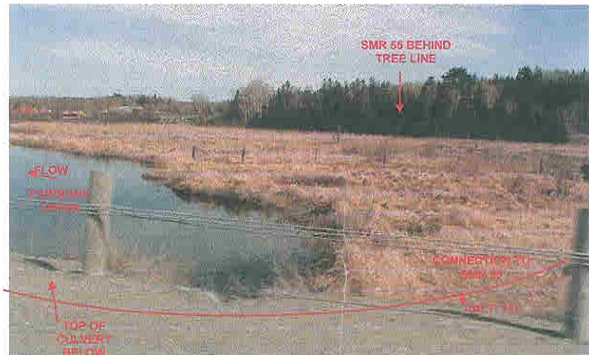
Photograph 6 VIEW: Looking south to Fairbank Creek across top of culvert from south shoulder of existing Highway 17 EBL. Depth to firm bottom in Fairbank Creek is about 19 m. (May 1, 2006)
