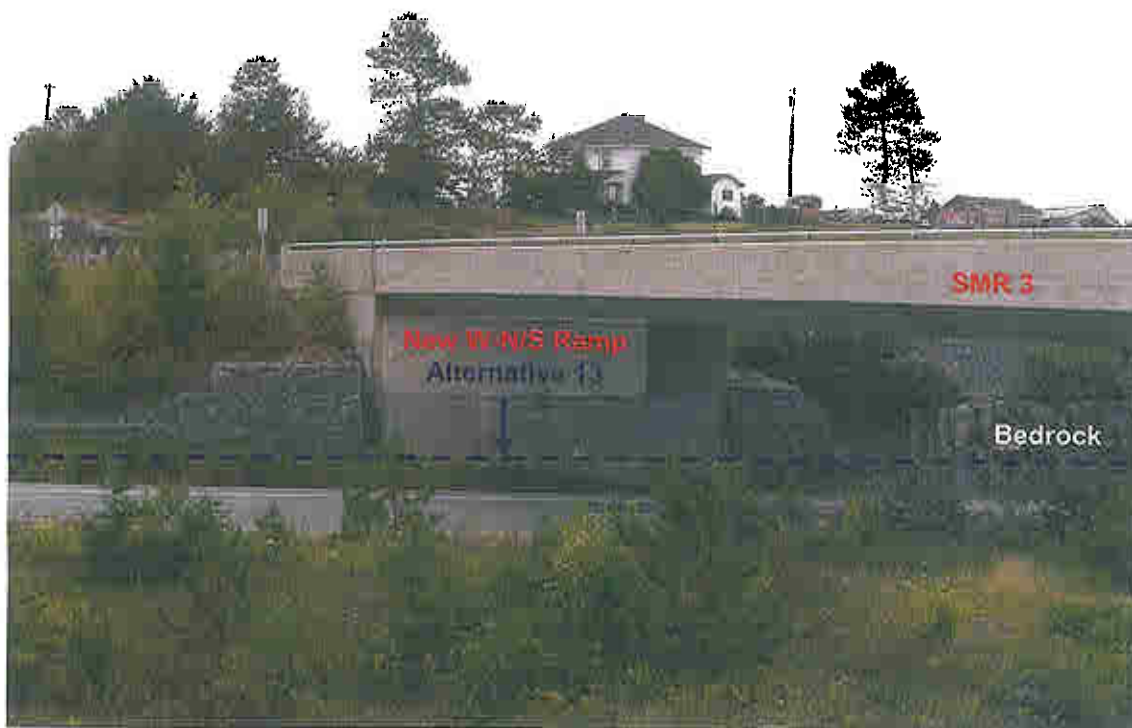
Photograph 79 VIEW: Looking south from north side of Highway 17 at about Sta. 19+060, some 20 m east of SMR 3 underpass structure at south abutment founded on bedrock. (September 12, 2006)
