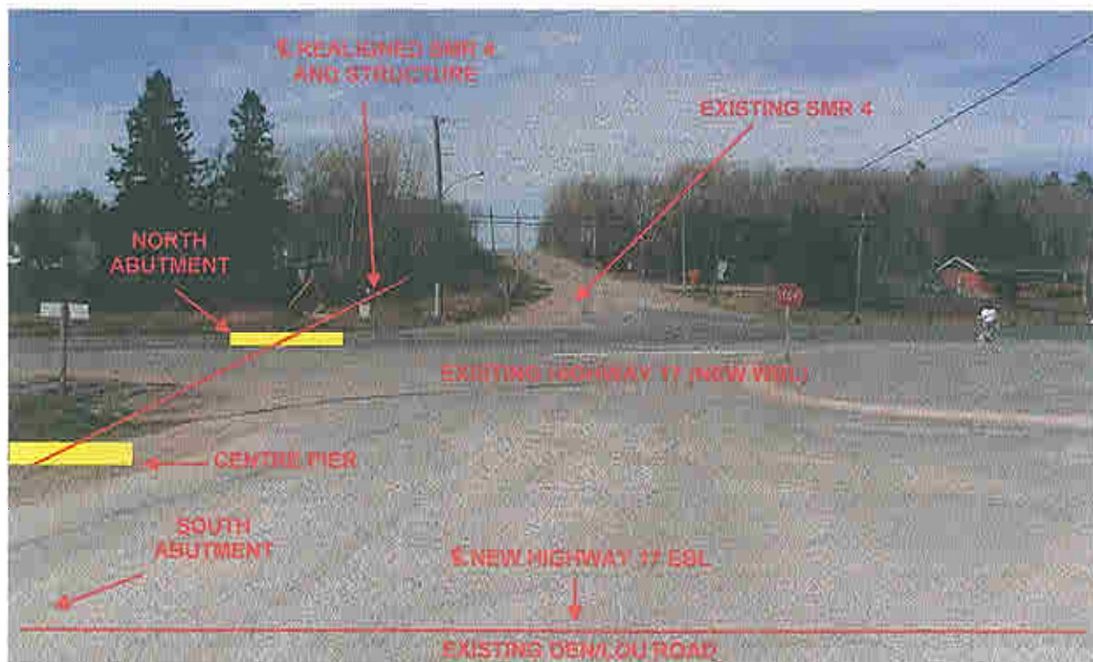
Photograph 42 VIEW: Looking north from east shoulder of Den/Lou Road about 30 m south of Highway 17. Depth to rock about 12 to 15 m. Alternative 3 – New Highway 17 Twinning South Alignment. (May 1, 2006)
