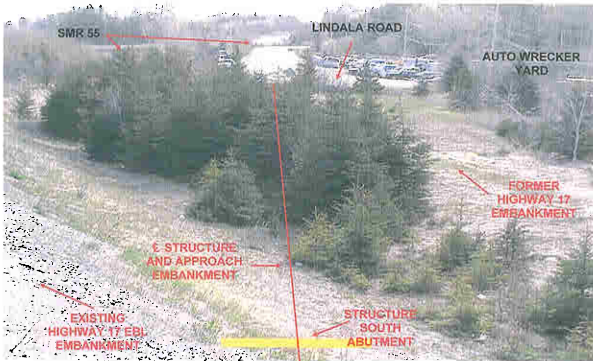
Photograph 13 VIEW: Looking southeasterly at Lindala Road from shoulder of Highway 17 EBL. Alignment of centreline for alternative connection using flyover. Former Highway 17 embankment in foreground right. Depth to bedrock over 19 m. Applicable to Alternatives 4 to 9. (May 1, 2006)
