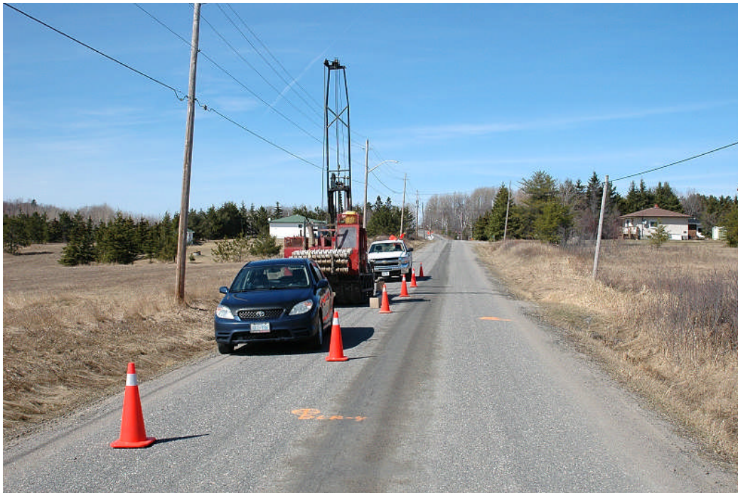
Photograph 2: Proposed Den-Lou Road Underpass site. Looking north at proposed structure location. Drill rig on north approach borehole. Note residences from former Town of Walden in background. (April 19, 2007)
