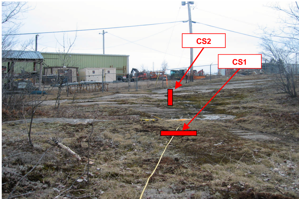
Photograph 1: Looking west from east of proposed east abutment. Location of centre pier is at fence line, proposed west abutment is located between the nearest hydro pole and Hydro One building. Note extensive bedrock outcrop. (April 17, 2007)
