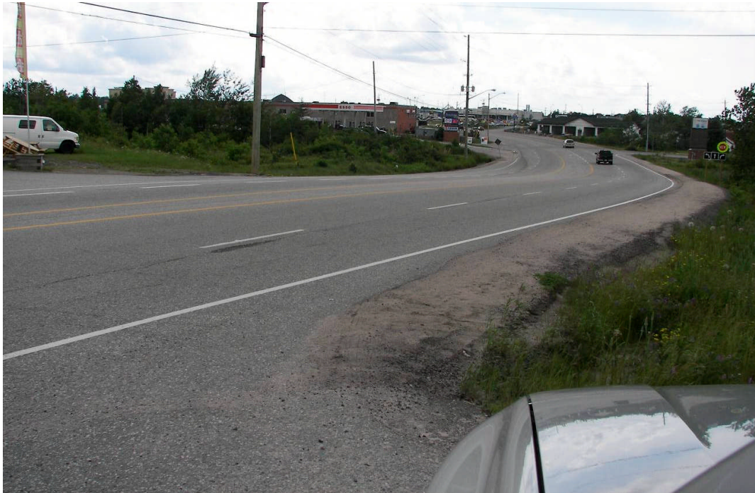
Photograph 1: Looking west along Seymour Street at location of proposed overpass. South abutment is located between the two nearest hydro poles. Note embankment through low-lying area for existing Seymour Street platform. (June 19, 2007)
