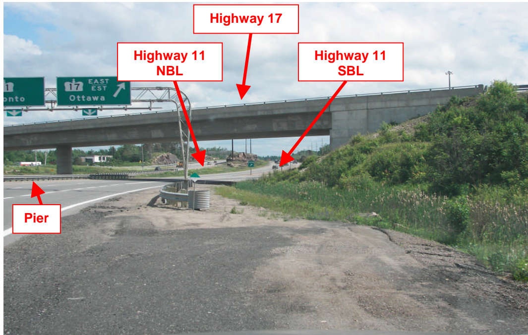
Photograph 1: Looking south at existing Highway 17 and Highway 11 interchange underpass. Note median retaining wall at west abutment. Existing grade was lowered at the underpass (note rock cut in distance on Highway 11 median). (June 19, 2007)
