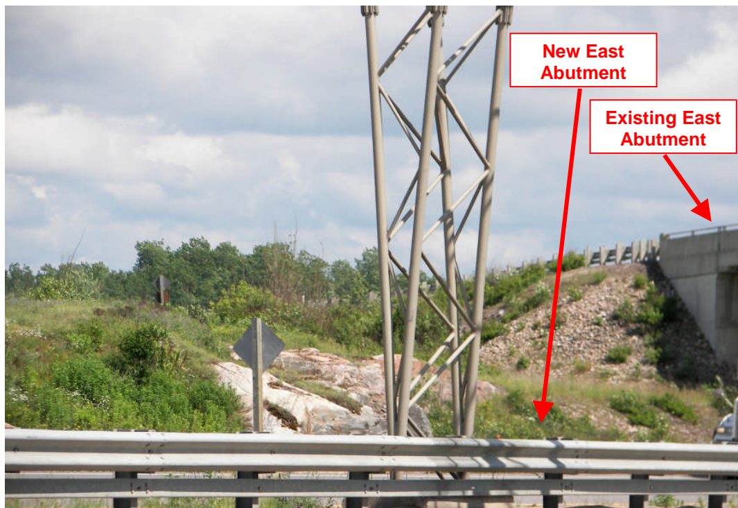
Photograph 2: Zoom view of east abutment showing extensive rock outcrop exposures. (June 19, 2007)
