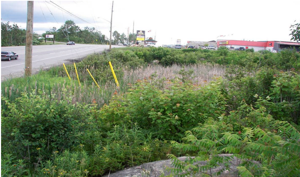
Photograph 5 (Sta. 16+560): Looking east across swamp 102 south of Seymour Street from outcrop at edge of Esso Gas Station. Parking lot beyond swamp is on bouldery fill pad. (June 19, 2007)
