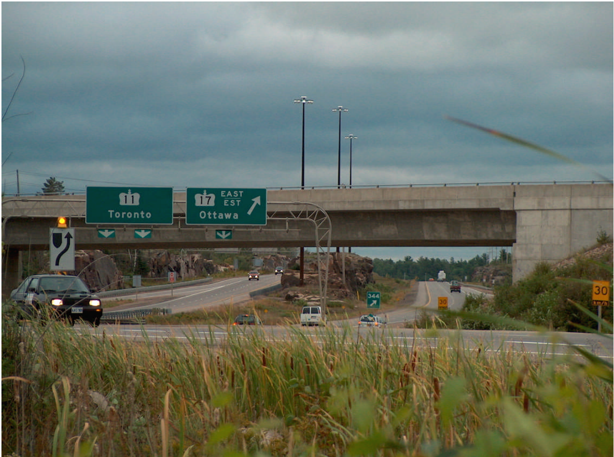
Photograph 1 (Sta. 16+920) (Zoom View): Looking southerly from east of Highway 11/17 (in foreground). Existing Highway 11 and Highway 17 interchange structure is to be widened. Rock outcrops occur at the median and east sides of Highway 11 and are visible under the bridge. View of swamp vegetation was captured at bottom of photograph. (September 14, 2005)
