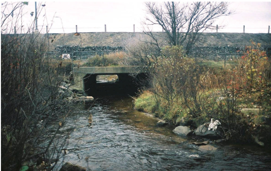
Photograph 20 (Sta. 13+930): Looking south at north end of the Chippewa Creek culvert. Note existing Highway 11/17 embankment and gabion baskets over top of culvert. (November 4, 2004)
