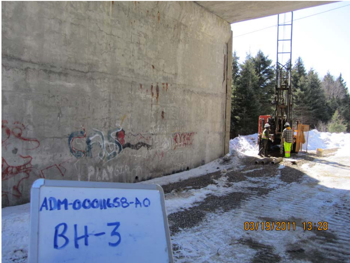
Photo No. 5: Set-up at BH-3 located on south-west side of bridge. Borehole advanced from historic railway surface. View looking south-west.
