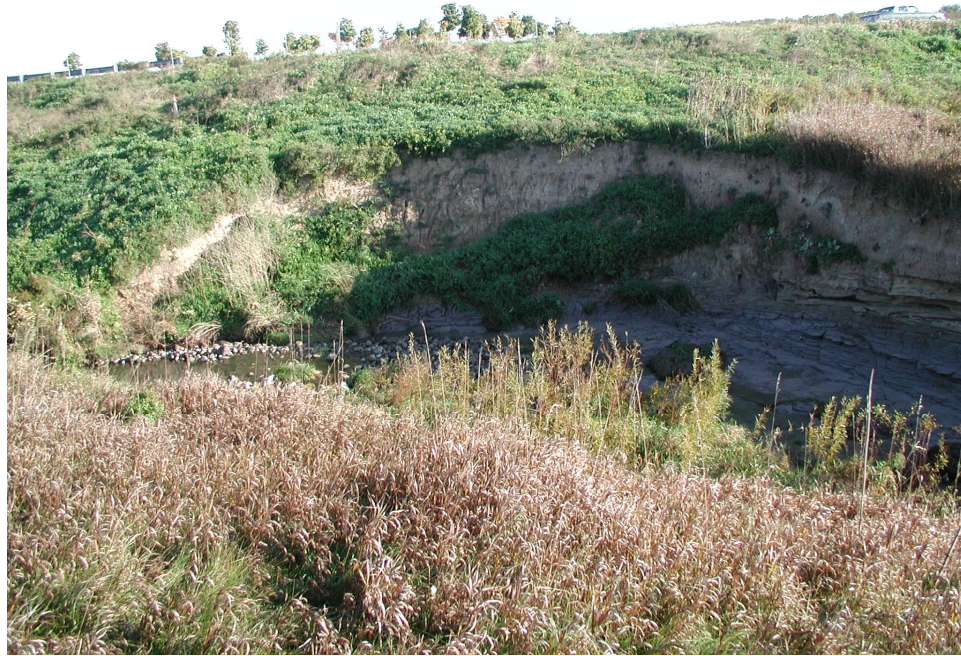
Photo 1 View of failure scarp below W-N/S ramp from west bank of creek. Cobbles washed downstream from original channel works are evident in left side of photo.
