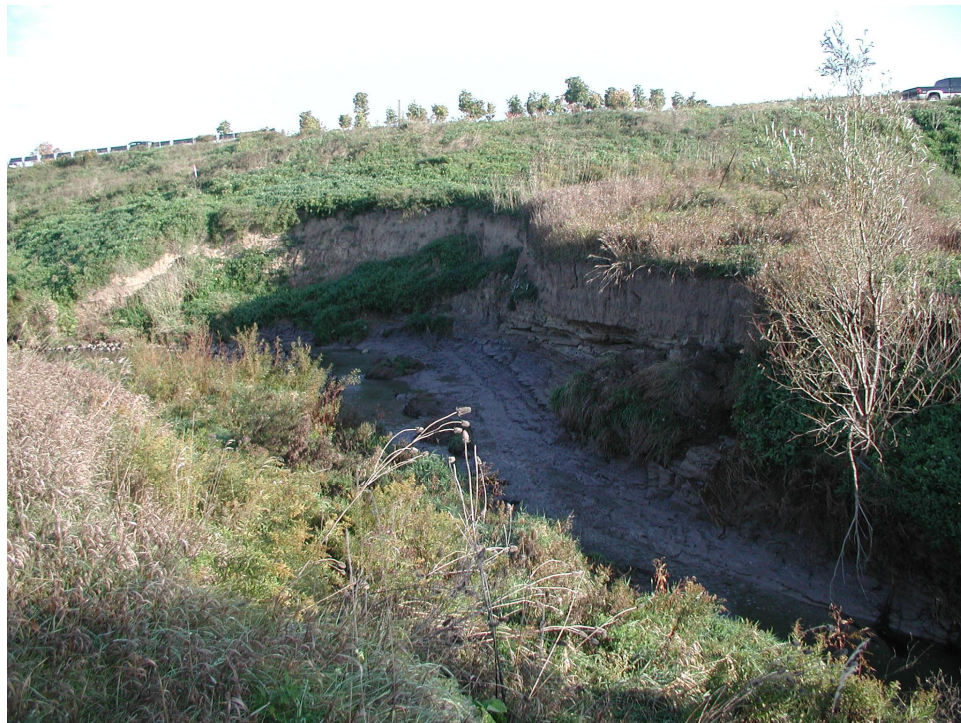
Photo 2 View of failure scarp looking upstream from west bank of creek.
