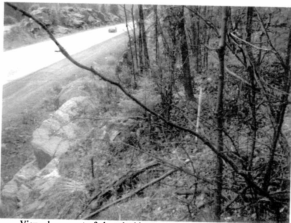
Image 2 View along crest of slope looking south. Note set back of abutment centerline from crest of rock face, and vegetation/soil cover materials to remove prior to final inspection.
