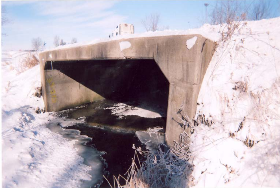
Photograph 5: View northeast of culvert outlet from south side of creek. Note crack in concrete.
