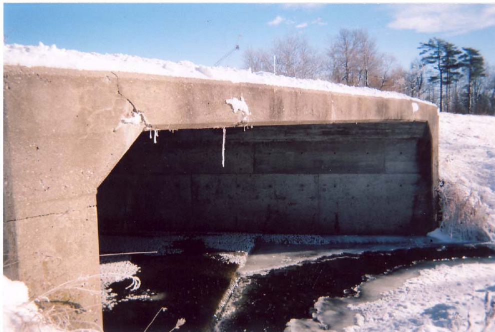
Photograph 6: View southeast of culvert outlet from north side of creek. Note crack in concrete.
