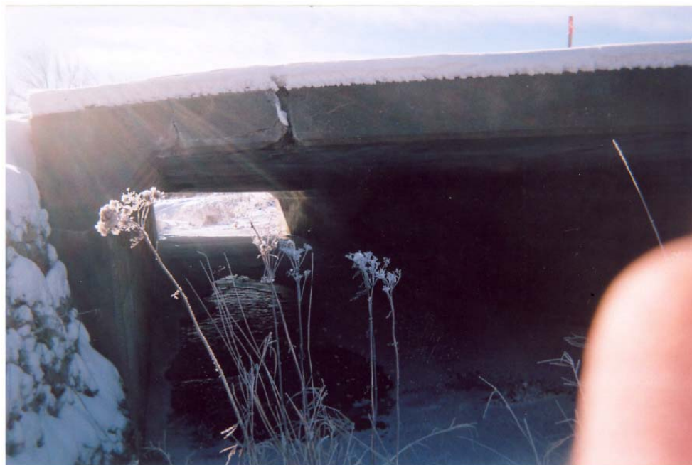
Photograph 4: View west of inlet to culvert. Note crack in concrete.
