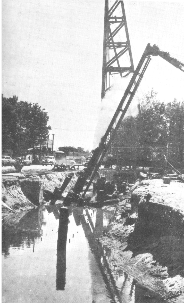
Photo 1 : Undated photograph 1 shows pile installation at an Ontario Department of Highways overpass in Sarnia. The site is believed to be Colborne Road. Vertical and battered jack pine piles were driven to found the abutments.
